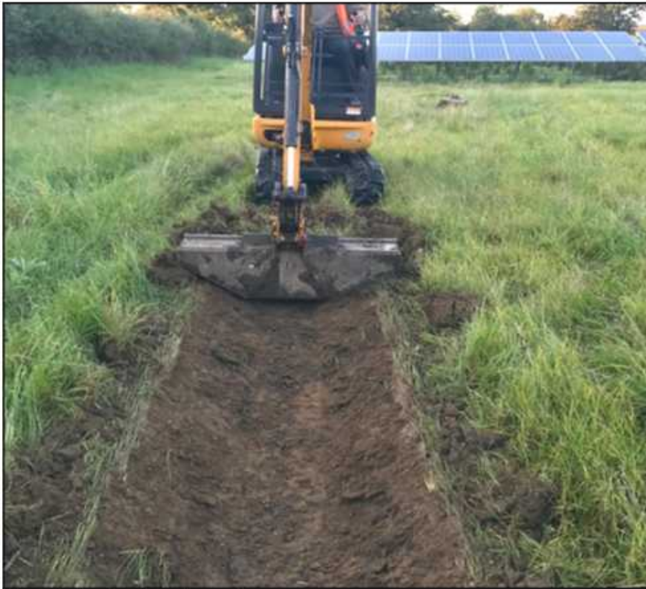
Figure 3: Construction of a swale
