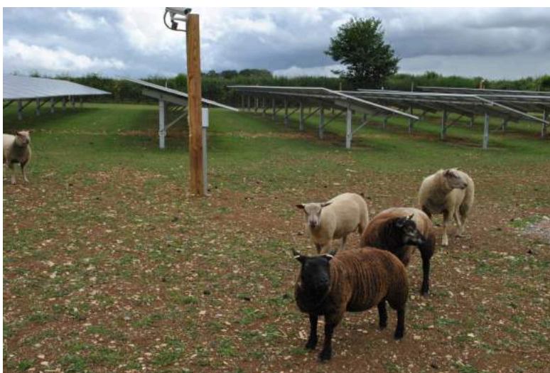
Figure 8 - solar panels mounted on galvanised metal frames set into the ground by either direct or screw piling
