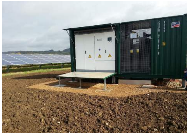
Figure 10: Typical inverter cabin
