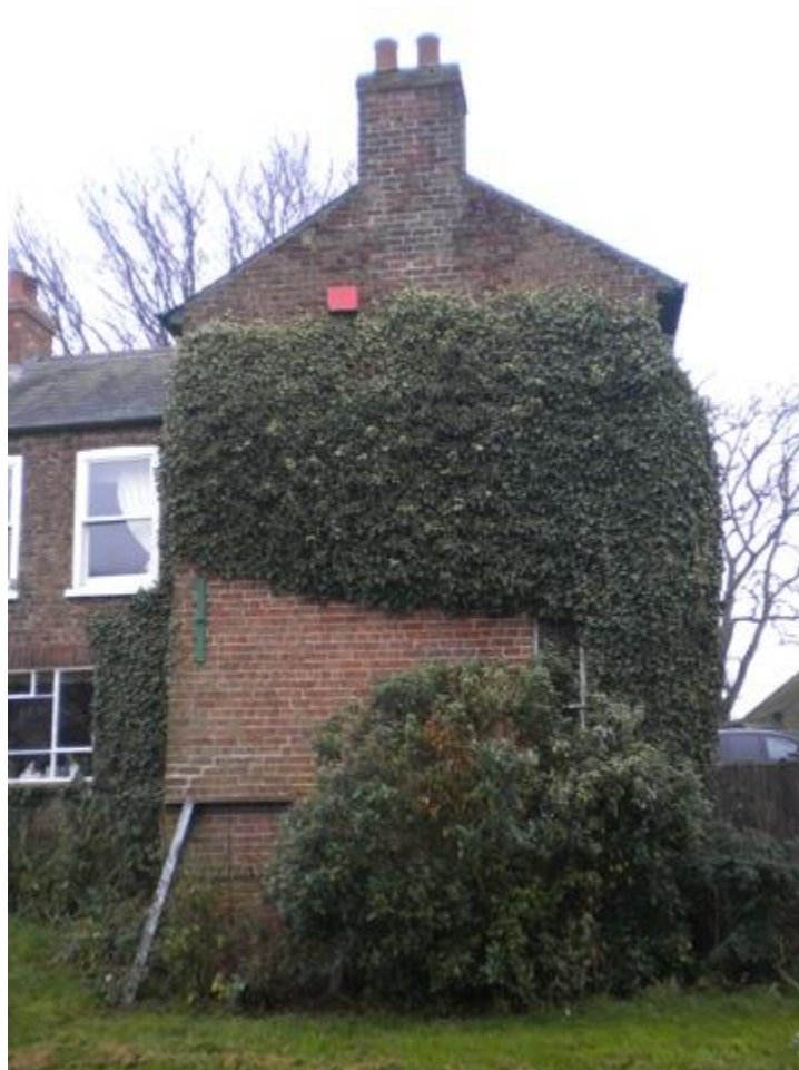
The rear projections showing the brickwork, which is in a poor state of repair, also with structural cracks. The guttering is predominantly plastic.
