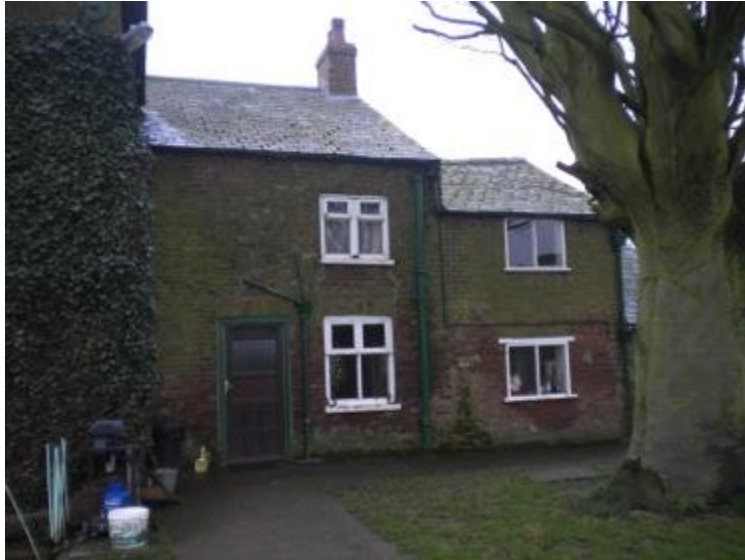
The rear projections showing the brickwork, which is in a poor state of repair, also with structural cracks. The guttering is predominantly plastic.
