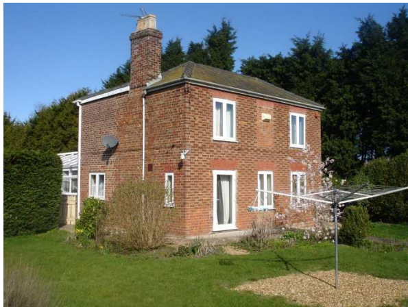
Front and side view of existing house (no. 279)
