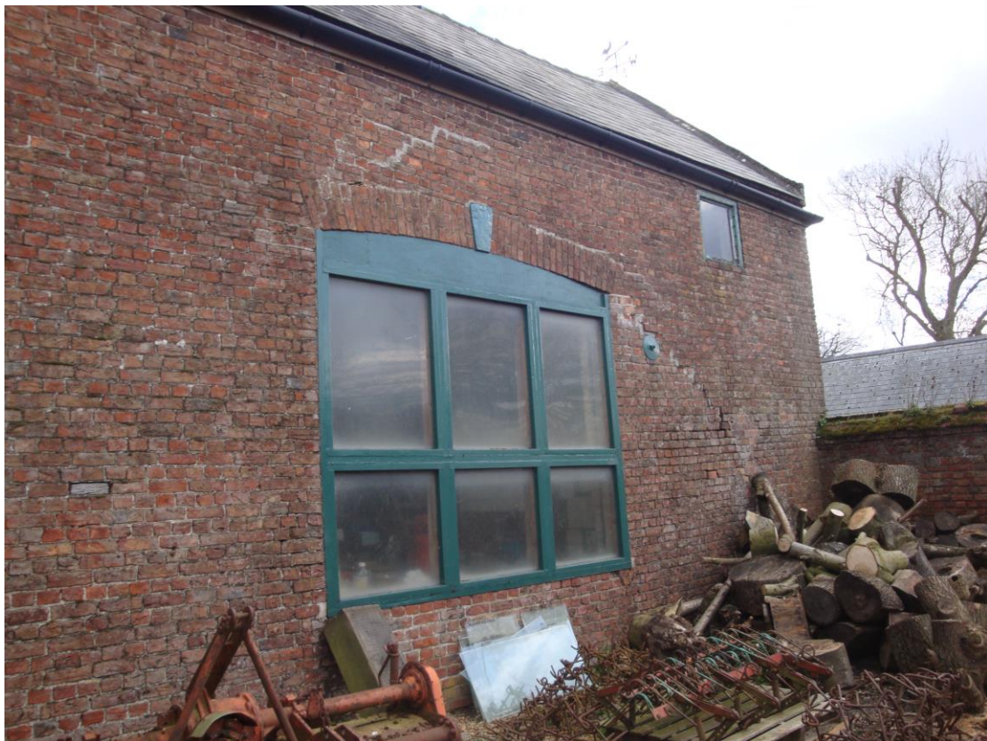
VIEW OF 2 STOREY BARN (1) LOOKING SE
