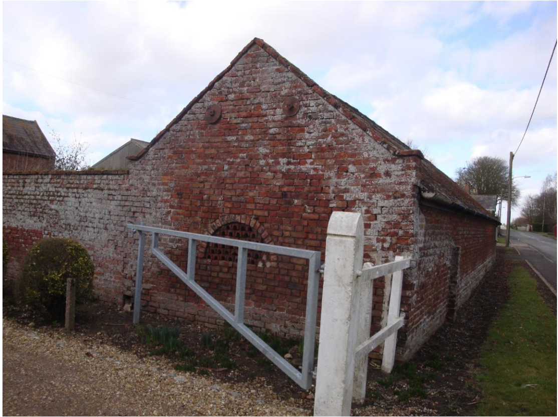
VIEW OF SINGLE STOREY BUILDING (3) FROM ACCESS
