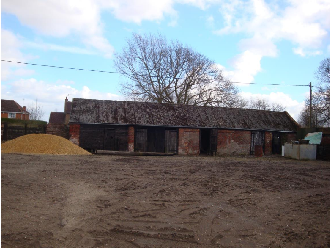
VIEW OF SINGLE STOREY BUILDING (3) LOOKING EAST
