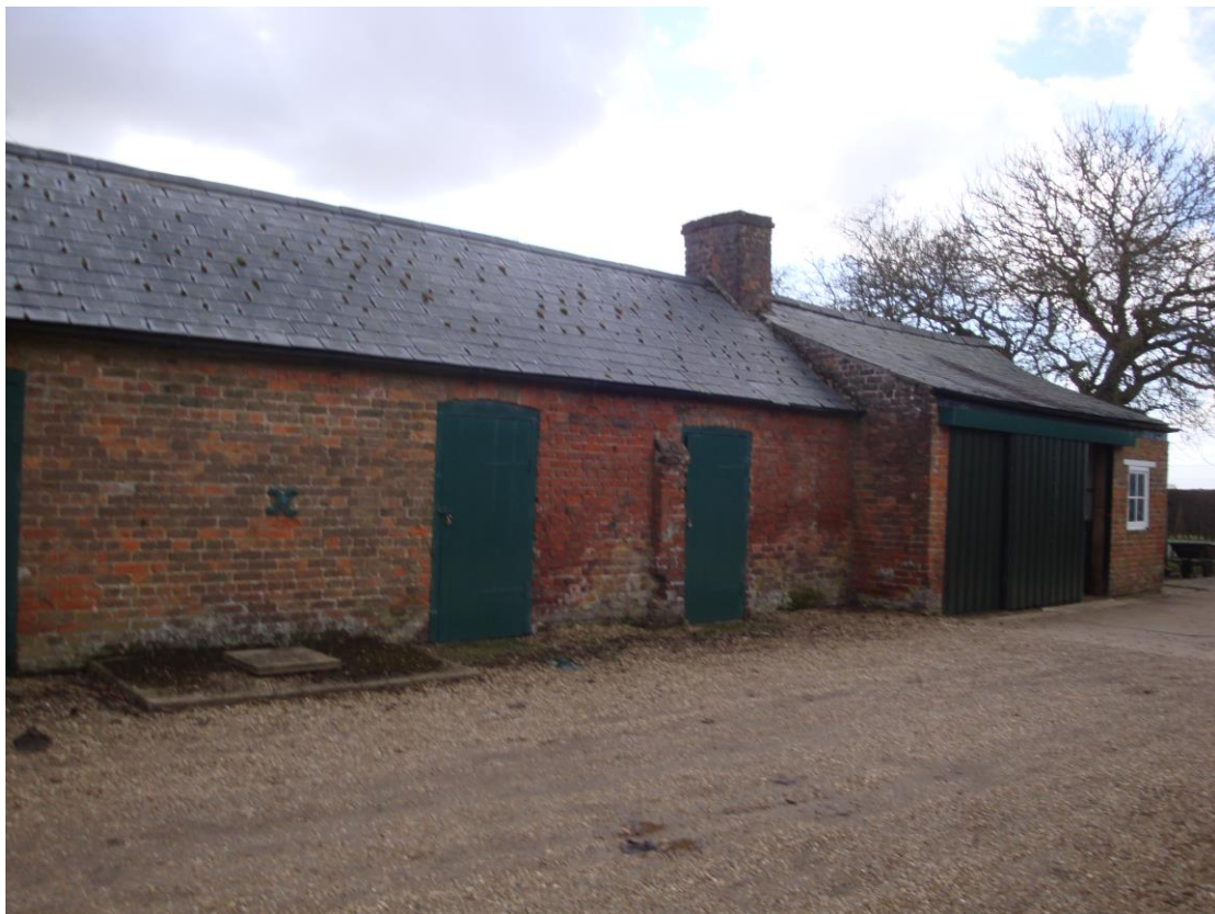
VIEW OF SINGLE STOREY BUILDING (2) LOOKING SW
