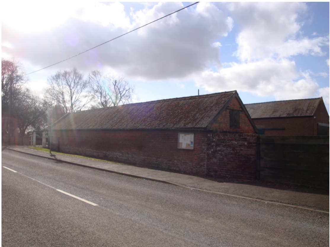
VIEW OF SINGLE STOREY BUILDING (3) FROM BROADGATE
