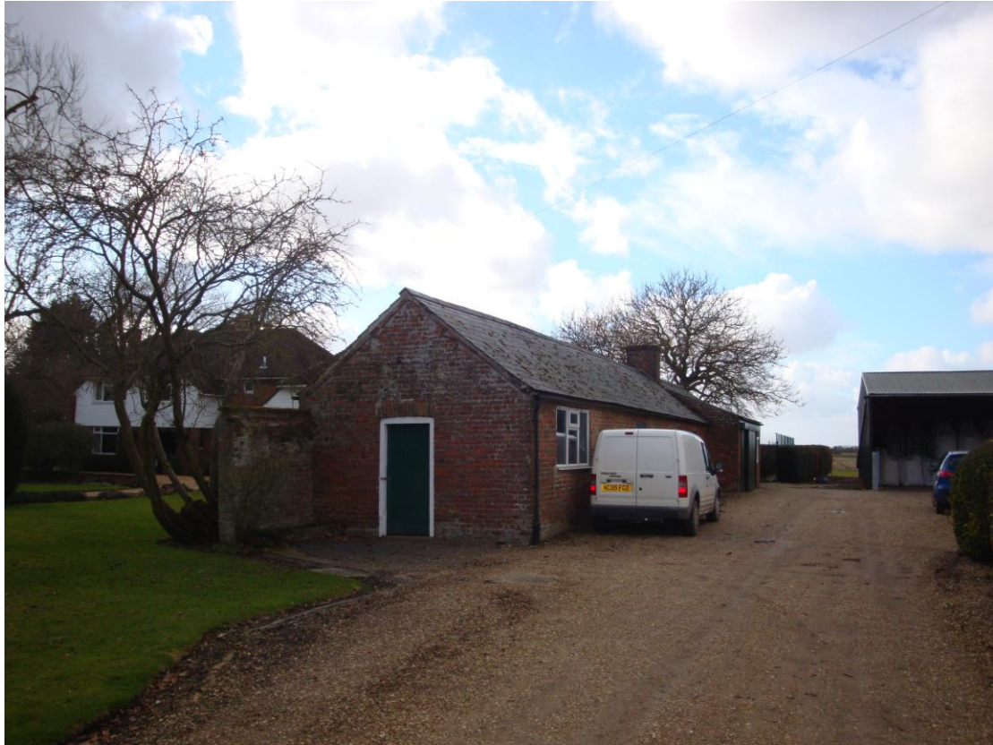
VIEW OF SINGLE STOREY BUILDING (2) FROM ACCESS
