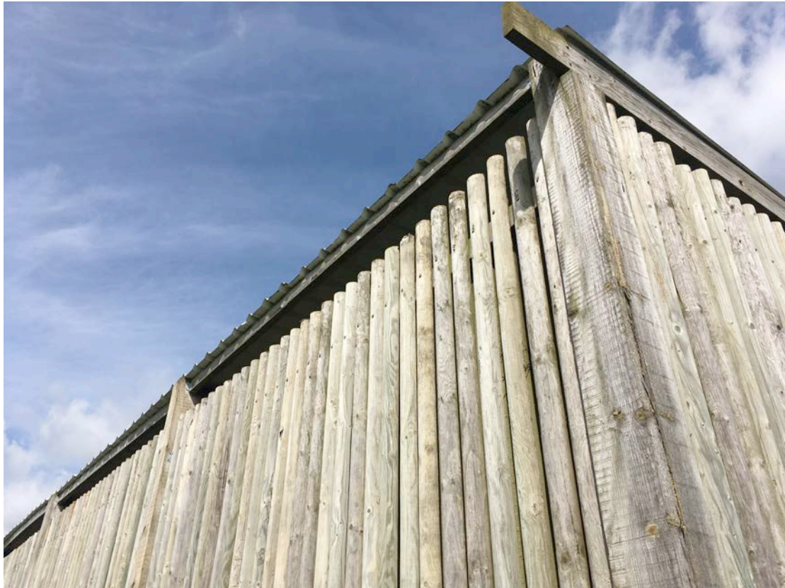
Image 9.0: Infill panel to exterior of structure
