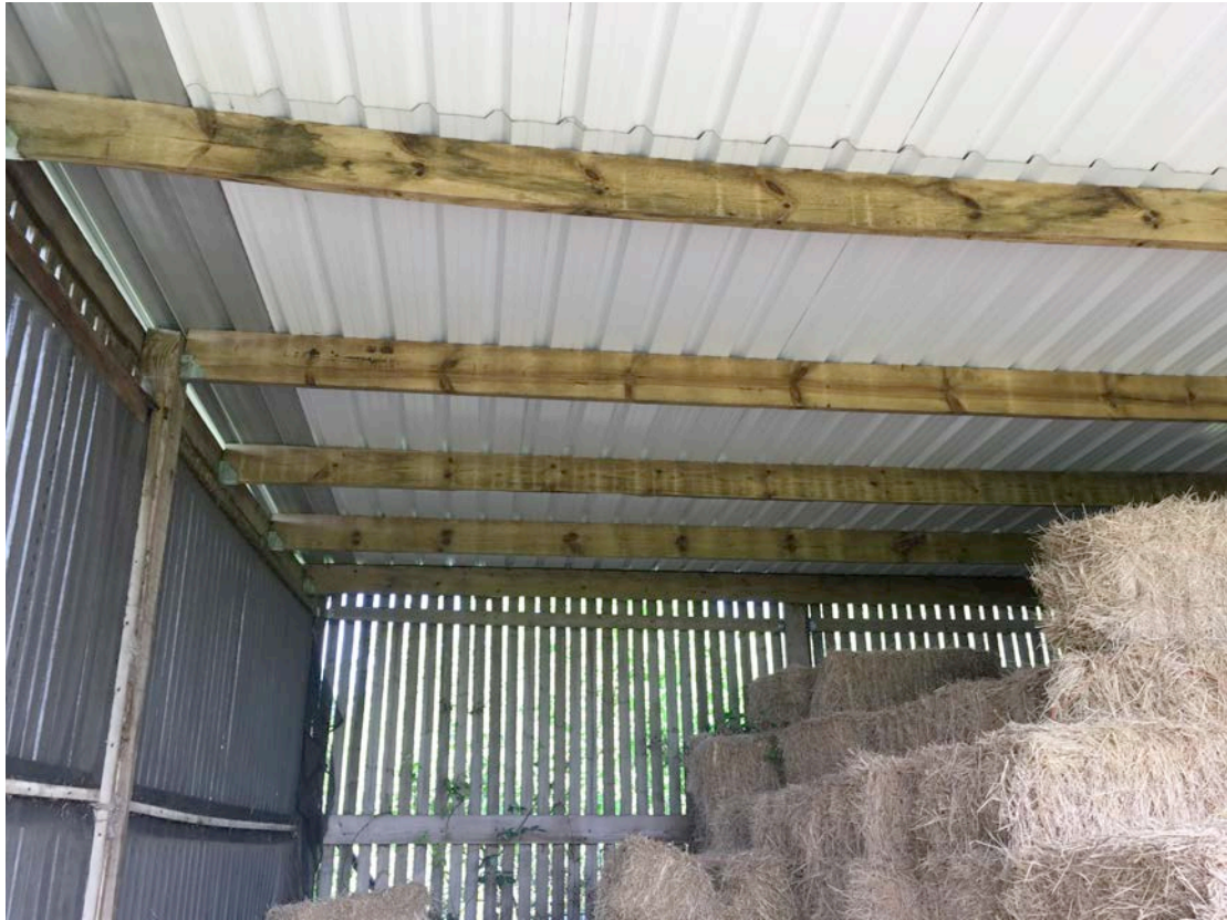
Image 7.0: View of rafters to rear half of structure, supported from columns and Primary beams.
