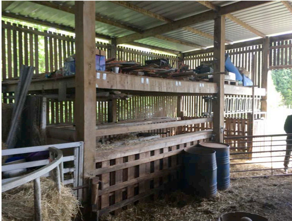
Image 4.0: View to interior of front half of structure.
