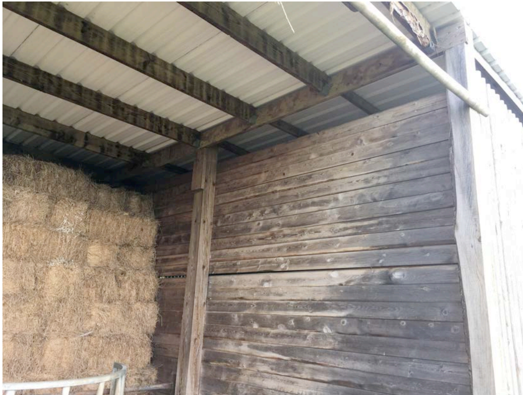
Image 6.0: View of timber columns to existing Barn.
