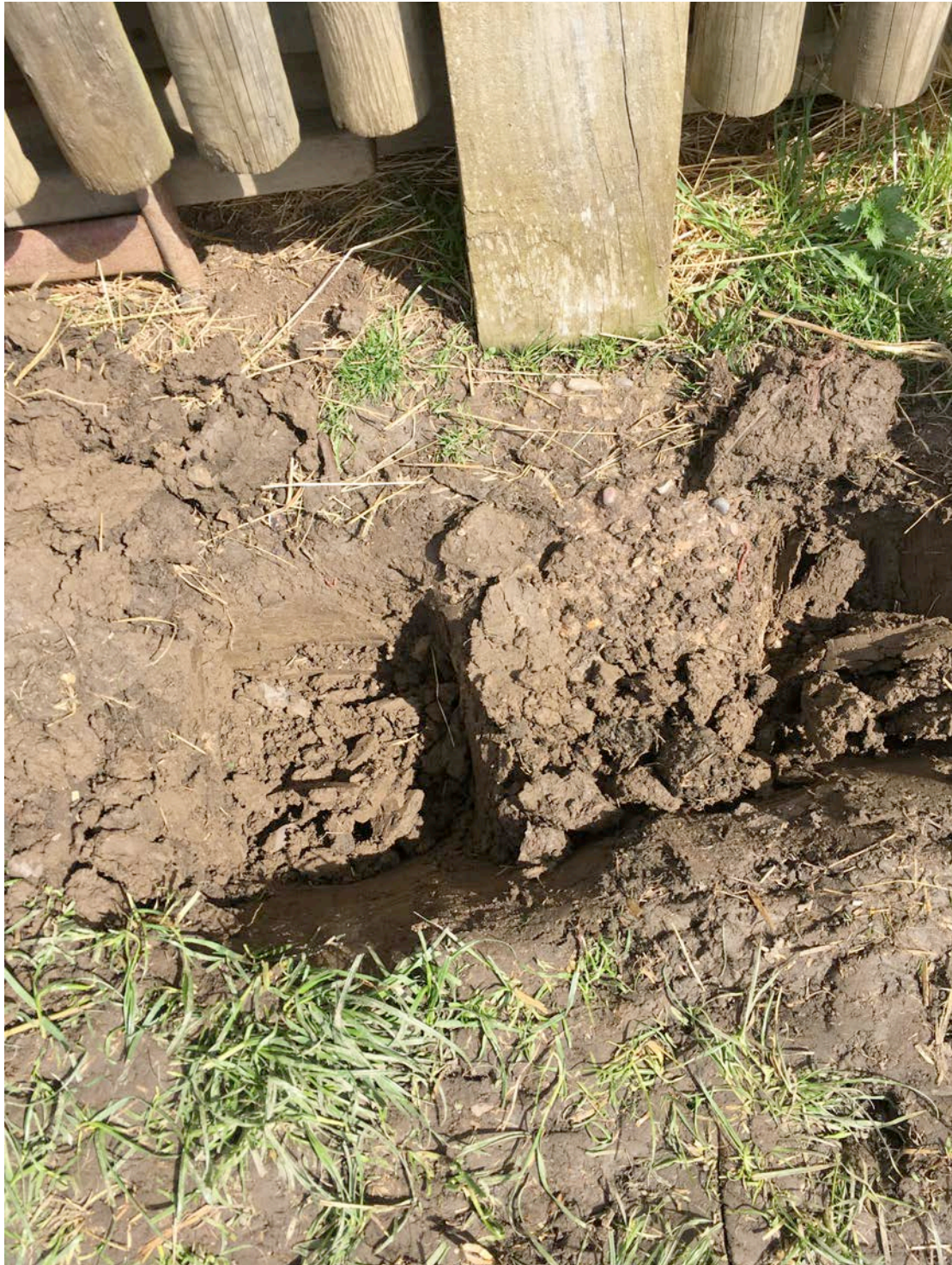
Image 8.0: View of Pad foundation to existing column.
