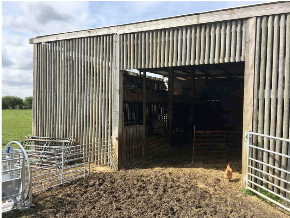
Image 3.0: Entrance to front of structure.
