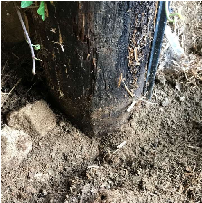
Photo 8. Timber post base
