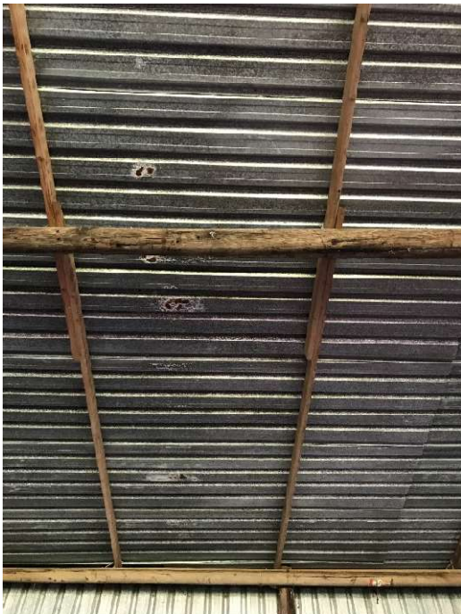
Photo 6. Roof cladding and supporting structural members
