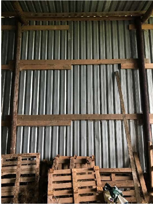
Photo 7. Side cladding and supporting structural members
