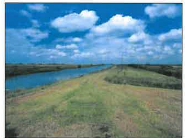
The Middle-level drain, in Norfolk, constructed in 1848. The hierarchy of embanked rivers and drains provide a strong influence throughout the area, often elevated above the low lying farmland, the level of which is falling due to drainage and farming practice.
