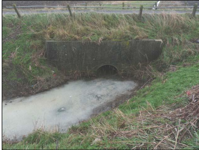
SHOWING THE CULVERT AT THE ROAD INTERSECTION, SANDY GATE (TN3)
