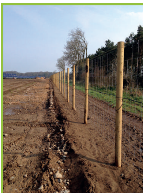
FENCING IN SITU
