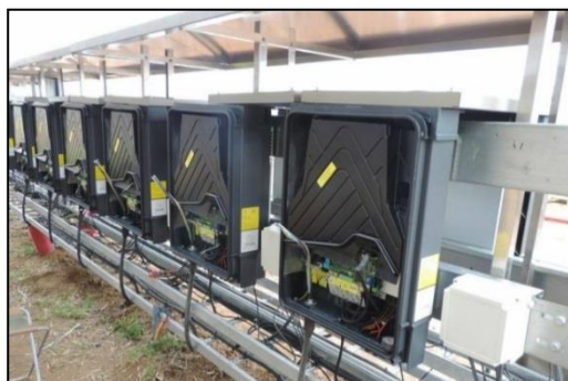
EXAMPLE: STRING INVERTERS WITHOUT COVER
