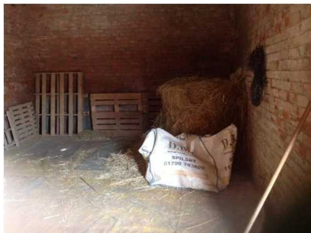
Interior of Main Barn – solid floors - used for storage of bedding / feed
