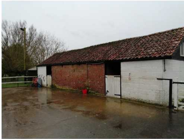
Detached Single storey building off concrete courtyard
