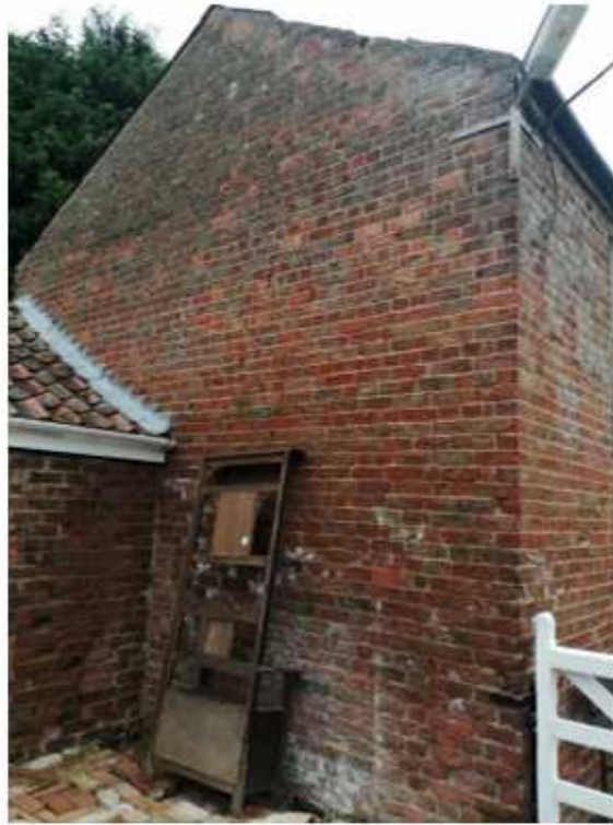
View 9 – west gable to main barn – stepped lead flashing at abutment with adjacent single storey
