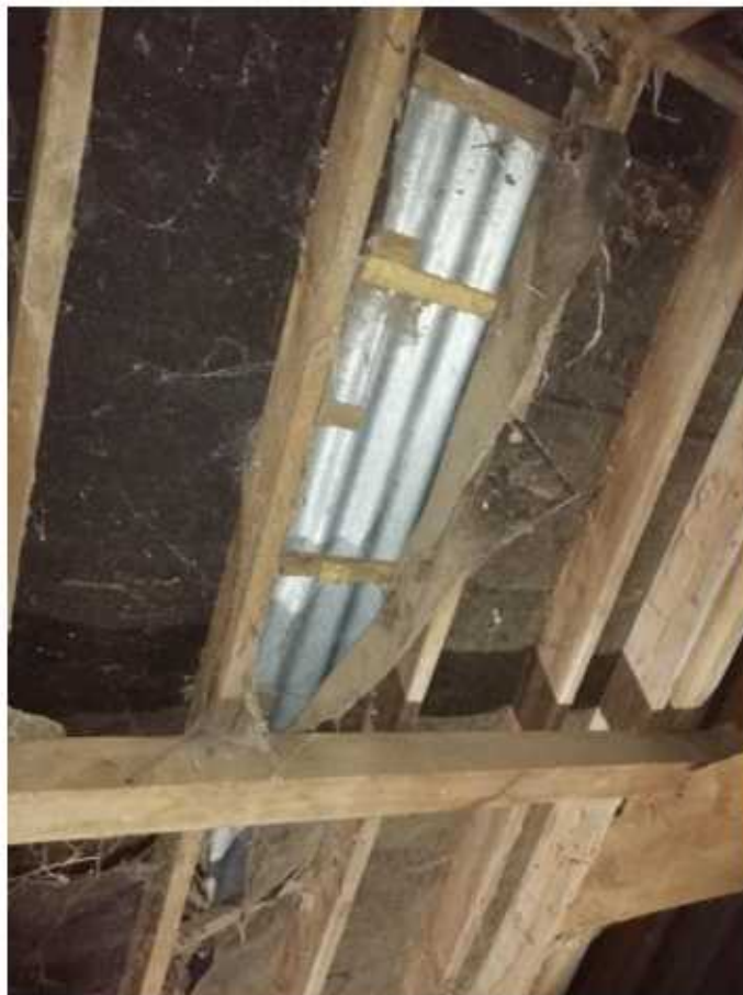
View 18 within loft area showing metal sheet roof cover
