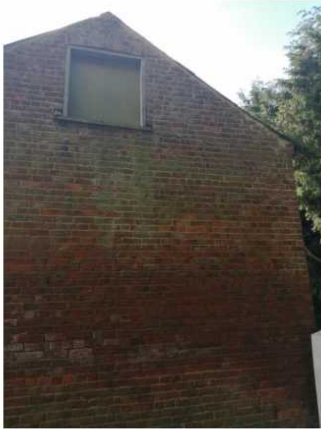
View 5 – gable to main barn east elevation -Single opening at ridge level
