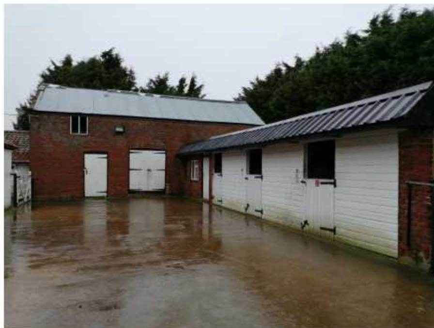
View 1 – view north-east towards buildings to be converted metal profile sheeting to main barn roof slope and single storey building
