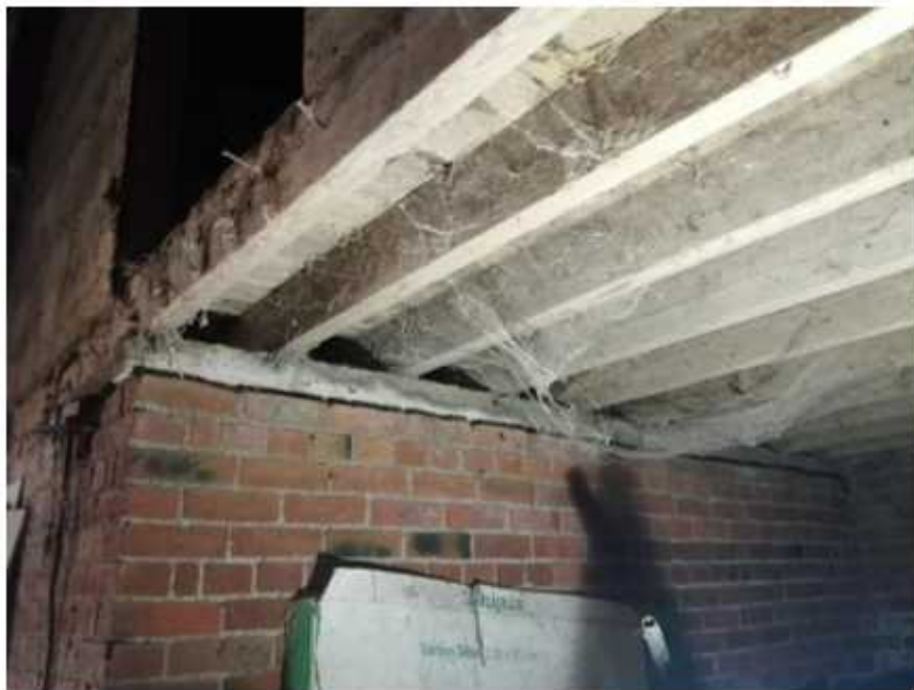
View 16 – timber floor support to loft area
