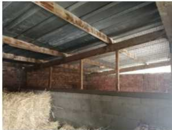
View 23 – middle stable showing internal partition and metal sheet roof cover
