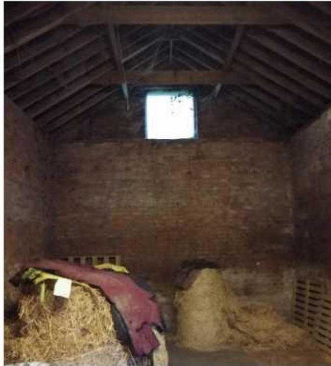
View 13 – Internal view in main barn – traditional raised collar and purlin roof Gable wall reduced to 225mm brickwork above wall plate level
