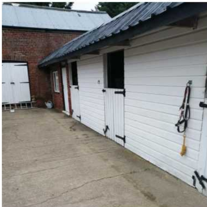
View 12 – elevation of boarded stable element of single storey
