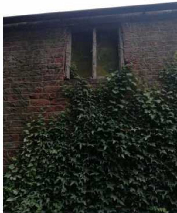
View 8 – existing loft window to main barn
