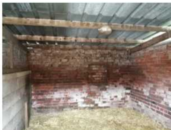
View 24 – end stable showing original brick rear and side walls
