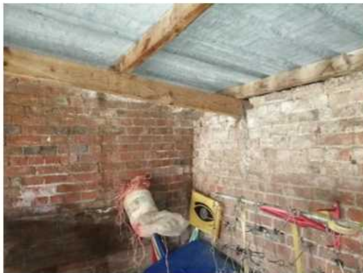
View 20 – brick built store – roof cover
