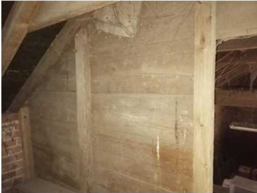
View 17 – horizontal boarded partition to loft area
