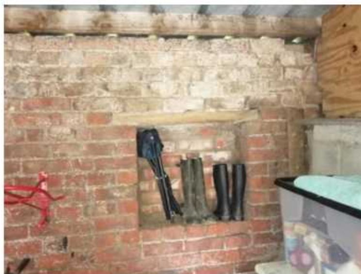
View 21 – brick built store timber lintelled recess rear wall
