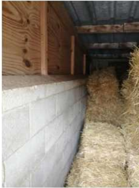
View 22 – internal view of stable showing blockwork and timber partition
