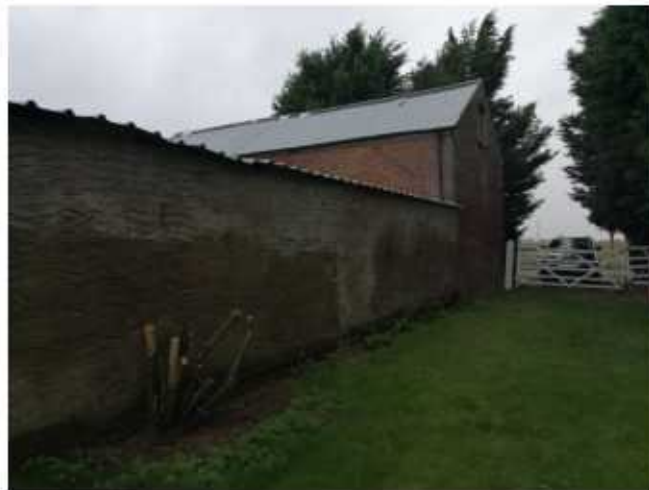
View 3 – rear elevation of single storey element and gable of main barn
