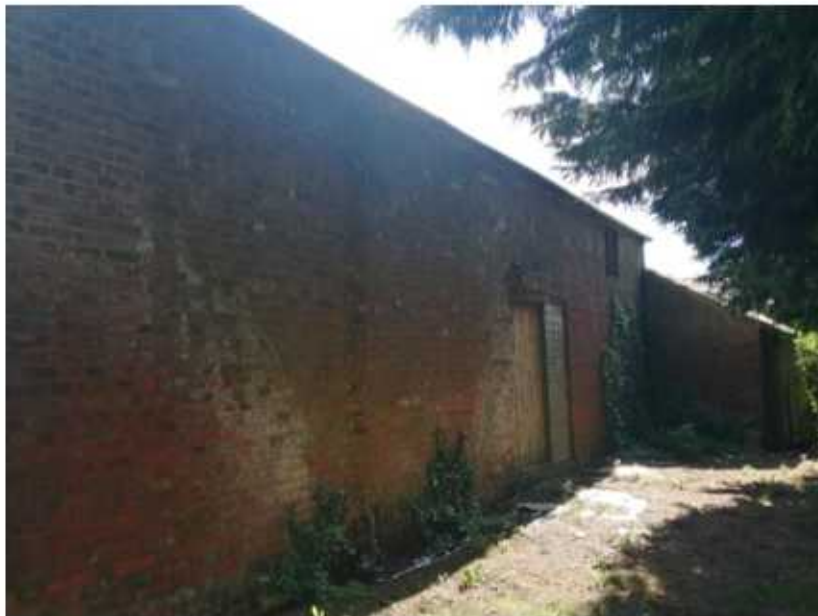
View 6 – main barn elevation towards Horsemoor Drove
