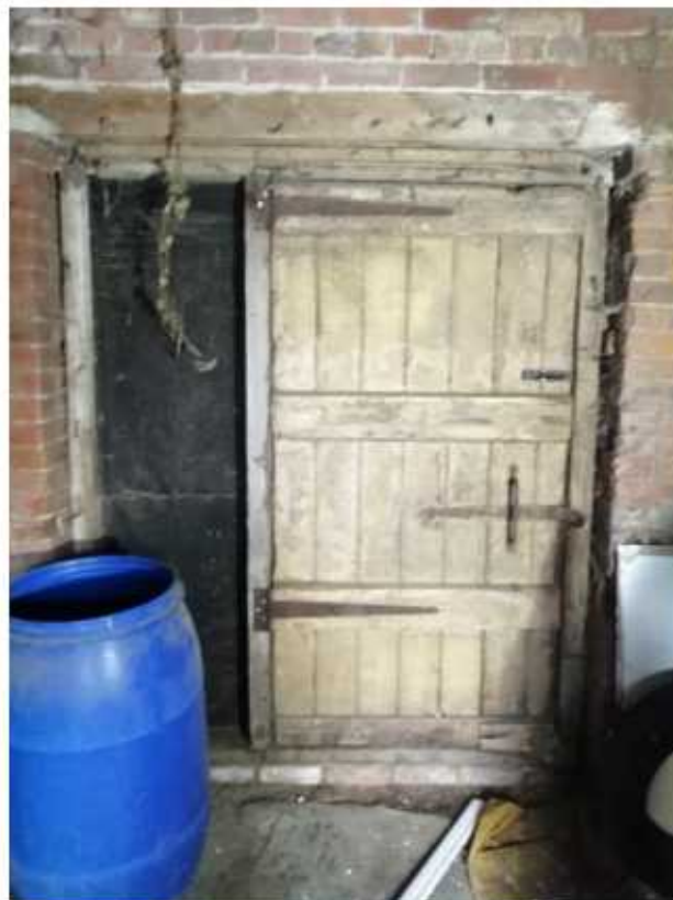
View 14 – Internal view of opening to north elevation of main barn
