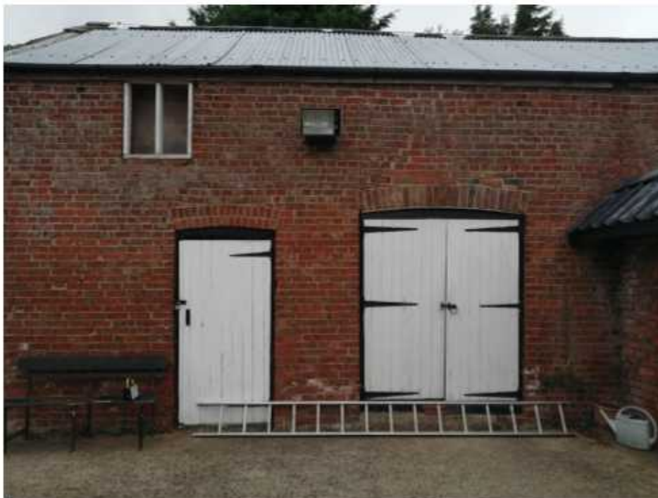
View 10 – south east elevation to main barn – brick arches to lower storey openings
