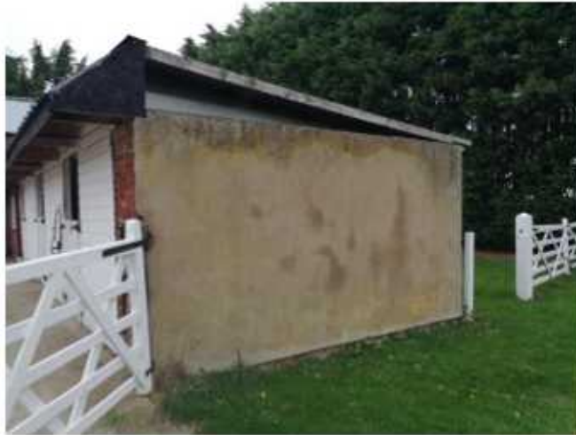
View 2 – gable end of single storey building
