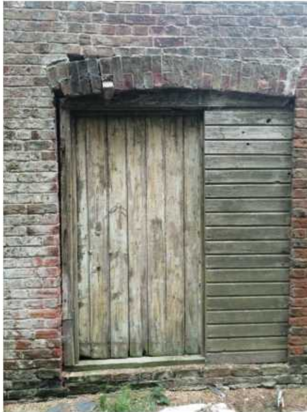
View 7 – Existing Ground Floor opening to north elevation of main barn
