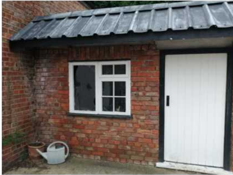
View 11 – elevation of single storey store building
