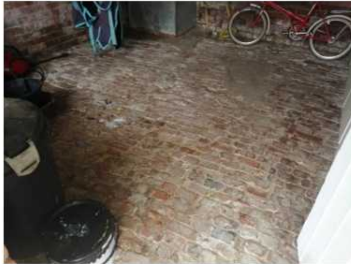
View 19 – floor to single storey brick built store
