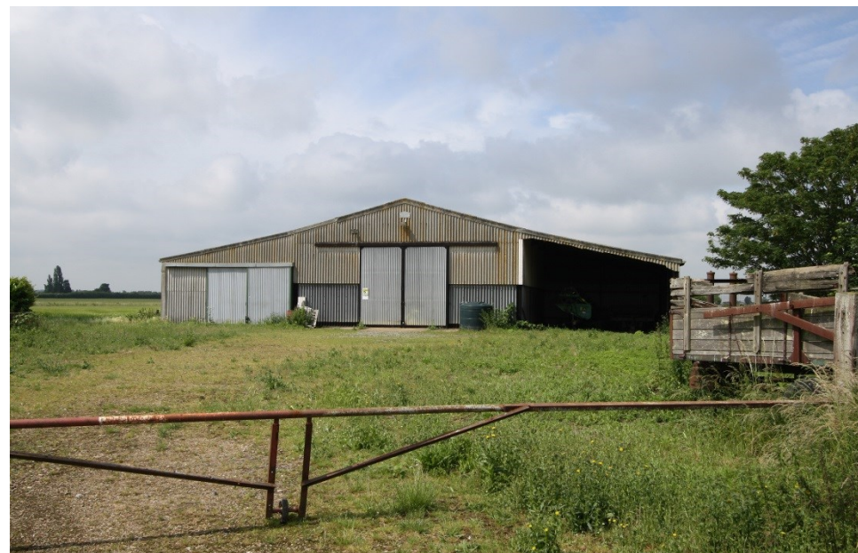
Modern Steel Frame Barn along Childersgate Lane
