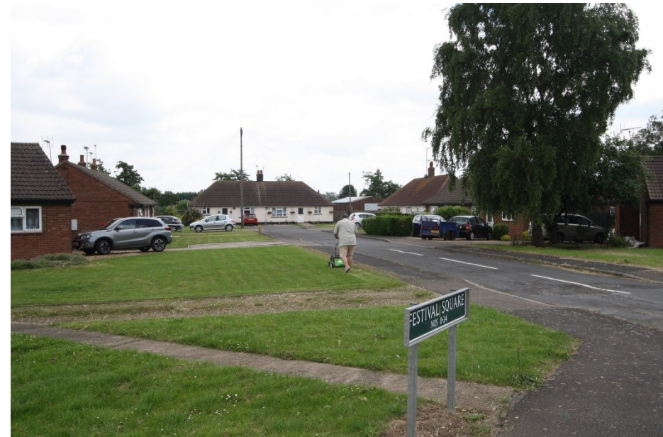
Local Authority Bungalow Cul-De-Sac development off Chapel Gate (Festival Gardens)
