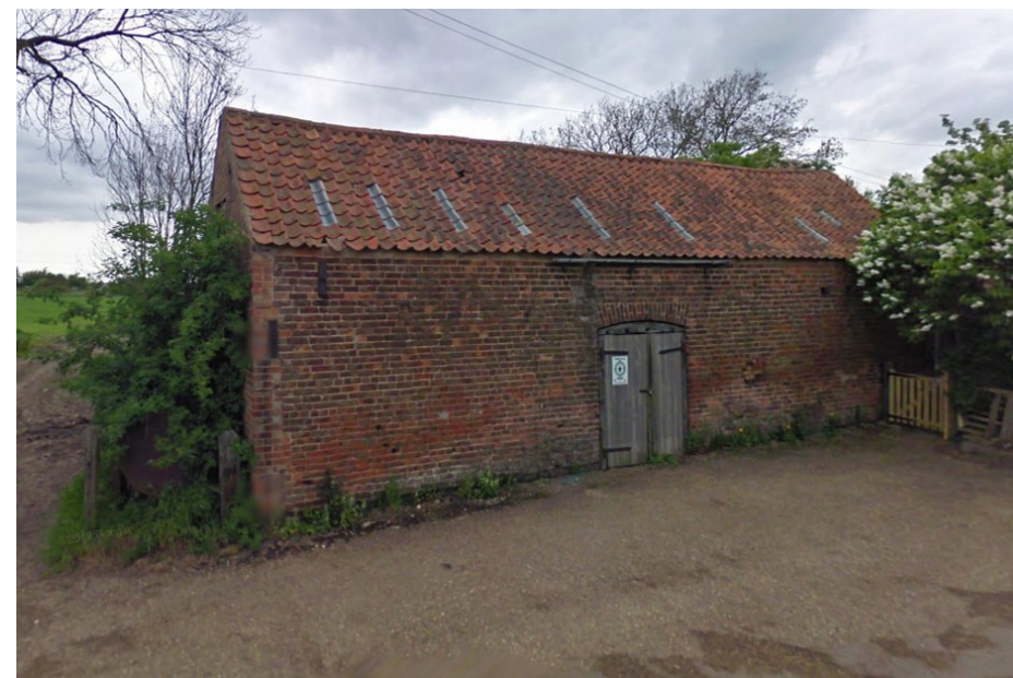
Brick Barn adjacent to Farmhouse at the Junction of Fishergate and Horsemoor Drove
