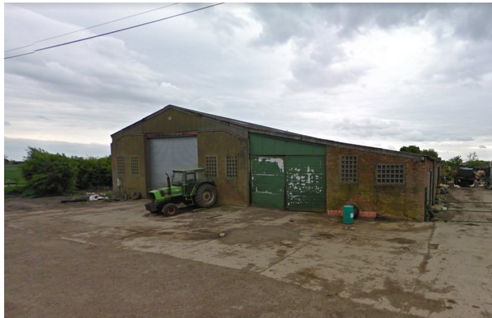
Brick and Angle Iron Barn on Old Fendike
