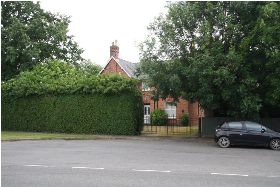
Image of Victorian House off Chapel Gate
