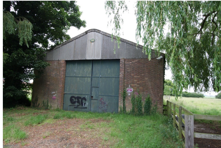
Modern Steel Frame Barn with Brickwork walls along Bells Drove
