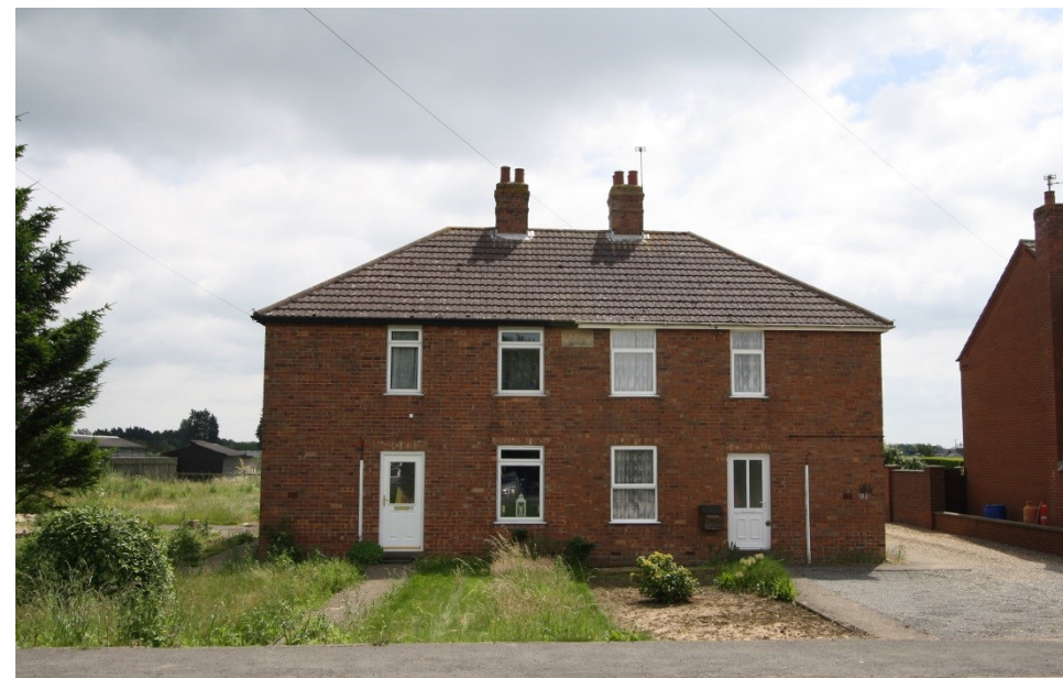
Local Authority Housing in Linear Form along Chapel Gate
