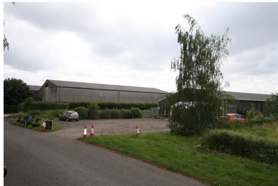
Former Johnsons Grain Stores along Bells Drove, Modern Steel Frame, Clad Barns
