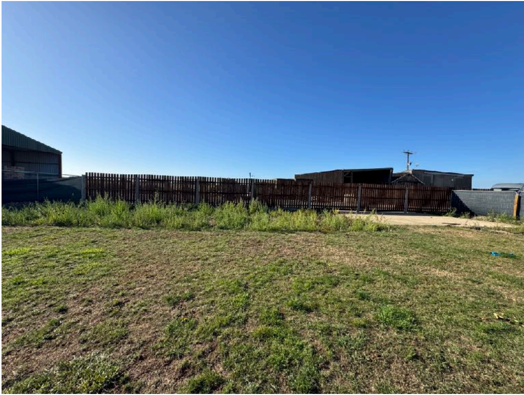
Figure 5: Weed growth present in the informal stoned up hardstanding adjacent to the main lawn
