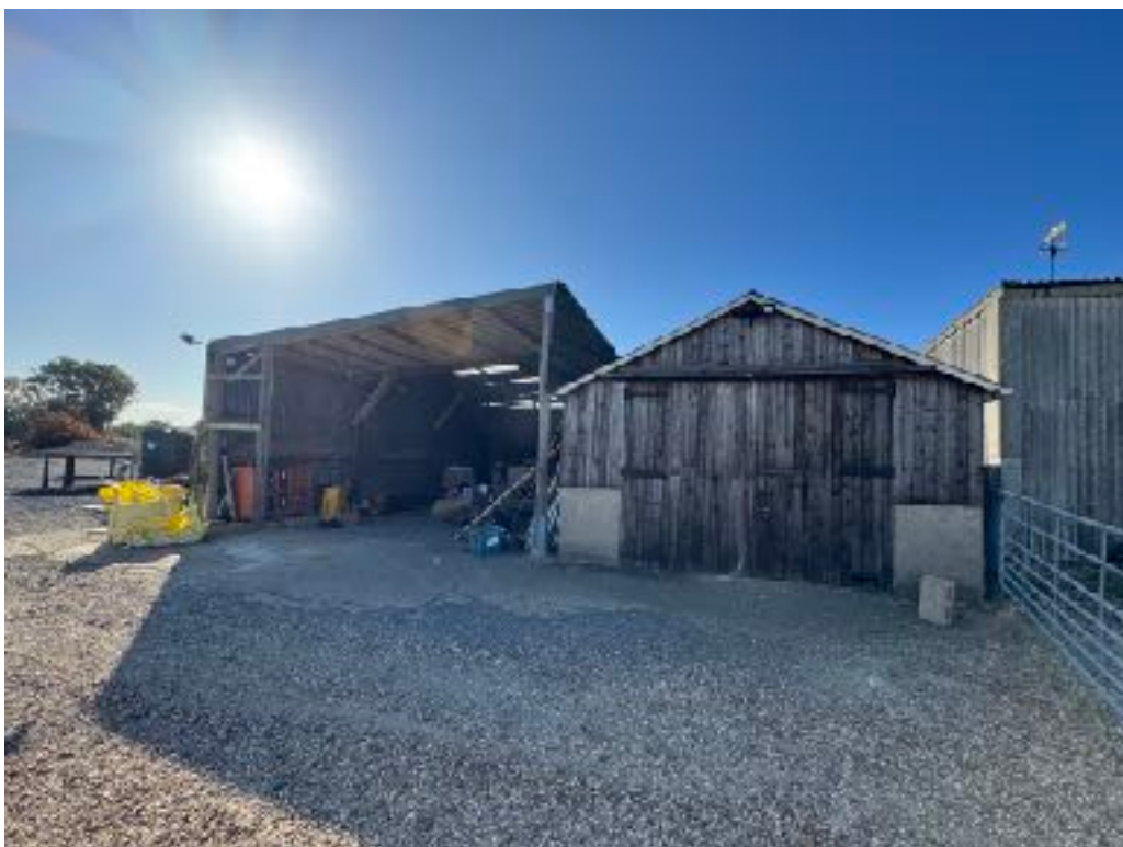
Figure 9: Various outbuildings on South West corner of the site
