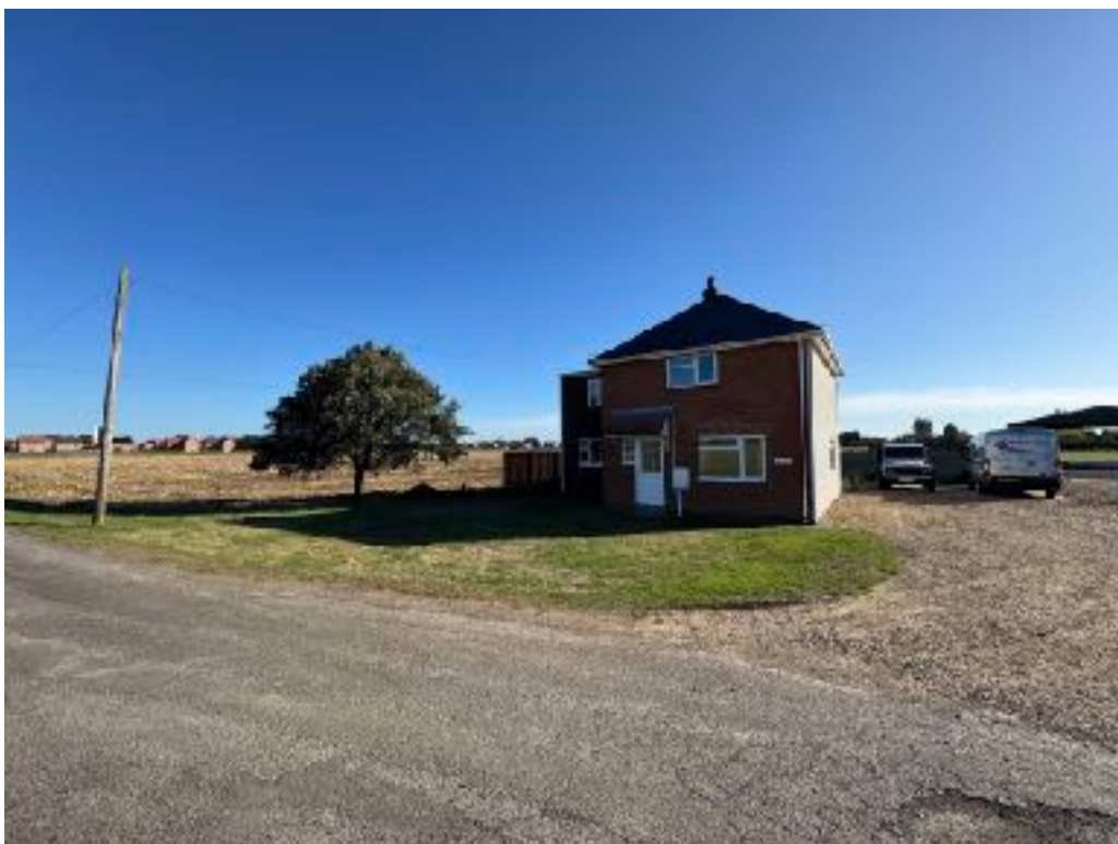
Figure 7: Lynn House viewed from Mill Lane (West facing elevation)
