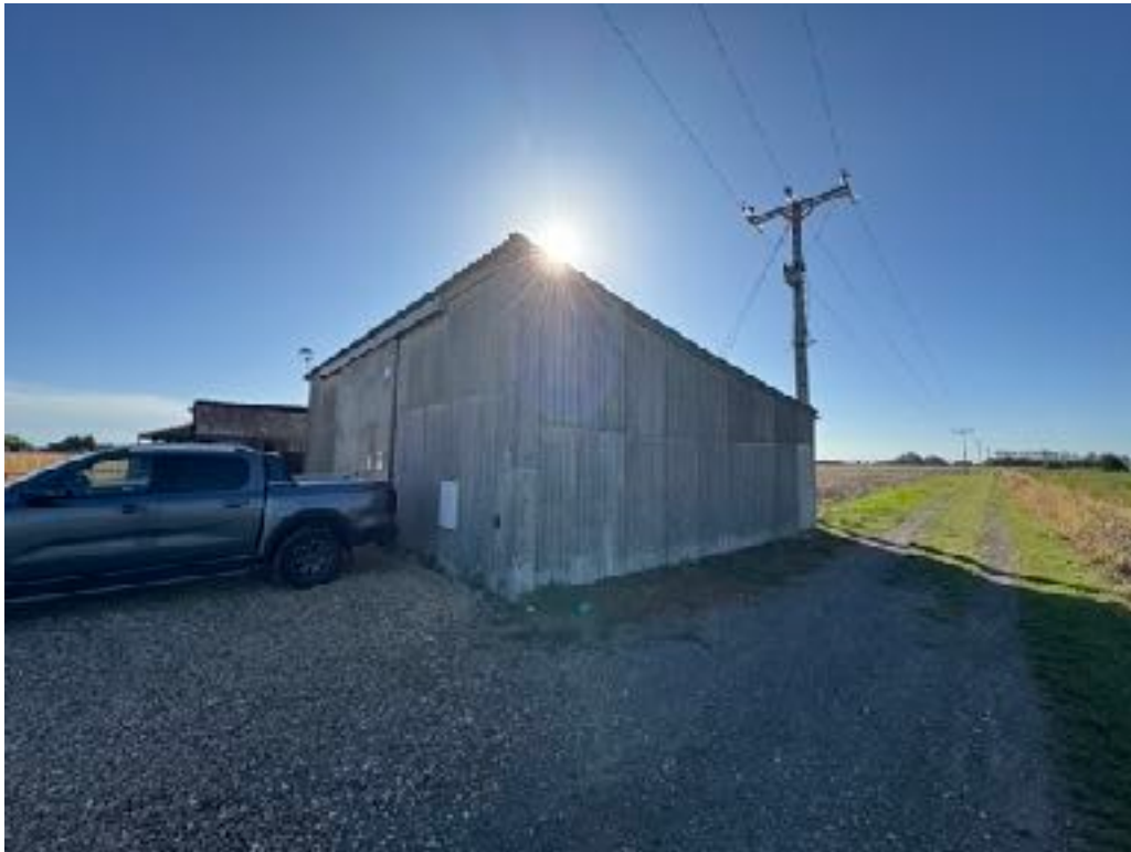
Figure 6: Existing Outbuilding and Taylor's Drove beyond (South facing)
