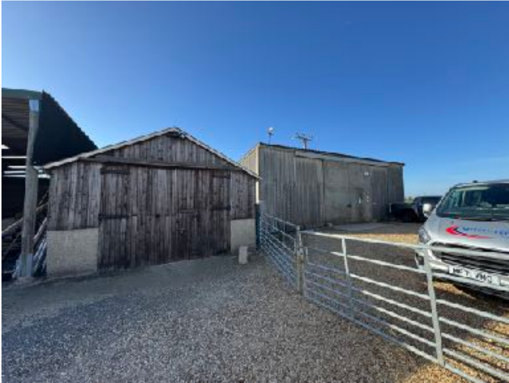
Figure 10: Various outbuildings on South West corner of the site
