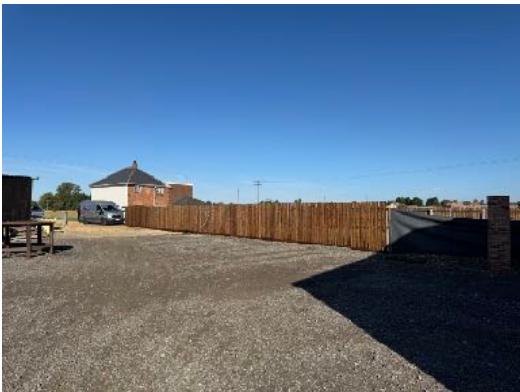
Figure 13: Boundary fence separating the residential areas from the commercial areas
