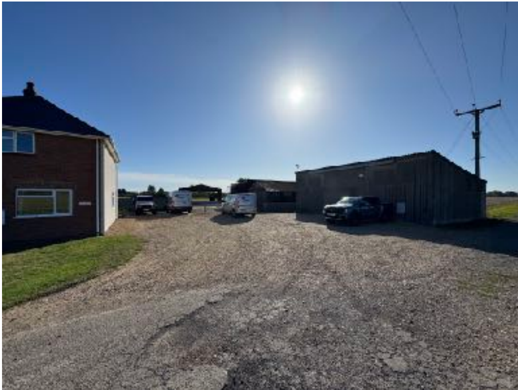
Figure 8: Vehicle driveway viewed from Mill Lane (West facing elevation)
