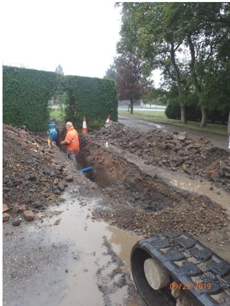
Plate 41: Excavation of the third section of service trench, from the north
