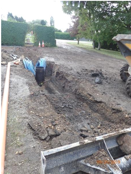
Plate 49: Excavation of the third section of service trench, from the north
