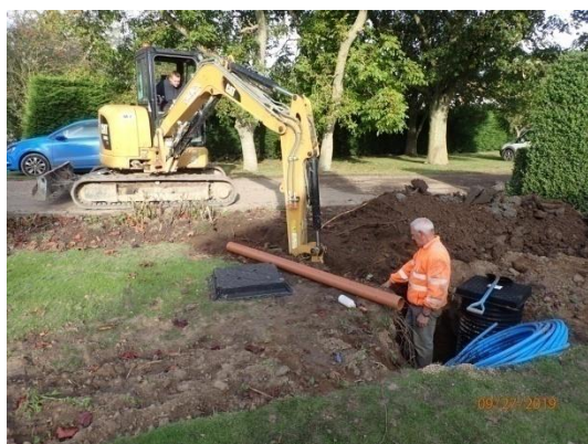
Plate 139: Excavation of the fourth section of service trench, from the south
