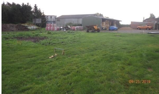
Plate 57: Pre-groundworks, from the east
