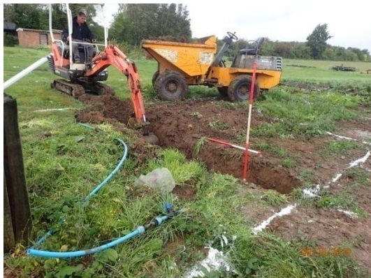
Plate 59: Excavation of the foundations, from the south-east
