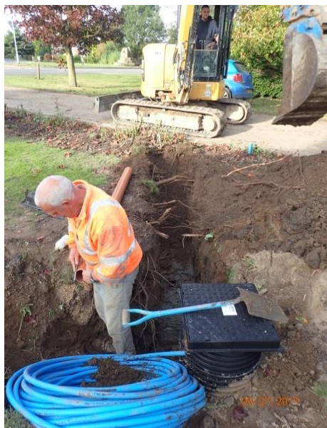
Plate 138: Excavation of the fourth section of service trench, from the east
