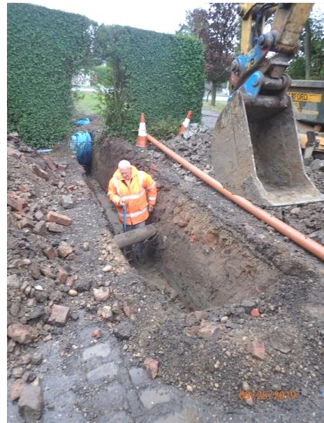
Plate 39: Excavation of the third section of service trench, from the north
