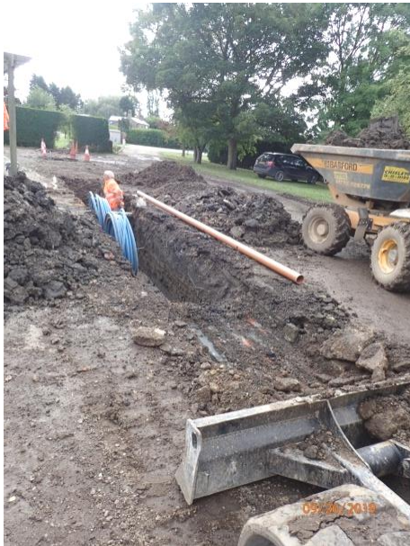
Plate 130: Excavation of the third section of service trench, from the north
