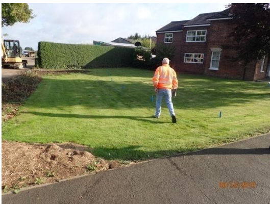
Plate 9: Pre-groundworks, from the south
