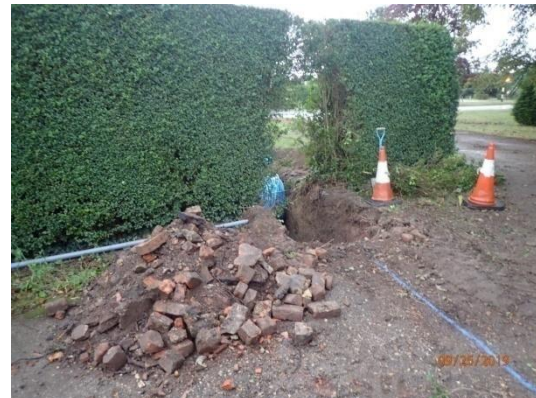
Plate 34: Excavation of the third section of service trench, from the north
