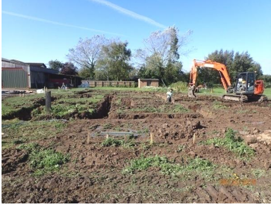
Plate 113: Excavation of the foundations, from the east
