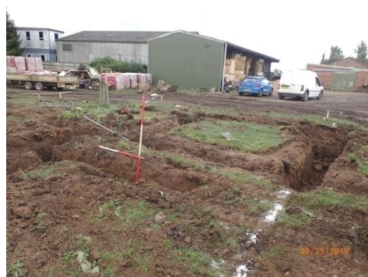
Plate 83: Excavation of the foundations, from the north
