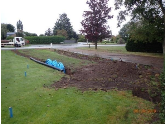
Plate 21: Excavated and partially backfilled first section of service trench, from the north
