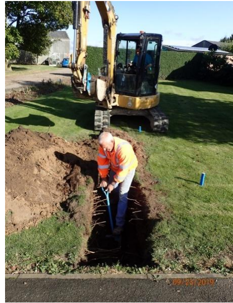
Plate 10: Excavation of the first section of service trenching, from the south
