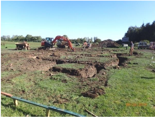
Plate 114: Excavation of the foundations, from the west
