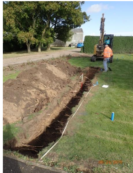
Plate 16: Excavation of the first section of service trenching, from the south
