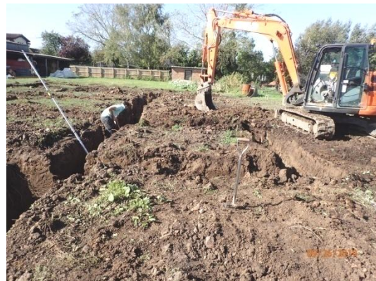
Plate 112: Excavation of the foundations, from the east
