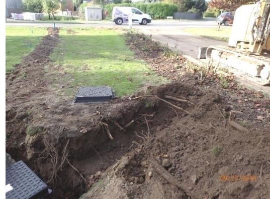
Plate 135: Excavation of the fourth section of service trench, from the north
