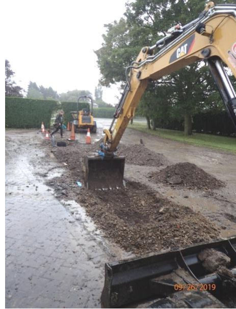
Plate 115: Excavation of the third section of service trench, from the north
