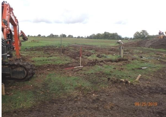
Plate 78: Excavation of the foundations, from the south
