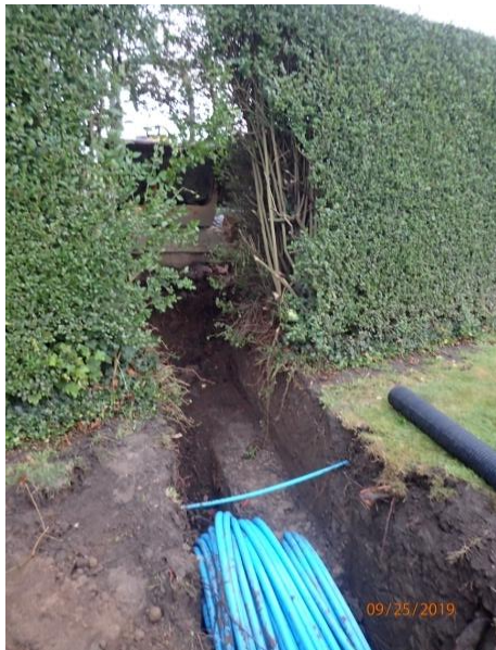
Plate 28: Excavation of the second section of service trench through the hedgerow, from the south
