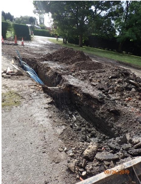
Plate 126: Excavation of the third section of service trench, from the north
