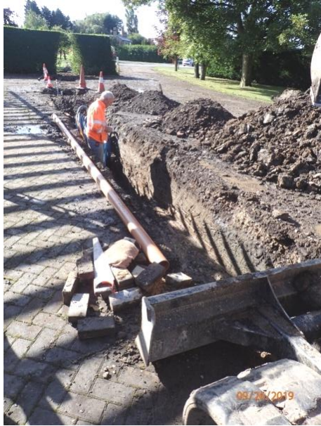
Plate 121: Excavation of the third section of service trench, from the north
