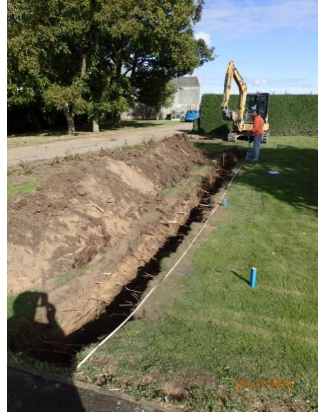
Plate 19: Excavation of the first section of service trenching, from the south
