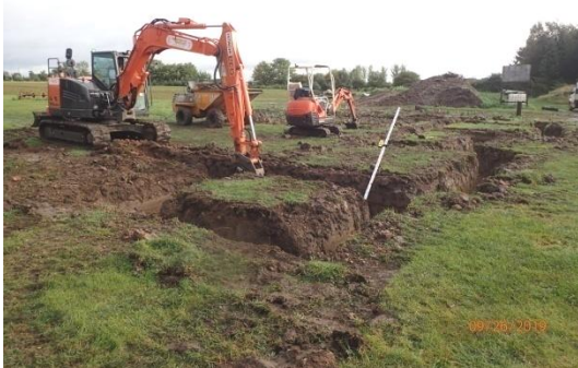
Plate 97: Excavation of the foundations, from the west
