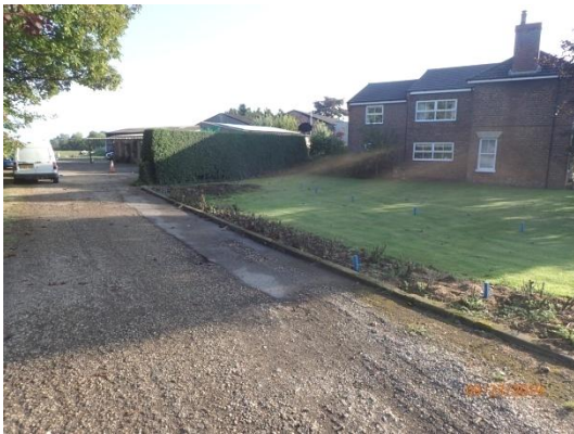
Plate 8: Pre-groundworks, from the south
