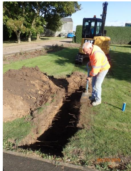
Plate 11: Excavation of the first section of service trenching, from the south
