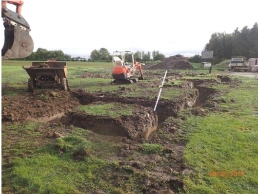
Plate 96: Excavation of the foundations, from the west
