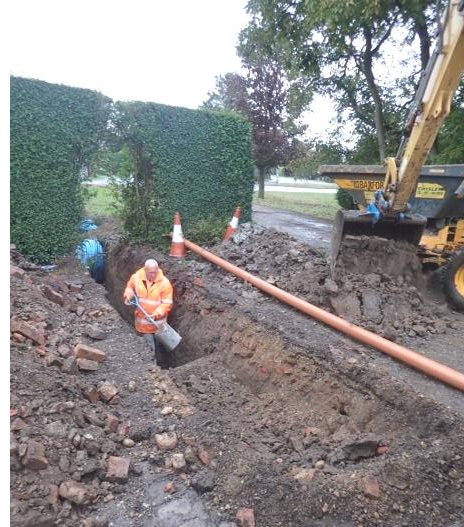
Plate 38: Excavation of the third section of service trench, from the north
