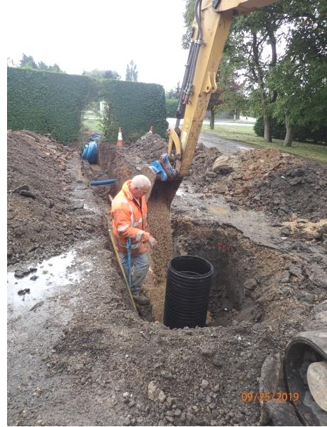
Plate 46: Excavation of the third section of service trench, from the north
