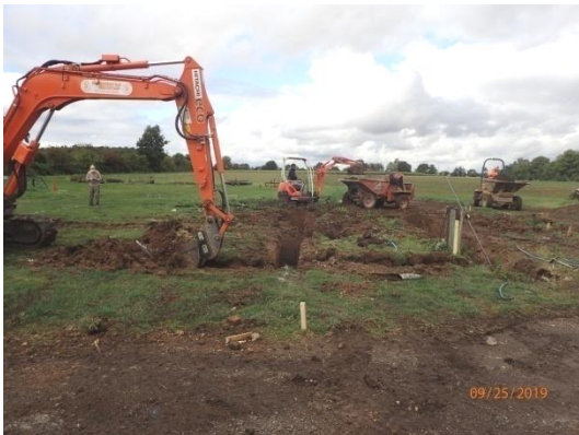
Plate 73: Excavation of the foundations, from the south
