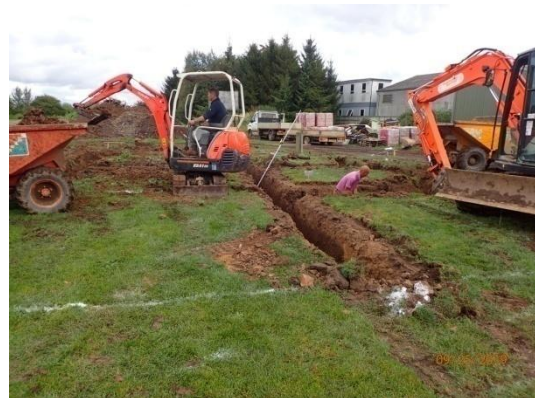
Plate 82: Excavation of the foundations, from the west
