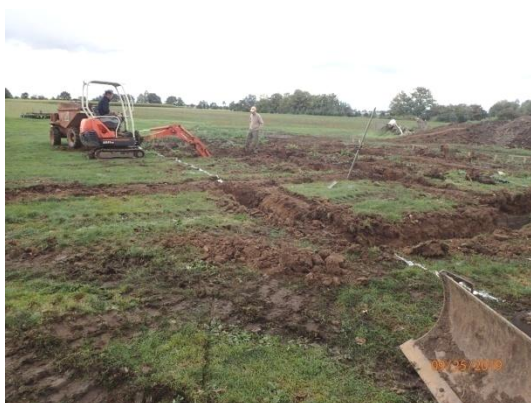
Plate 80: Excavation of the foundations, from the south
