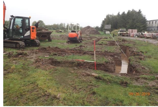
Plate 93: Excavation of the foundations, from the west
