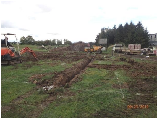
Plate 79: Excavation of the foundations, from the west
