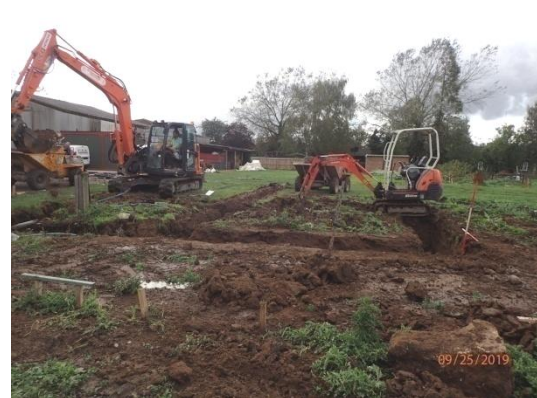
Plate 70: Excavation of the foundations, from the east
