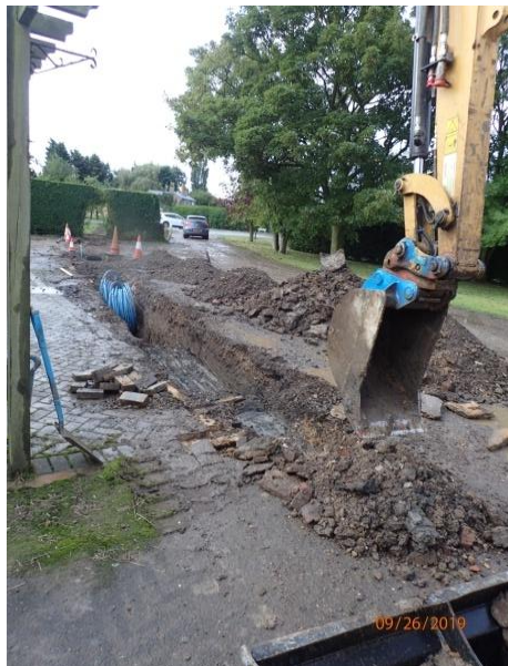
Plate 118: Excavation of the third section of service trench, from the north
