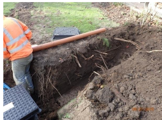
Plate 137: Excavation of the fourth section of service trench, from the north
