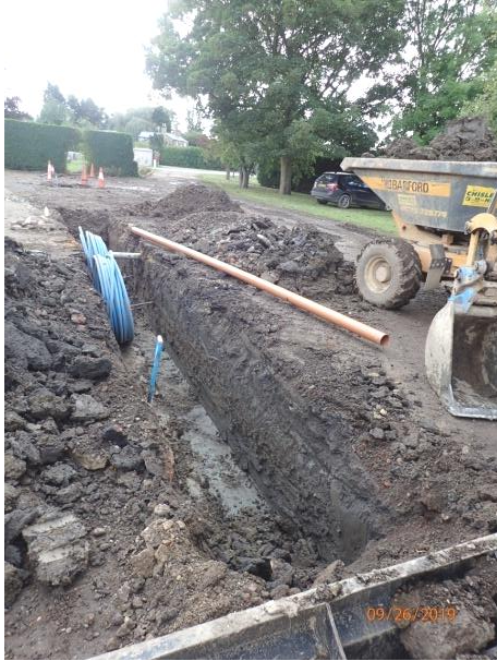
Plate 133: Excavation of the third section of service trench, from the north
