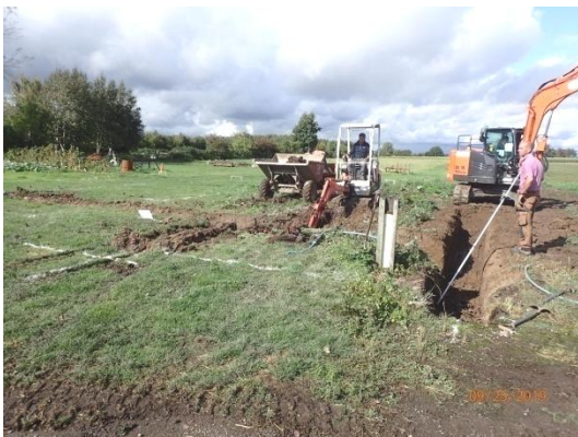
Plate 68: Excavation of the foundations, from the south
