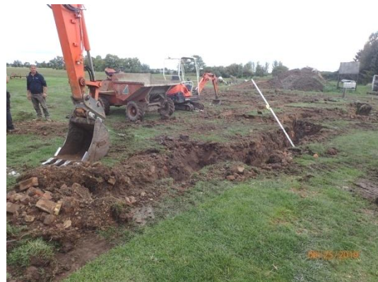
Plate 88: Excavation of the foundations, from the south-west
