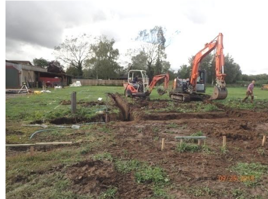
Plate 69: Excavation of the foundations, from the east
