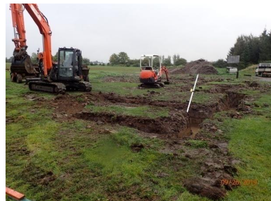
Plate 95: Excavation of the foundations, from the west
