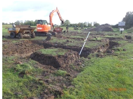
Plate 100: Excavation of the foundations, from the west
