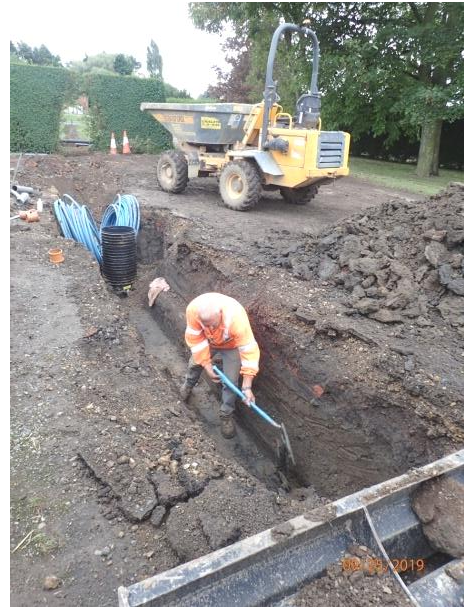
Plate 50: Excavation of the third section of service trench, from the north
