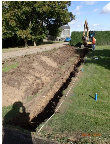
Plate 20: Excavation of the first section of service trenching, from the south
