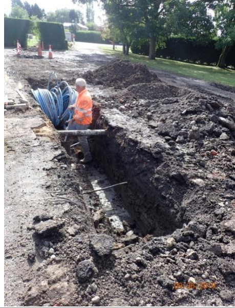
Plate 127: Excavation of the third section of service trench, from the north
