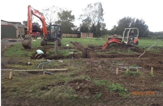
Plate 72: Excavation of the foundations, from the east
