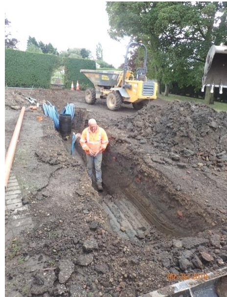
Plate 51: Excavation of the third section of service trench, from the north
