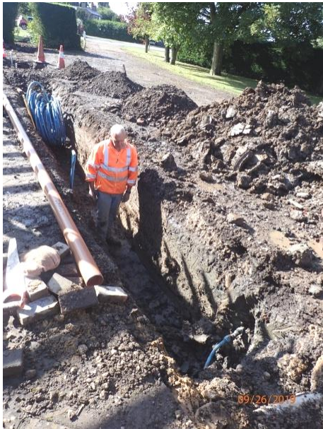
Plate 122: Excavation of the third section of service trench, from the north
