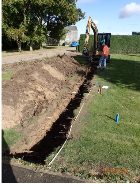
Plate 17: Excavation of the first section of service trenching, from the south
