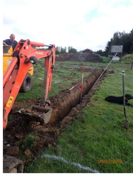
Plate 64: Excavation of the foundations, from the west
