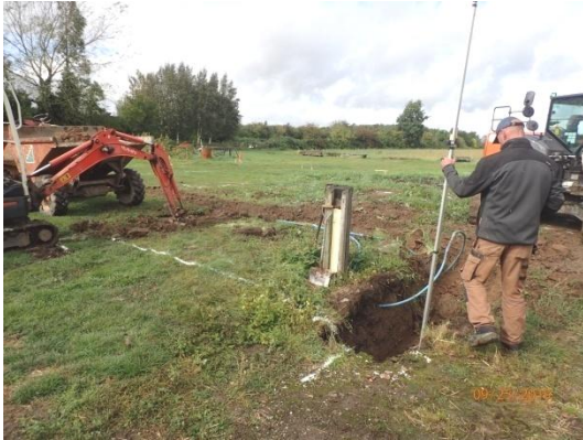
Plate 66: Excavation of the foundations, from the south-east
