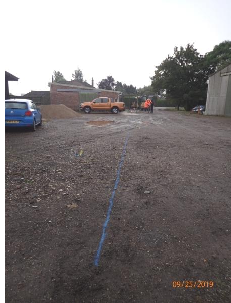
Plate 33: Set out third section of service trench, from the south
