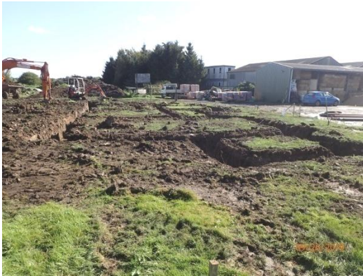
Plate 109: Excavation of the foundations, from the west
