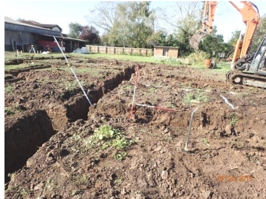
Plate 111: Excavation of the foundations, from the east
