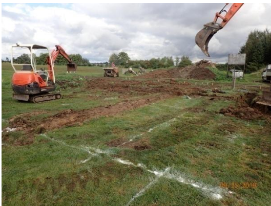
Plate 74: Excavation of the foundations, from the south-west
