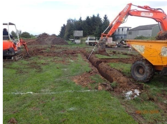
Plate 76: Excavation of the foundations, from the west
