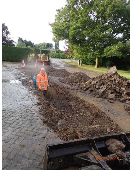
Plate 117: Excavation of the third section of service trench, from the north
