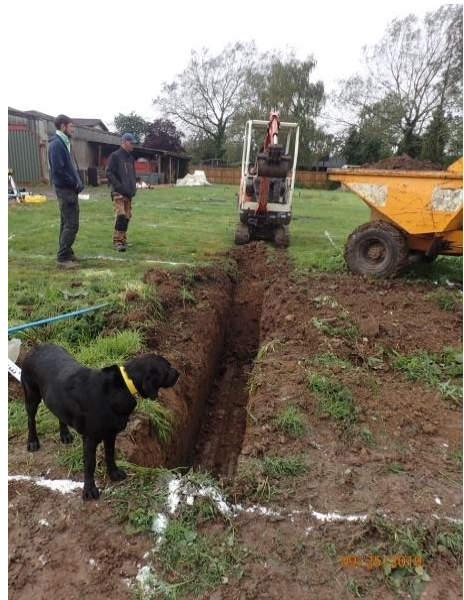
Plate 61: Excavation of the foundations, from the east
