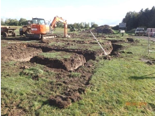
Plate 102: Excavation of the foundations, from the west
