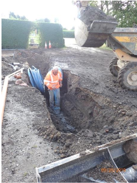
Plate 48: Excavation of the third section of service trench, from the north
