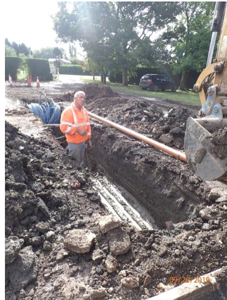
Plate 128: Excavation of the third section of service trench, from the north
