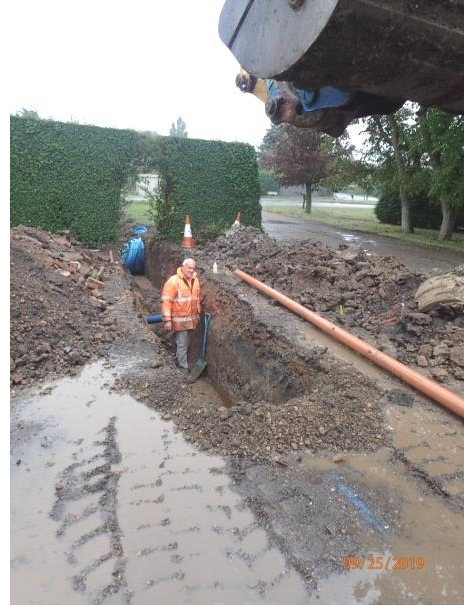
Plate 42: Excavation of the third section of service trench, from the north
