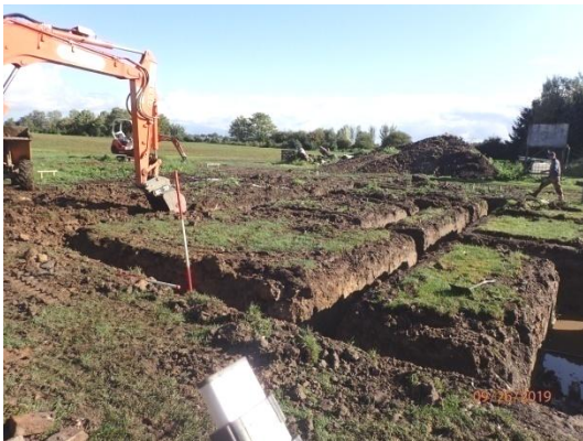
Plate 103: Excavation of the foundations, from the west
