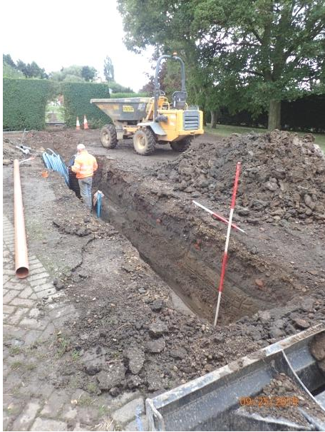
Plate 52: Excavation of the third section of service trench, from the north
