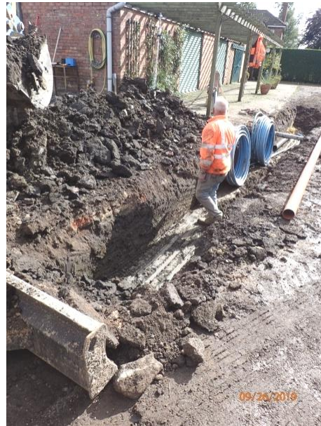
Plate 132: Excavation of the third section of service trench, from the north
