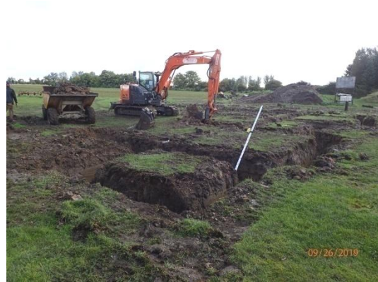
Plate 99: Excavation of the foundations, from the west
