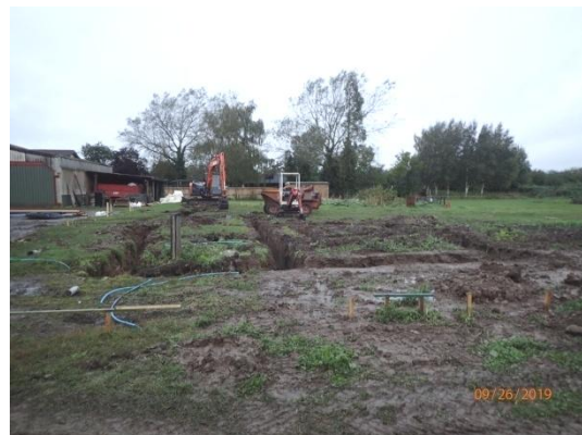
Plate 89: Excavation of the foundations, from the east
