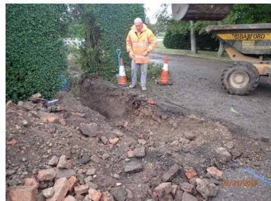
Plate 35: Excavation of the third section of service trench, from the north
