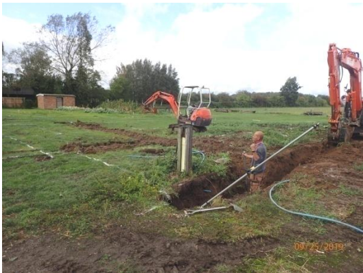
Plate 67: Excavation of the foundations, from the south-east
