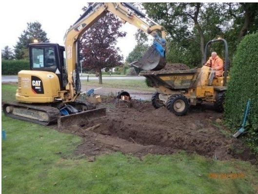
Plate 23: Re-excavation of the first section of service trench, from the east
