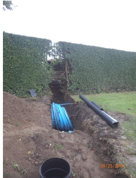
Plate 29: Excavation of the second section of service trench through the hedgerow, from the south
