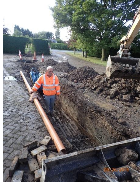
Plate 119: Excavation of the third section of service trench, from the north
