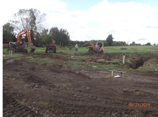
Plate 87: Excavation of the foundations, from the south-east
