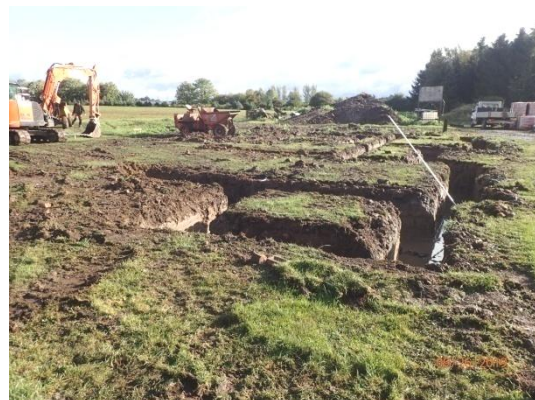
Plate 101: Excavation of the foundations, from the west
