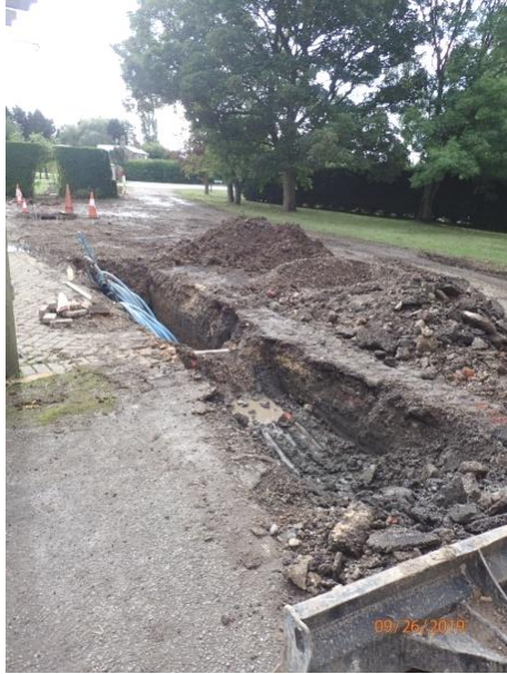
Plate 125: Excavation of the third section of service trench, from the north
