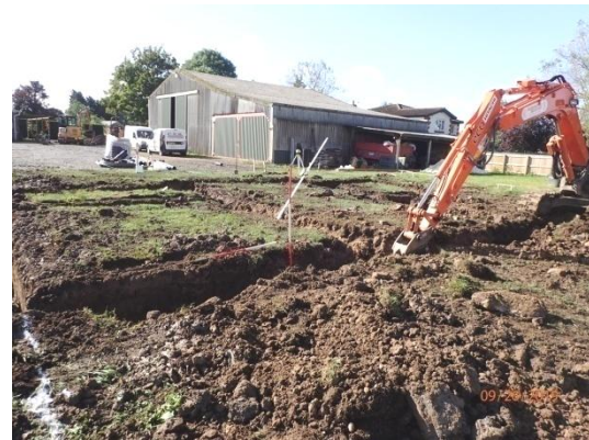
Plate 107: Excavation of the foundations, from the north-east
