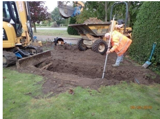
Plate 25: Re-excavation of the first section of service trench, from the east
