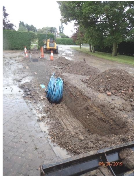
Plate 116: Excavation of the third section of service trench, from the north
