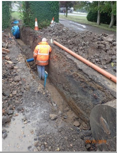
Plate 43: Excavation of the third section of service trench, from the north
