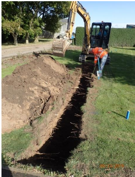
Plate 14: Excavation of the first section of service trenching, from the south
