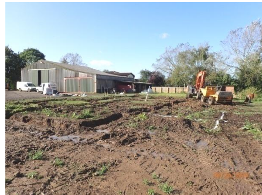
Plate 106: Excavation of the foundations, from the east
