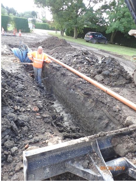
Plate 129: Excavation of the third section of service trench, from the north
