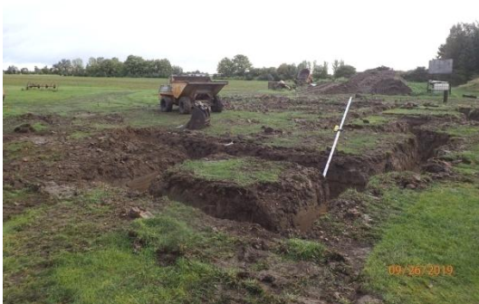
Plate 98: Excavation of the foundations, from the west
