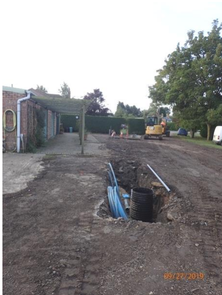
Plate 134: Excavation of the third section of service trench, from the north
