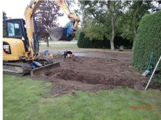
Plate 24: Re-excavation of the first section of service trench, from the east
