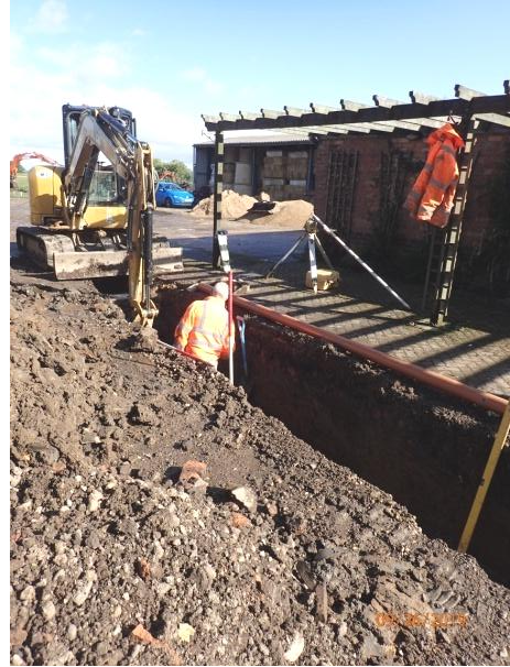
Plate 123: Excavation of the third section of service trench, from the north
