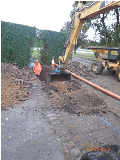
Plate 37: Excavation of the third section of service trench, from the north
