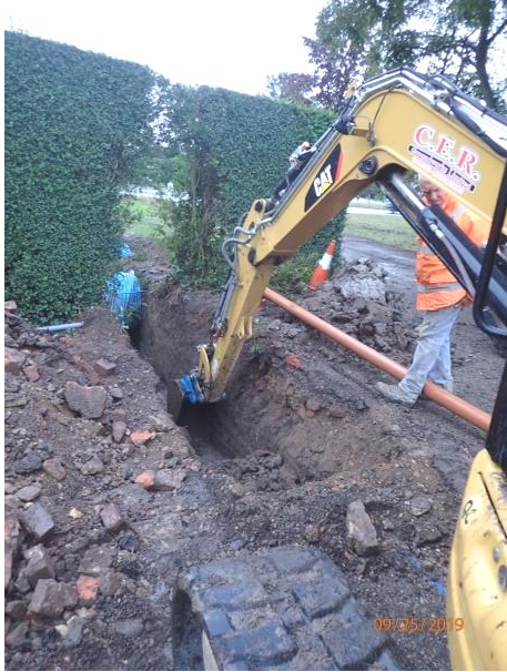
Plate 36: Excavation of the third section of service trench, from the north
