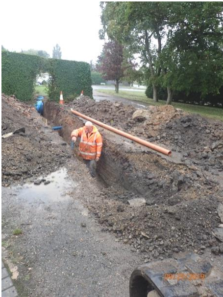
Plate 45: Excavation of the third section of service trench, from the north
