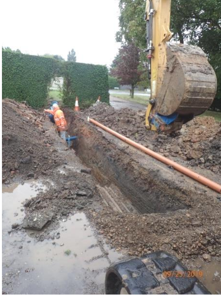
Plate 44: Excavation of the third section of service trench, from the north
