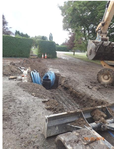
Plate 47: Excavation of the third section of service trench, from the north
