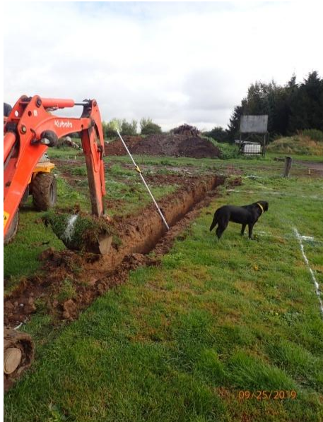
Plate 63: Excavation of the foundations, from the west
