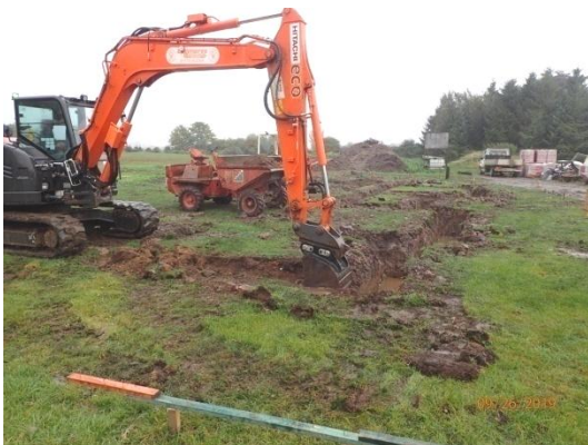
Plate 92: Excavation of the foundations, from the west
