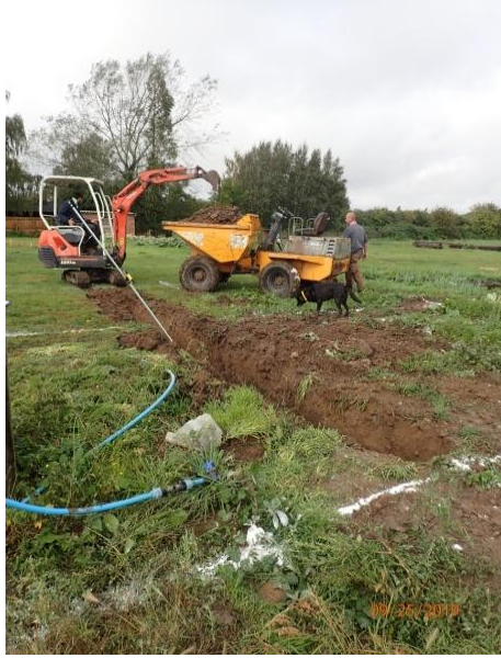
Plate 62: Excavation of the foundations, from the east
