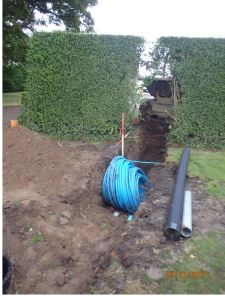
Plate 31: Excavation of the second section of service trench through the hedgerow, from the south
