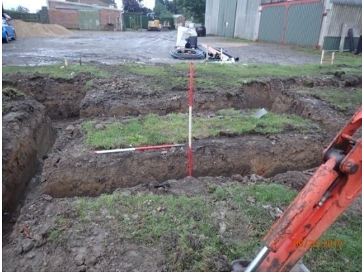
Plate 90: Excavation of the foundations, from the north
