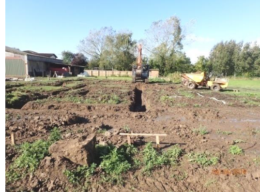
Plate 105: Excavation of the foundations, from the east
