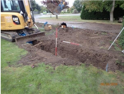
Plate 27: Re-excavation of the first section of service trench, from the east
