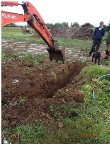
Plate 58: Excavation of the foundations, from the west
