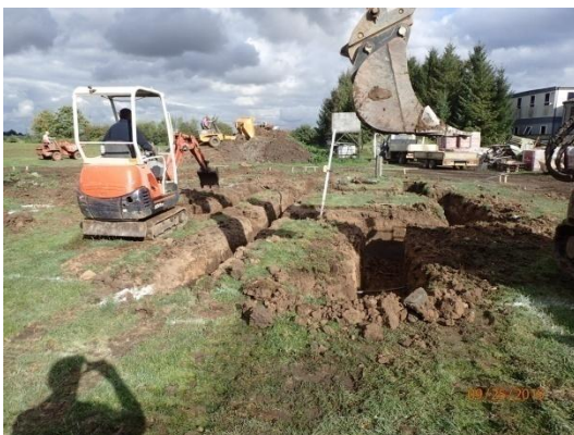
Plate 86: Excavation of the foundations, from the west
