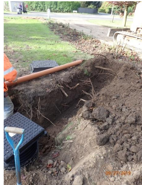
Plate 136: Excavation of the fourth section of service trench, from the north
