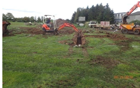
Plate 81: Excavation of the foundations, from the west
