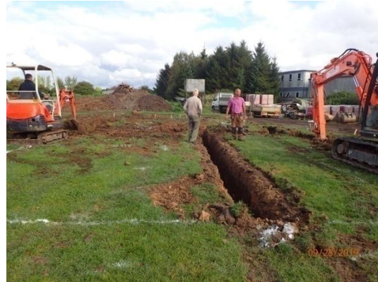
Plate 75: Excavation of the foundations, from the west
