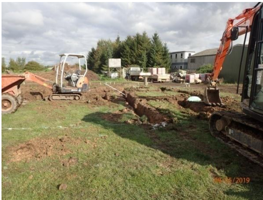
Plate 85: Excavation of the foundations, from the west
