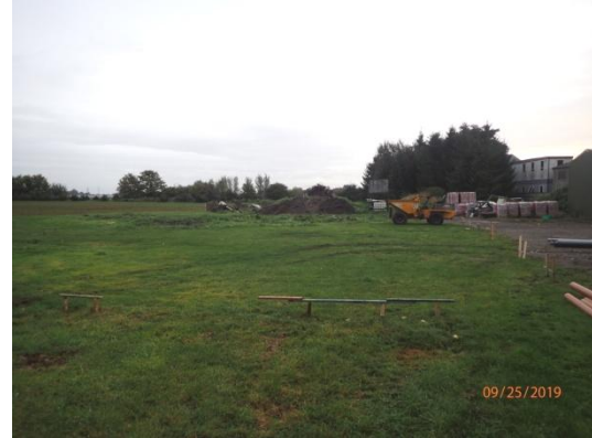
Plate 54: Pre-groundworks, from the west
