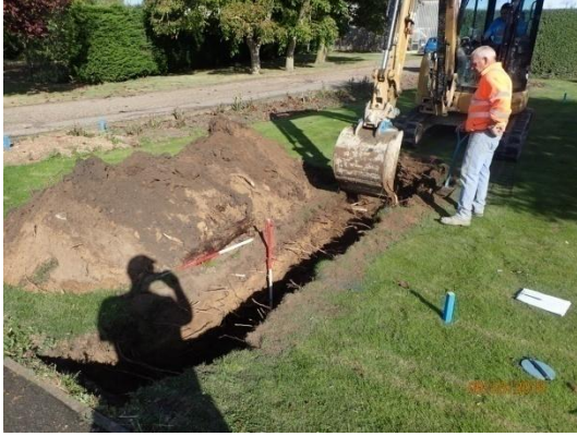
Plate 12: Excavation of the first section of service trenching, from the south
