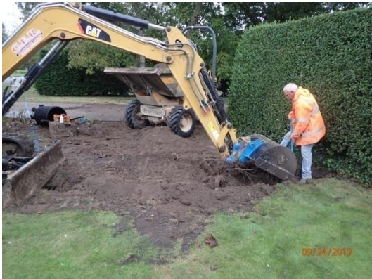
Plate 22: Re-excavation of the first section of service trench, from the east
