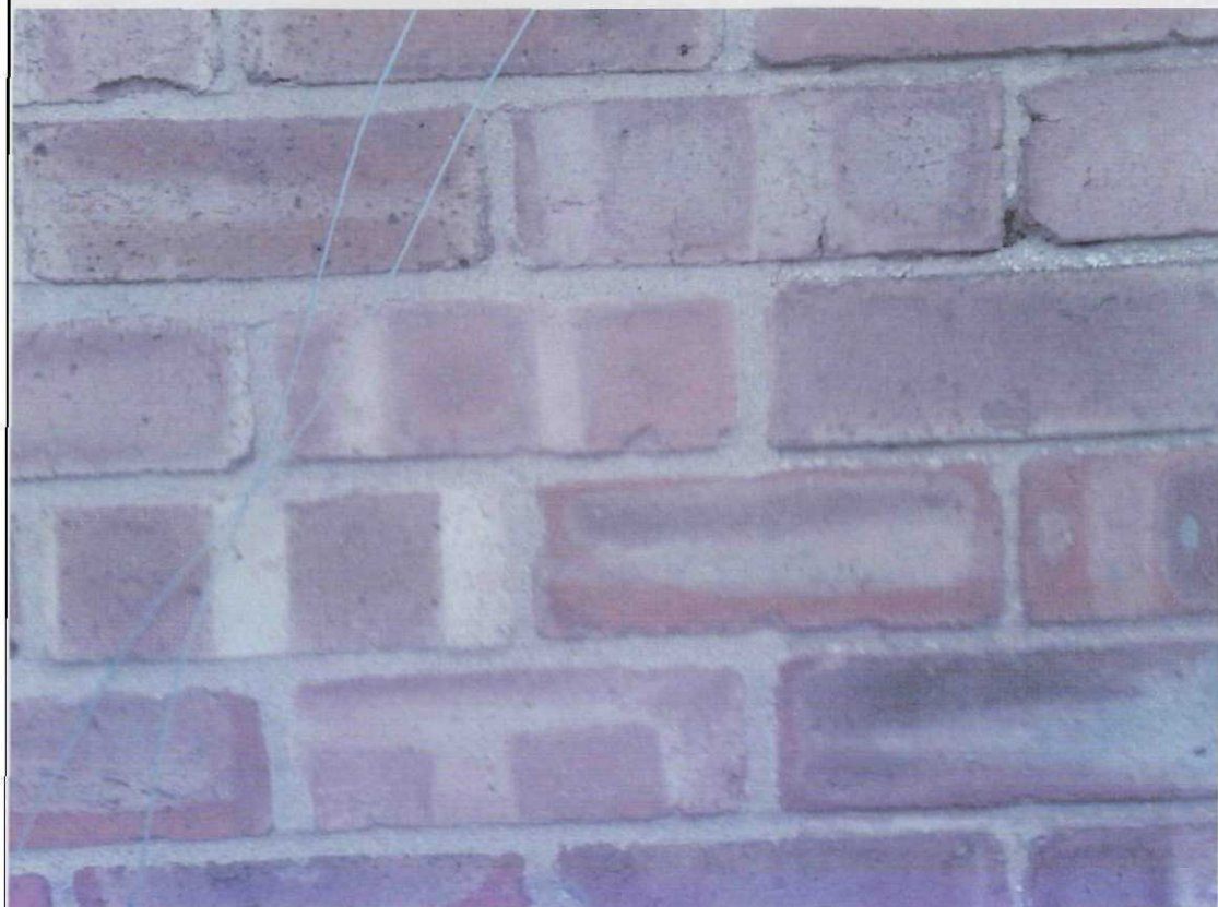
SAMPLE OF THE EXISTING BRICK WORK
