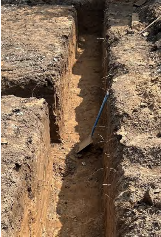
Foundation excavation
