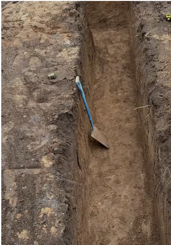
Foundation excavations
