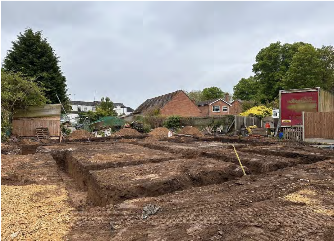
Building footprint after excavation of foundation trenches
