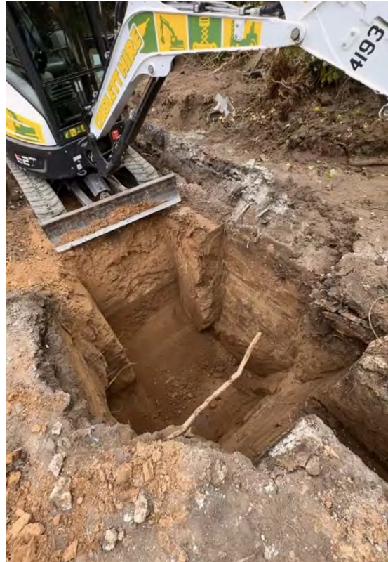
Septic tank excavation
