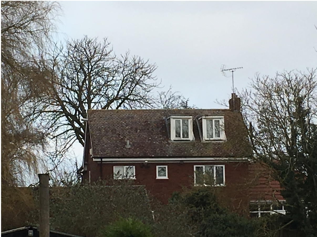
Figure 8: Dwelling to the rear of the site
