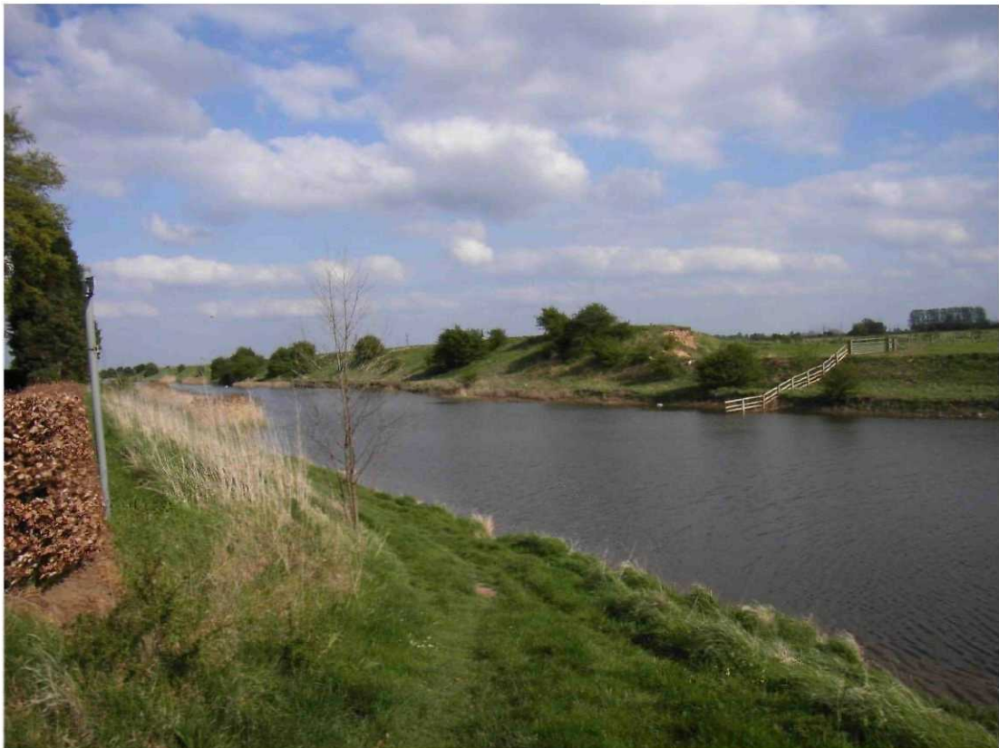
Facing south east along the North Level West Drain.
