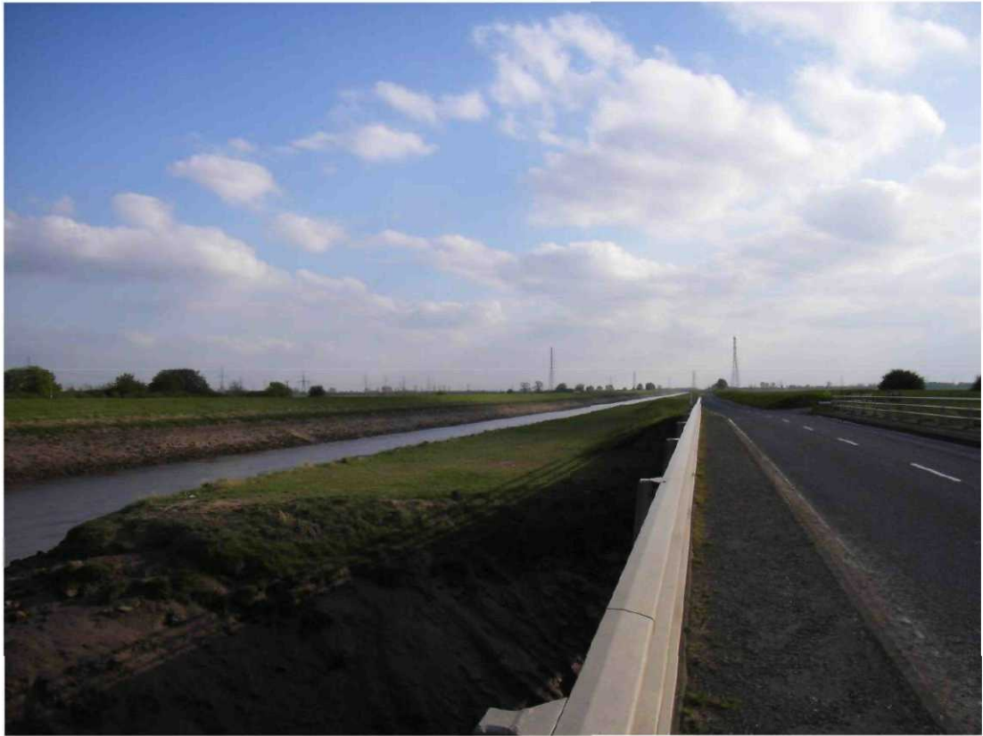
River Nene from the road bridge at the confluence with South Holland Main Drain. Facing south.
