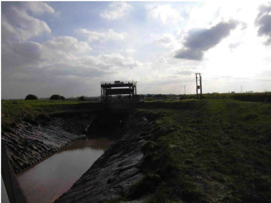
Sluice gate on the South Holland Main Drain before the confluence with Nene Outfall Cut. Facing south west.
