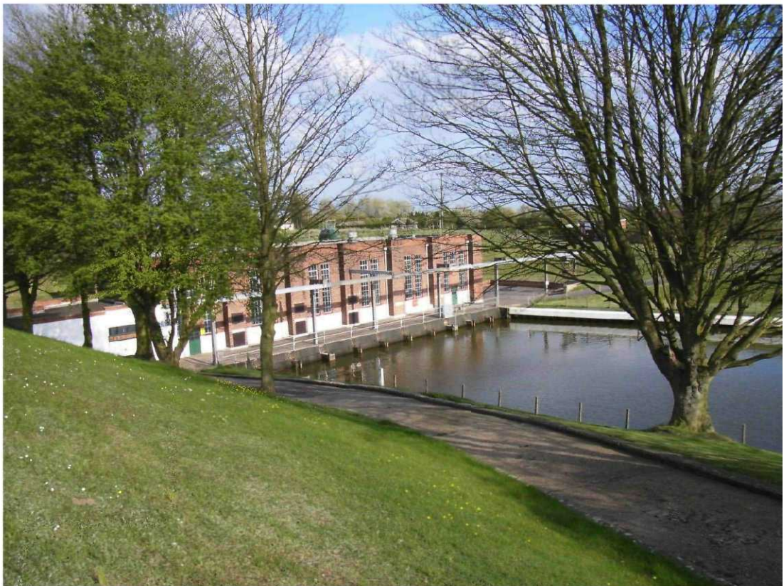
Photograph of the North Level IDB pumping station and the sluice complex. Facing south east.
