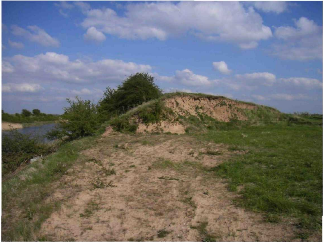
Facing East along the South Level Main Drain, the photo shows the cross section of the flood defence bunds.
