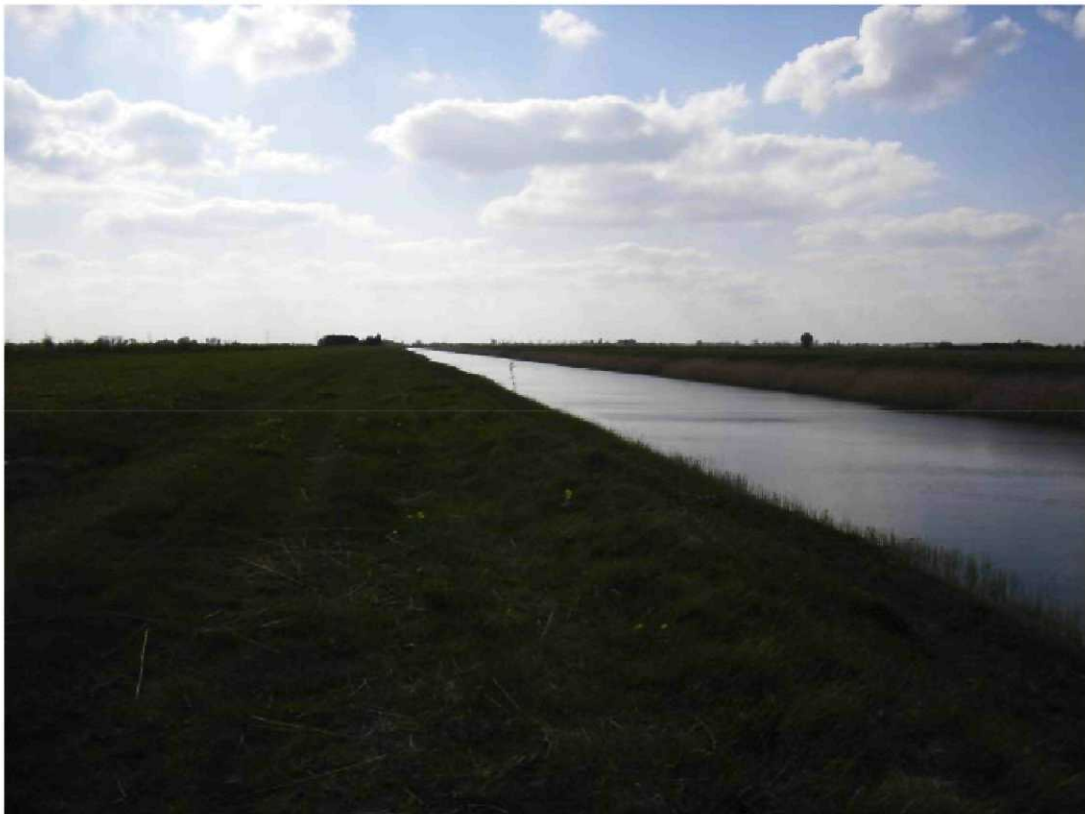
Facing west along the South Level Main Drain.
