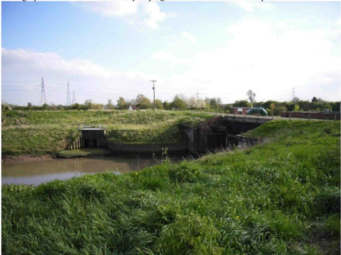
Photograph of the North Level IDB pumping station and the sluice complex. Facing south west.
