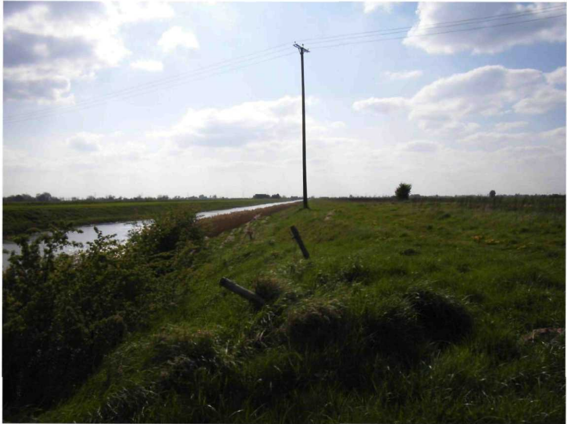
Facing west, along the North Level West Drain.
