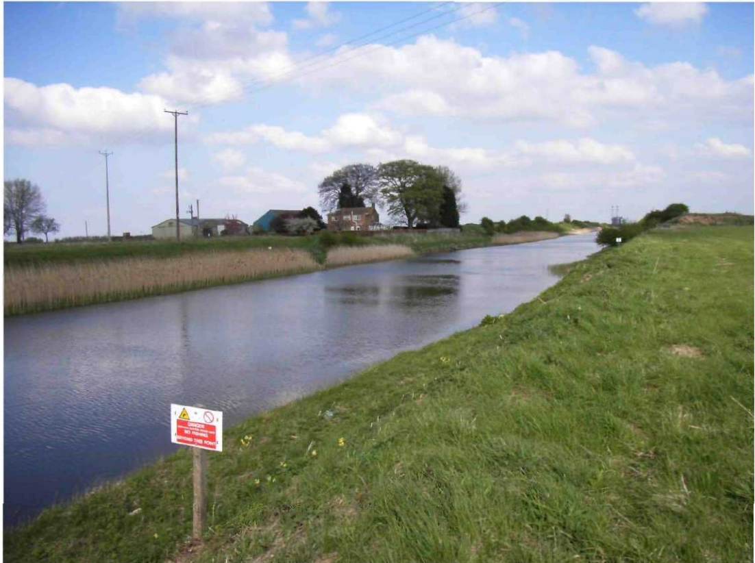
Facing east, view of the South Level Main Drain to the north west of the site where bunds are absent.
