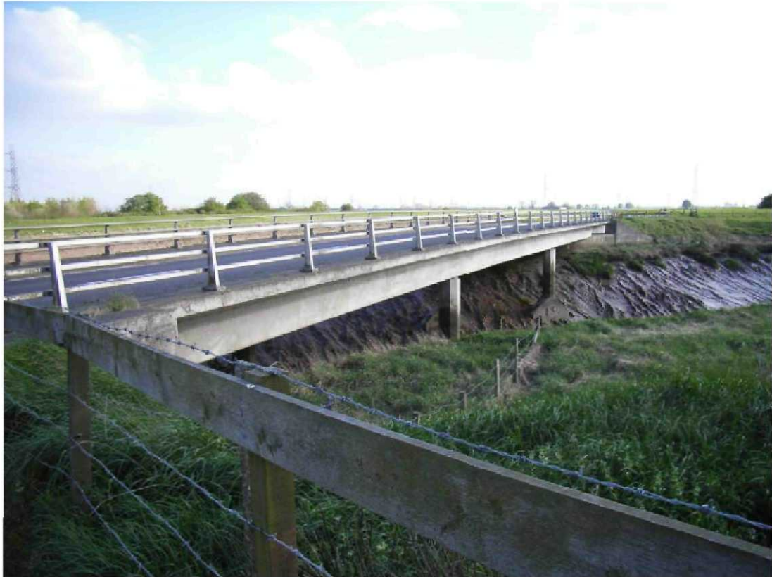
Road bridge over the South Level Main Drain confluence with the Nene Outfall.
