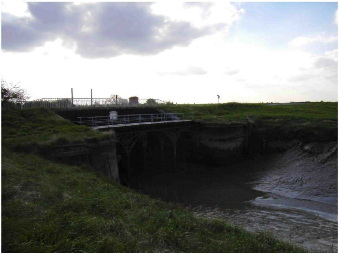
Sluice gates at the confluence of the River Nene and North Level West Drain. Facing south west.
