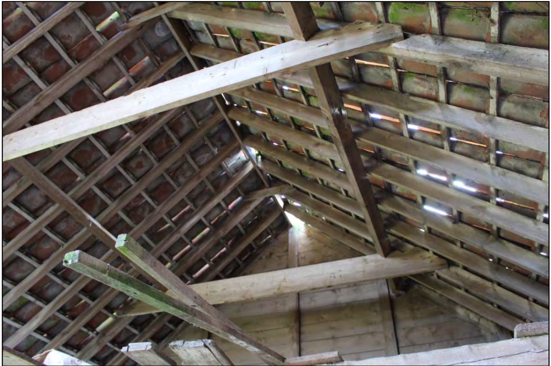
Photo 33: Overview of roof structure within Building E, note the underside of the clay pantiles above
