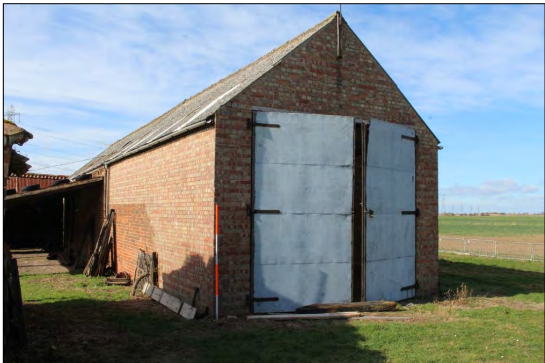
Photo 1: Overview of Building A, viewed from the south-east
