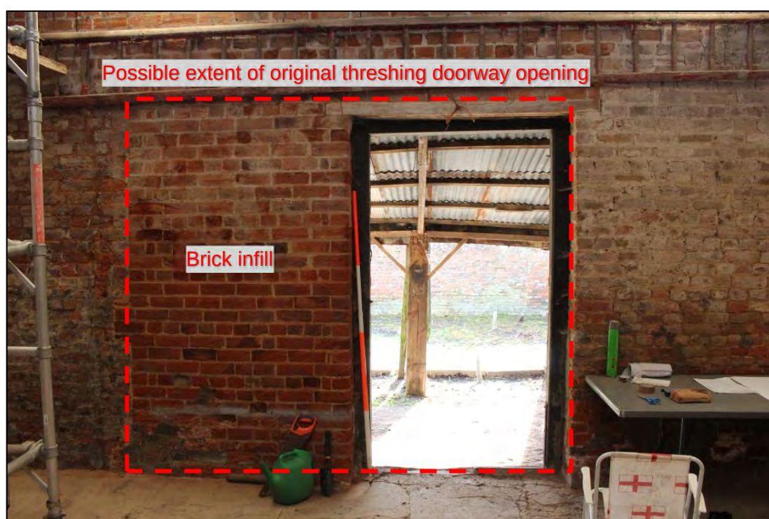
Photo 13: Overview of single doorway within the southern elevation, note the renewed brickwork to the north of the door
