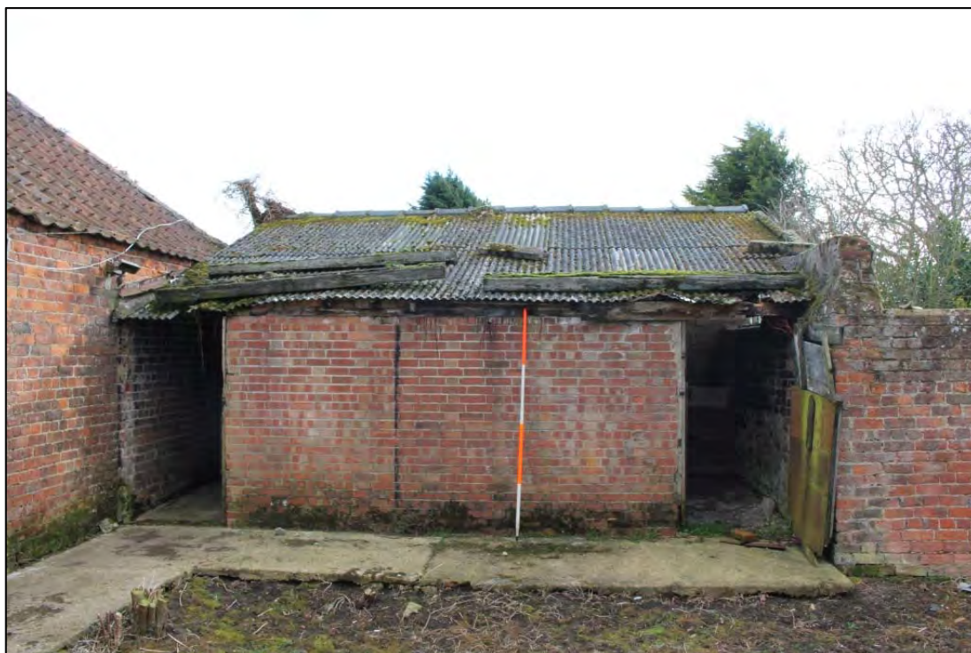
Photo 27: Overview of Building D, looking south
