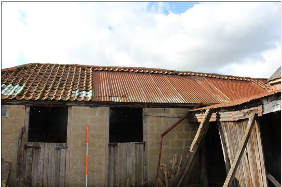
Photo 18: Overview of eastern elevation of Buildings B and C
