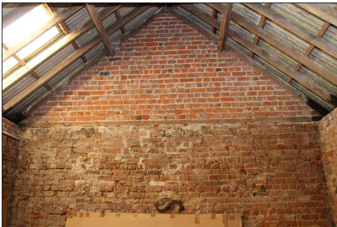
Photo 14: Overview of western gable of the barn, note the change in brickwork and the incorporation of a horizontal roof timber
