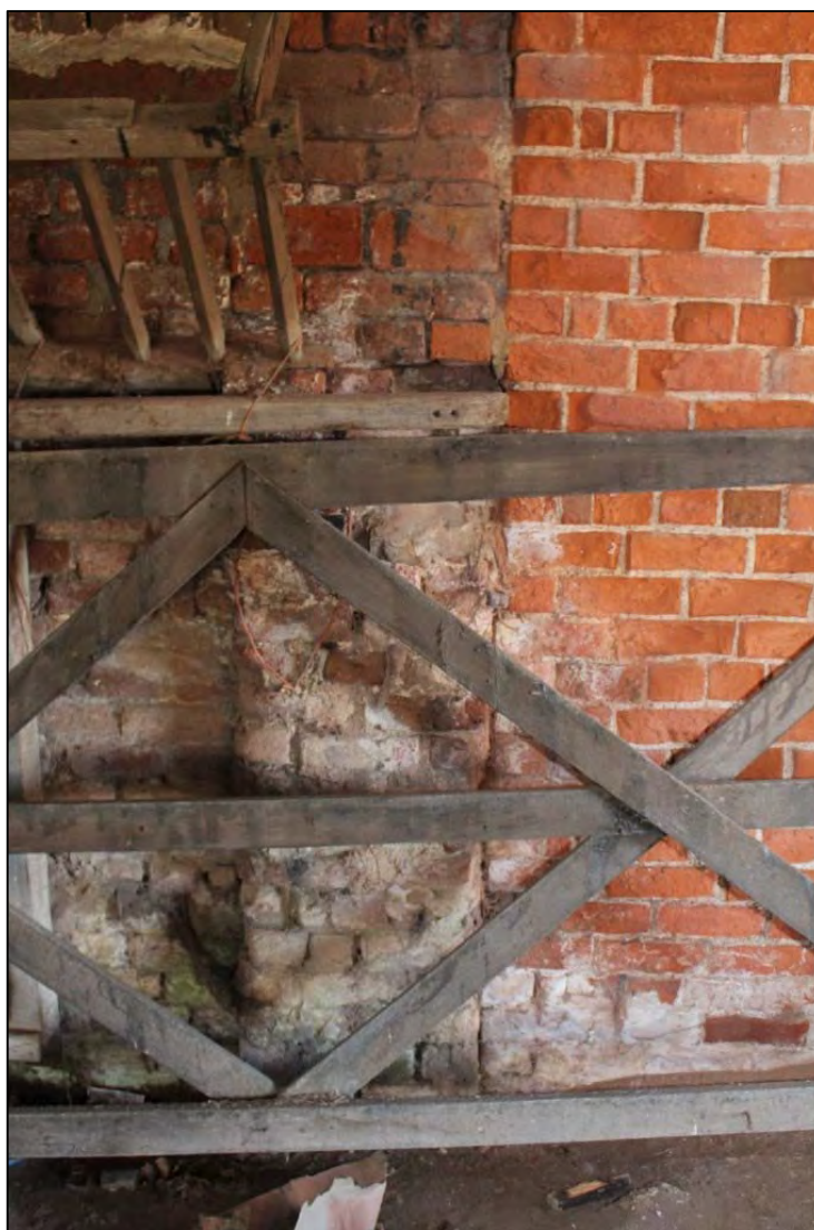
Photo 20: Detail of butt joint within western elevation of Building B. Note the tapering of the buttress as it rises
