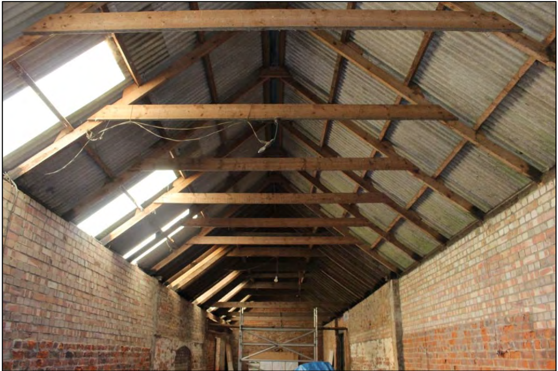
Photo 15: Overview of roof structure, looking west
