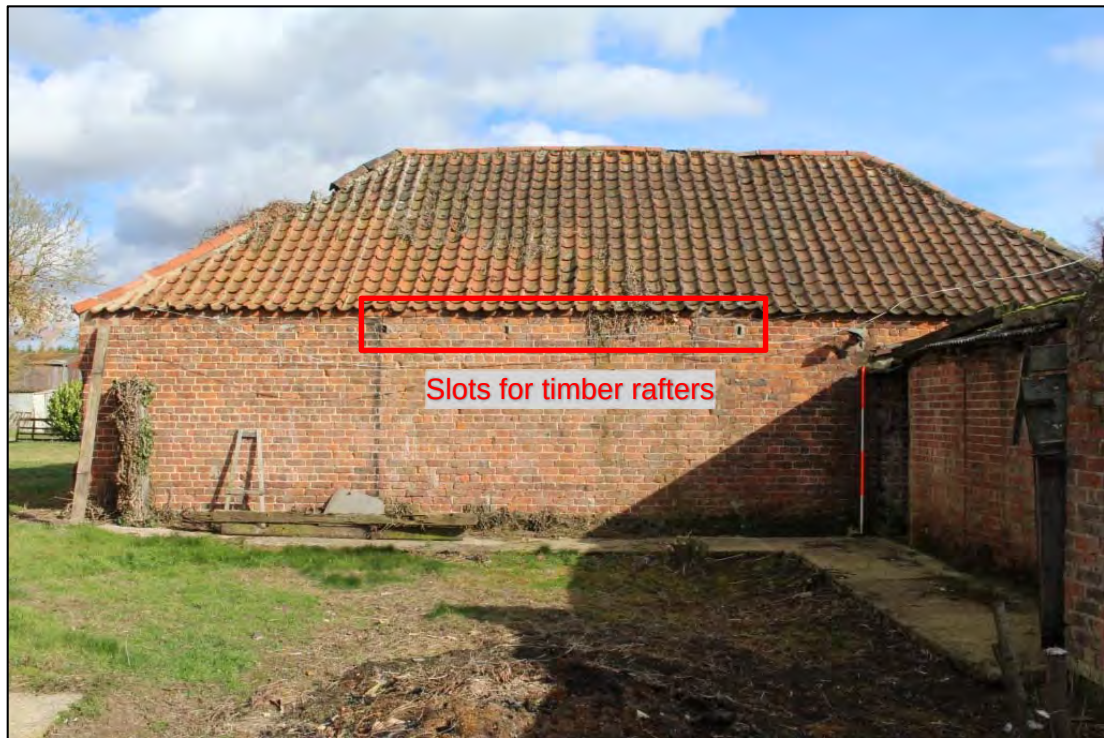
Photo 36: Overview of western elevation of Building E
