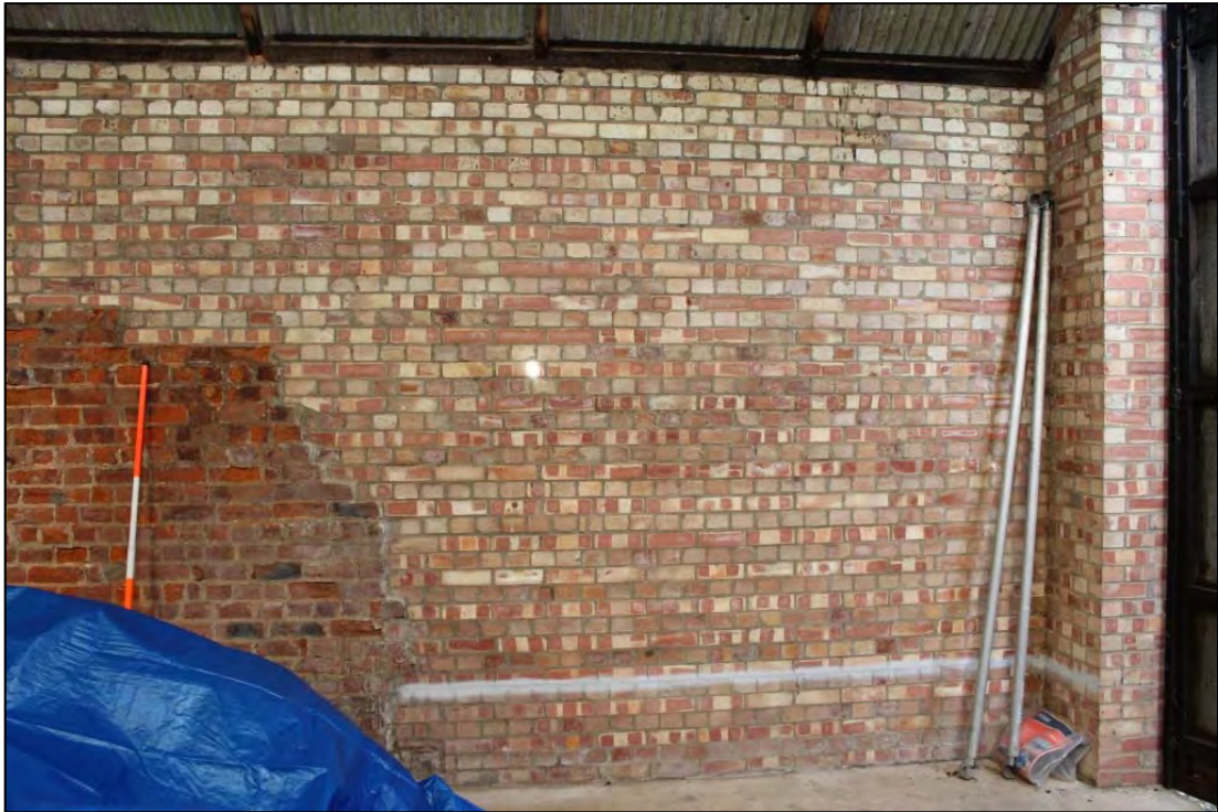
Photo 3: Internal view of north-eastern extent of Building A, showing 20th-century repair and extension works
