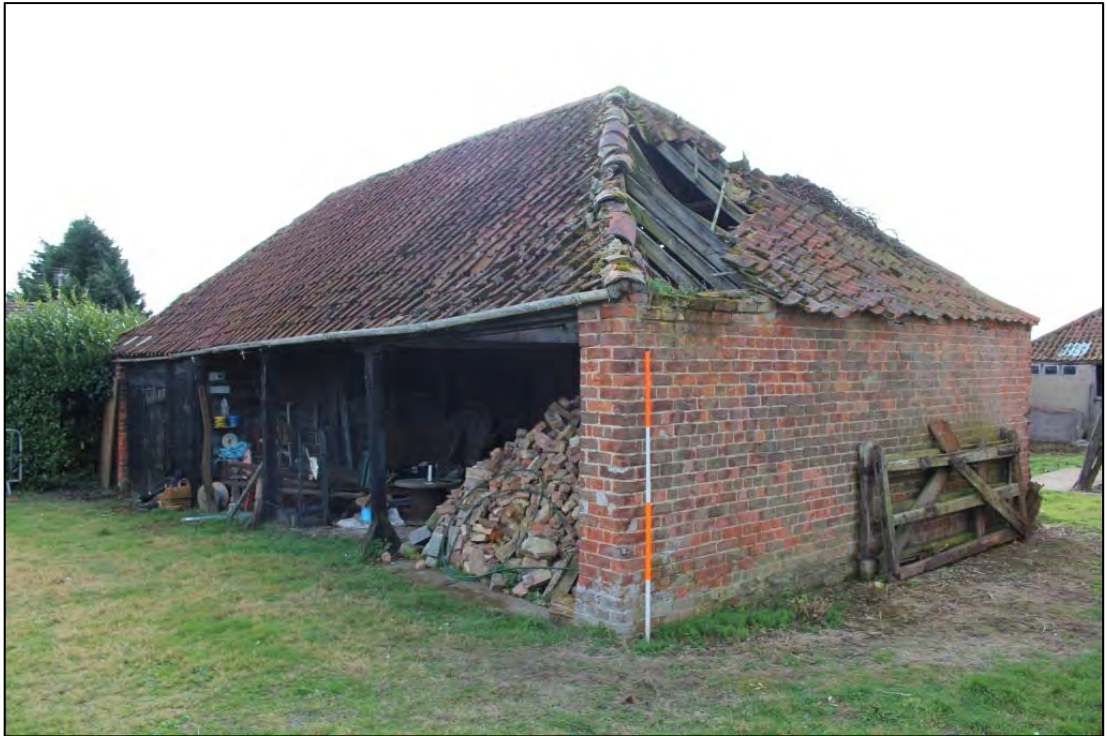
Photo 30: Overview of Buildings E & F, looking south-west
