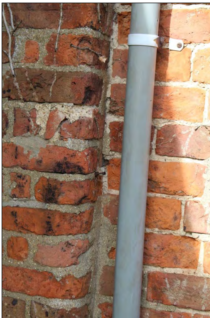
Photo 5: Detail of butt joint within southern elevation. Note the rounded bricks to the western side of the joint
