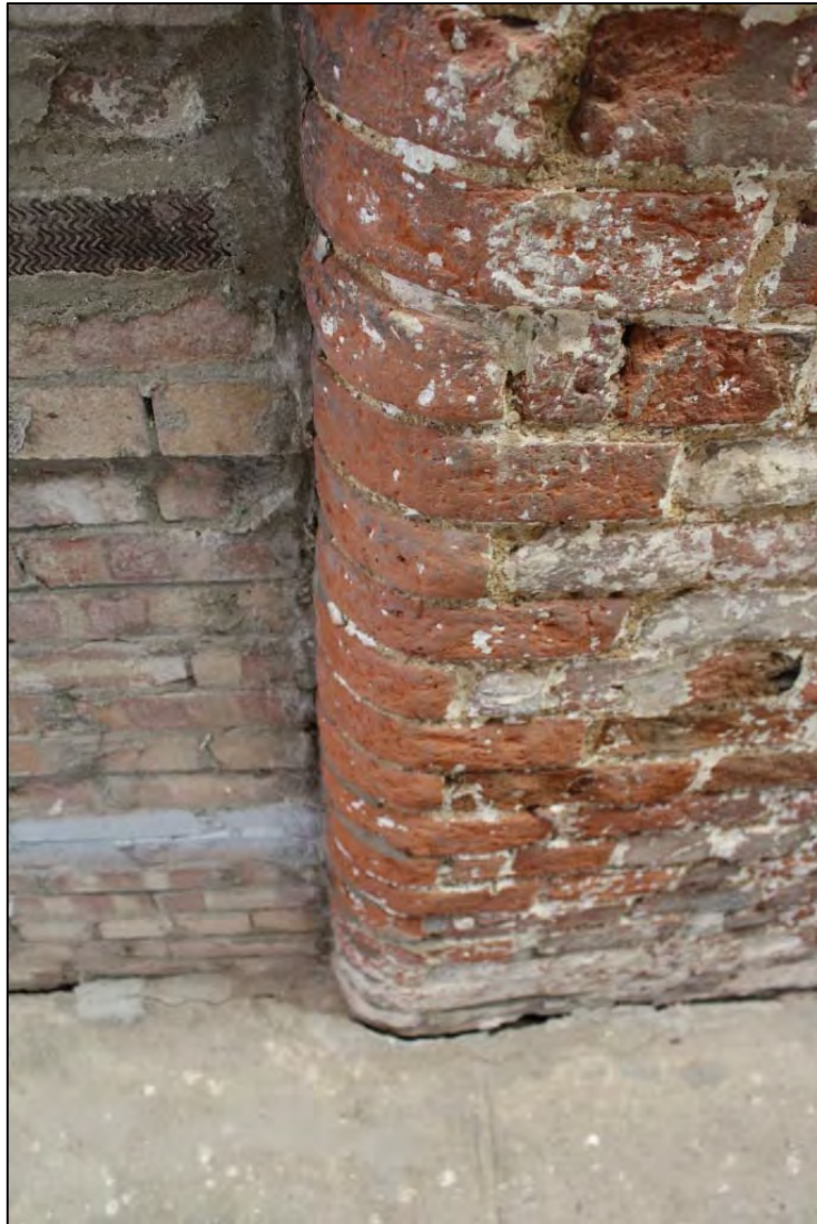
Photo 8: Detail of bullnose bricks to the blocked-up opening
