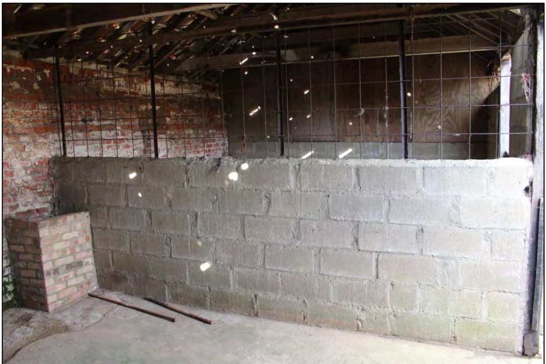
Photo 23: Overview of Building C, looking north
