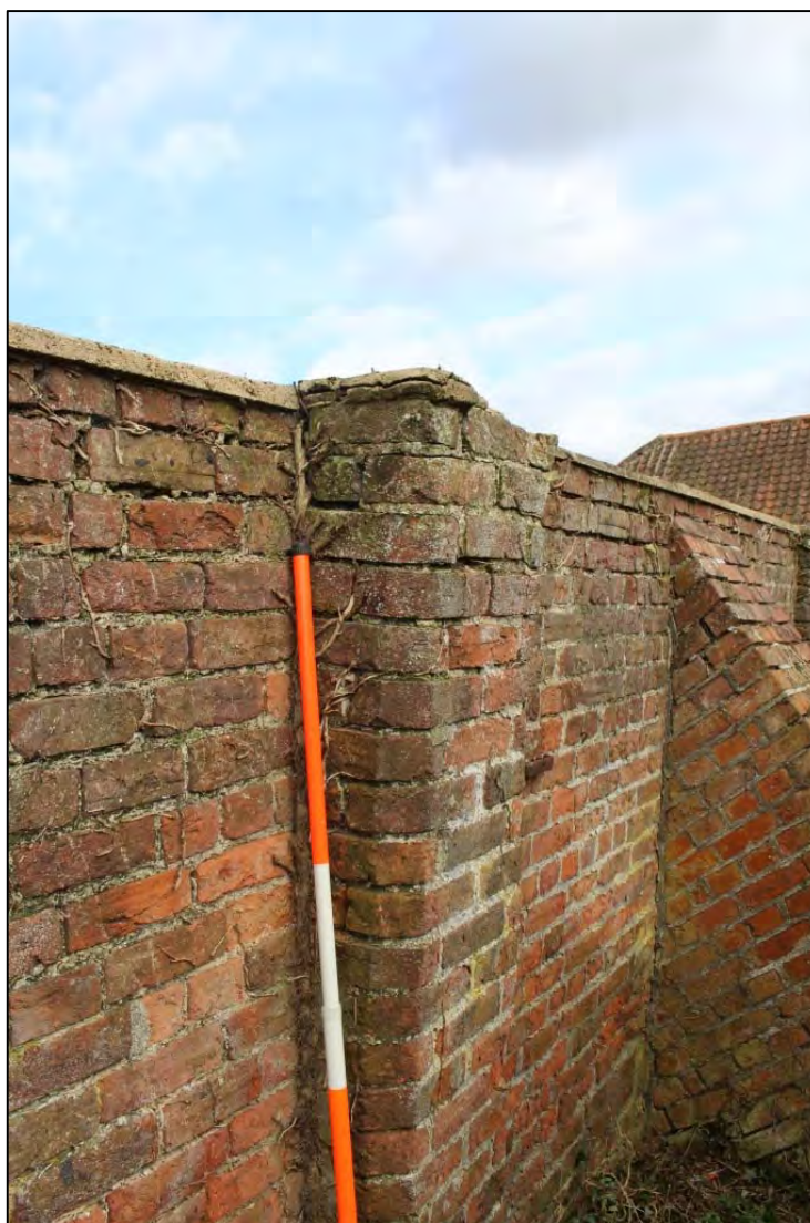
Photo 41: Detail of buttress within southern wall
