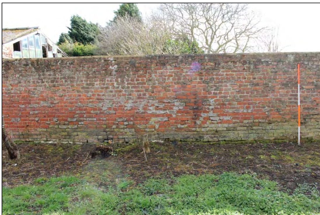
Photo 38: Overview of southern wall, looking south
