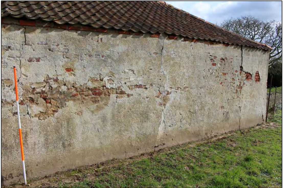
Photo 25: Overview of the southern extent of the western elevation
