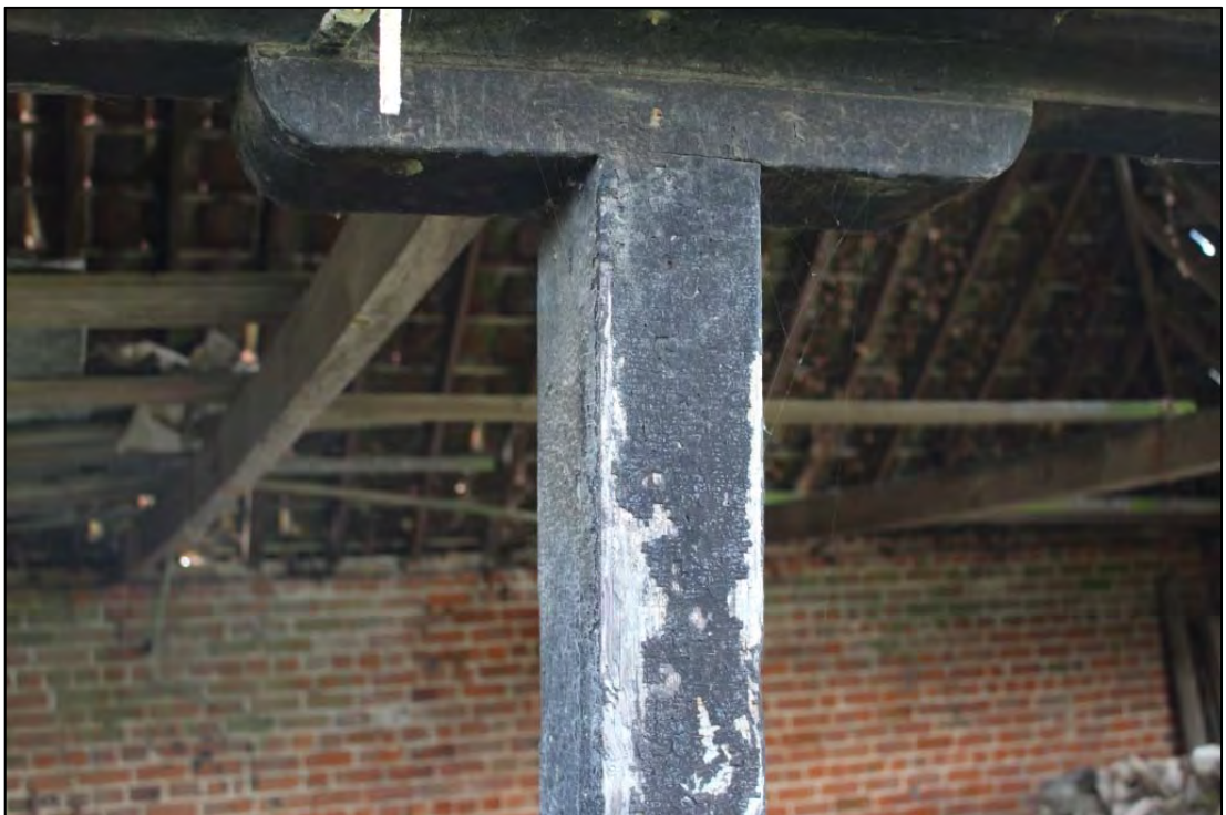
Photo 31: Post and pad arrangement to the open side of Building E
