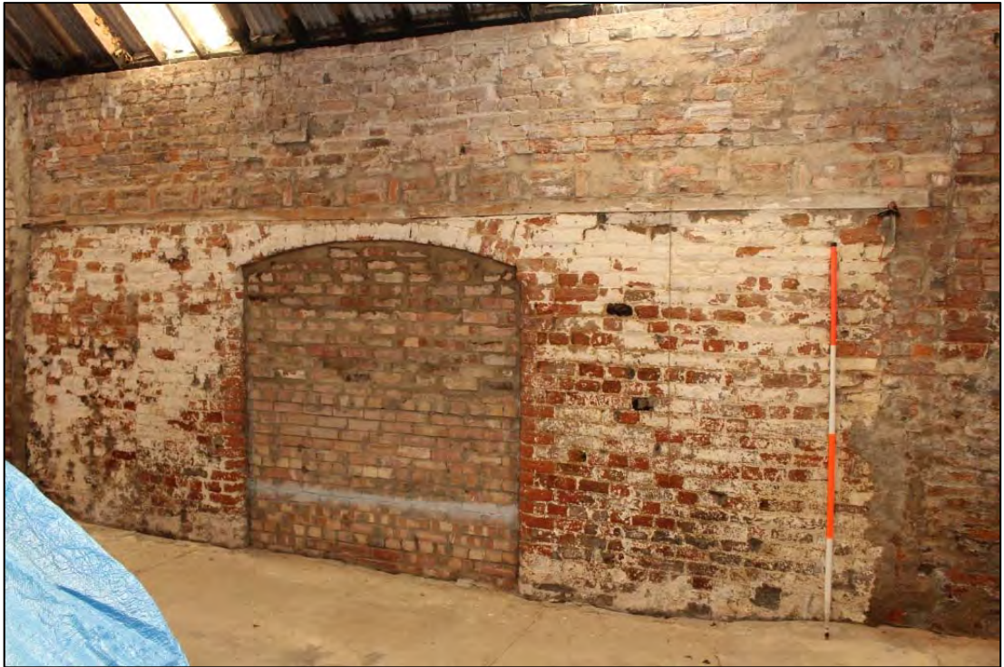
Photo 9: Internal view of southern elevation incorporating segmental arch opening and possible slots for first floor joists
