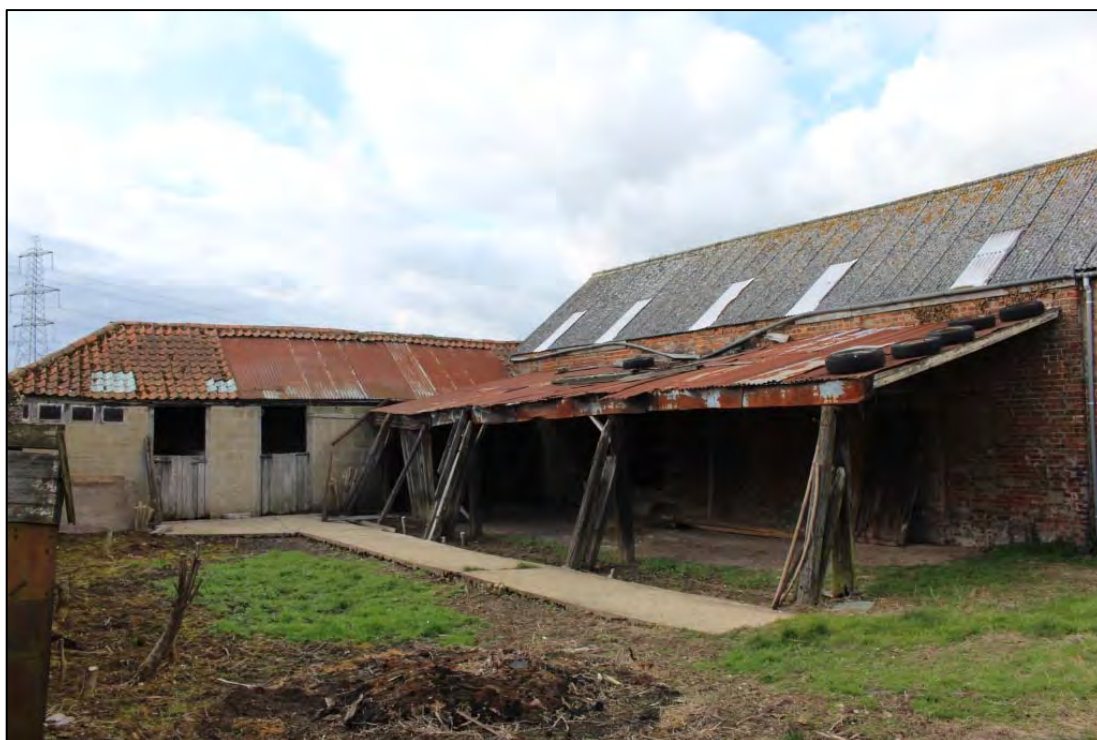
Photo 37: Overview of Building G, looking north-west
