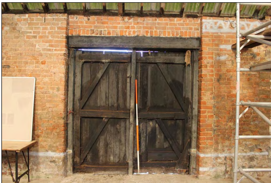
Photo 12: Overview of double timber doors within the northern elevation
