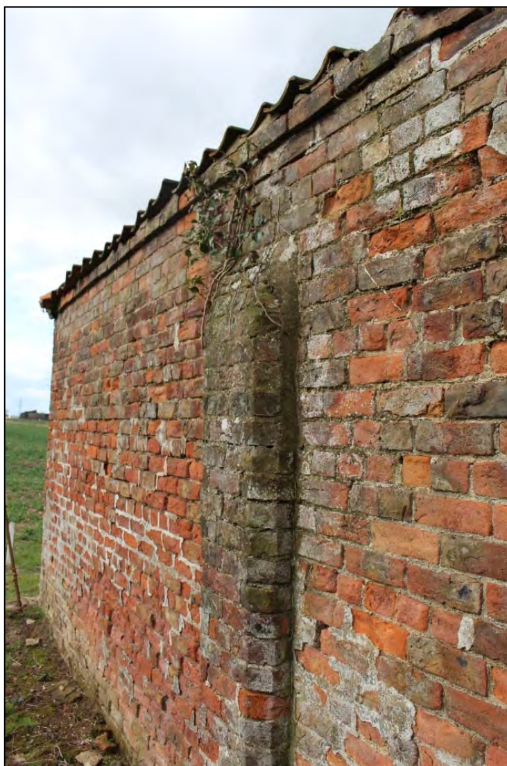
Photo 40: Detail of westernmost buttress to the southern elevation of Building C, note the decorative chamfering and taper
