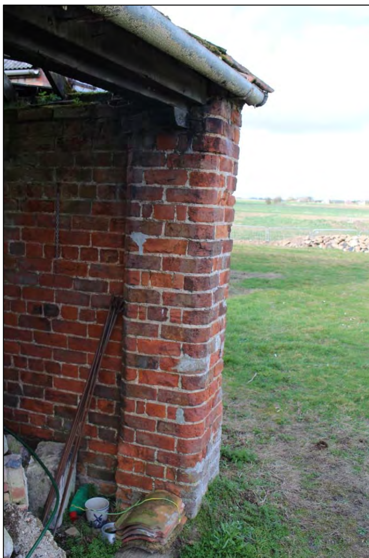
Photo 32: Chamfered brickwork to the northern extent of the eastern elevation
