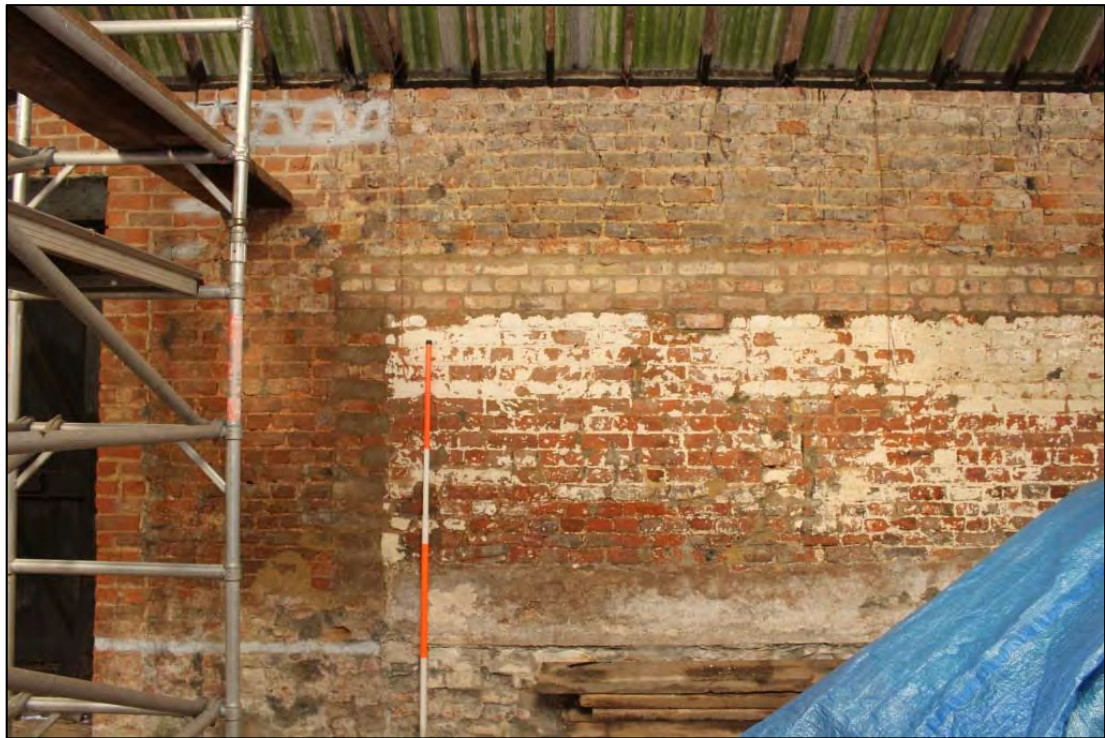
Photo 11: Detail of northern elevation showing evidence of alterations
