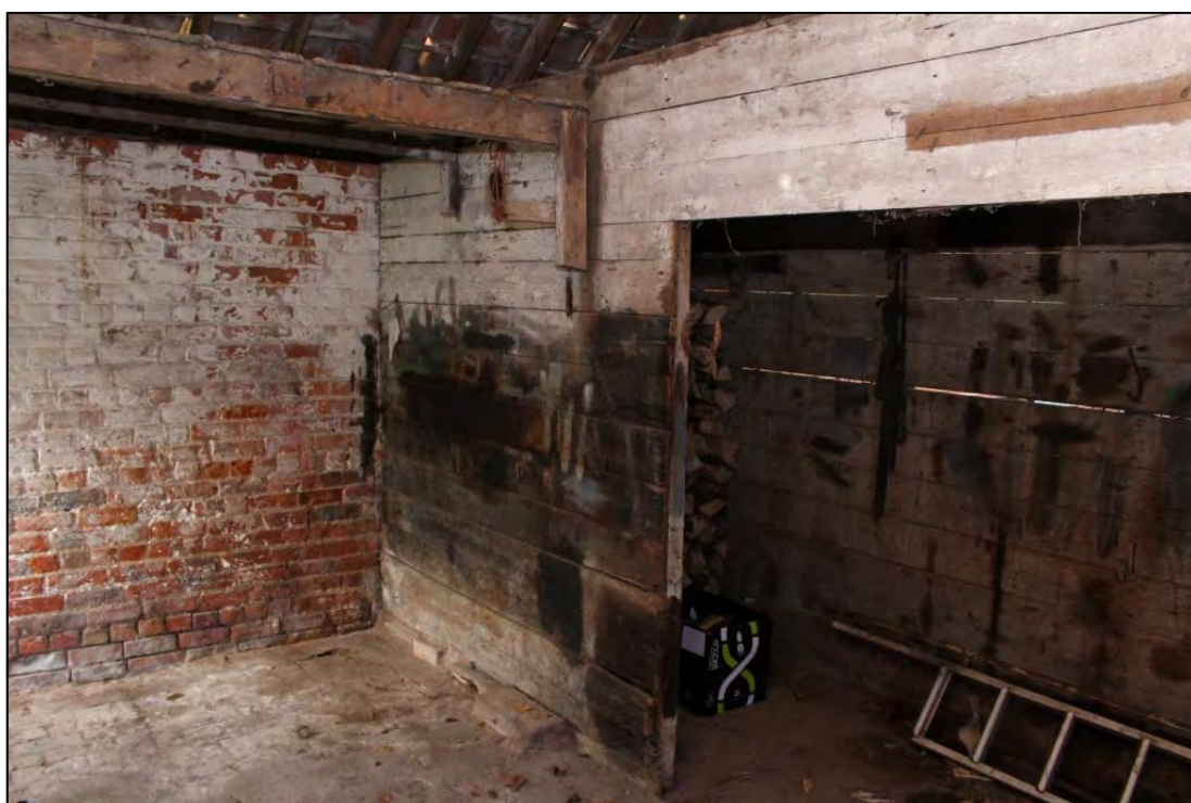
Photo 35: Remnants of workshop within Building F, the timber partitioning separates the building from Building E
