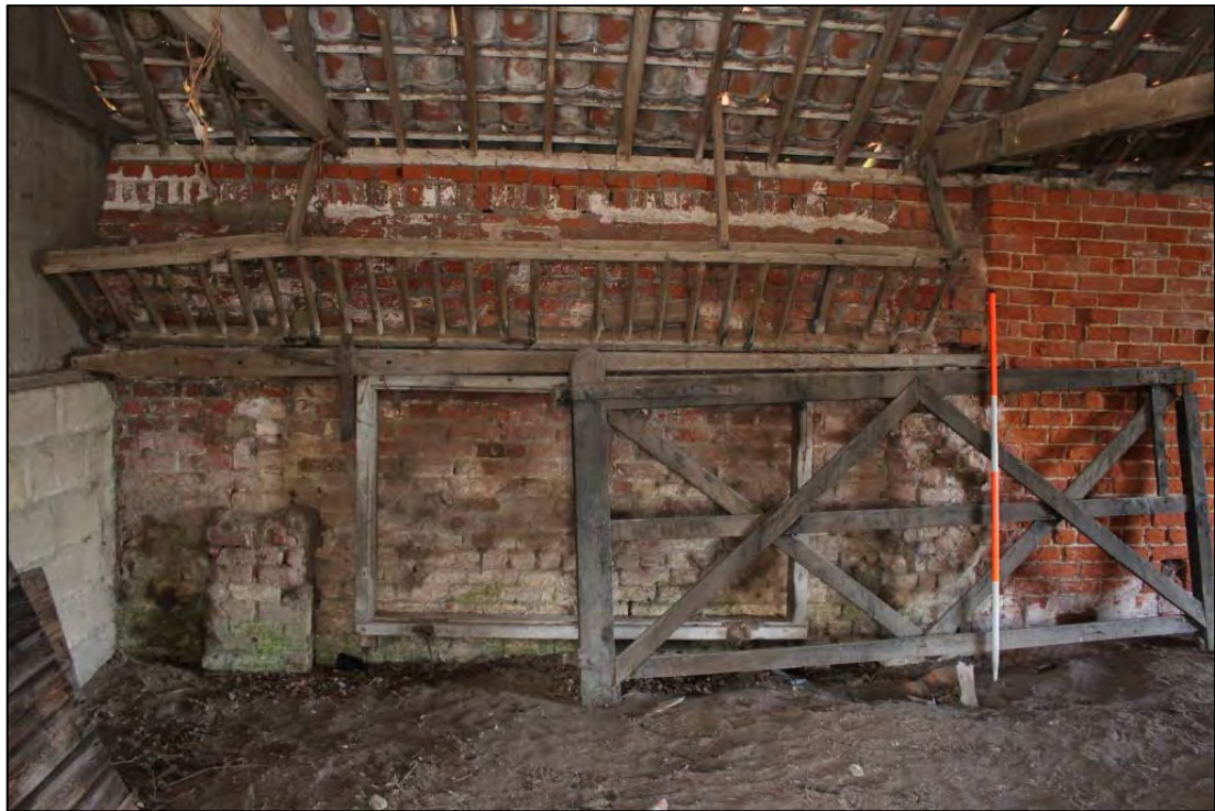
Photo 21: Overview of southern extent of western elevation within Building B
