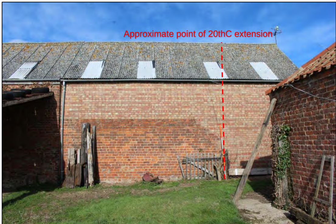
Photo 2: Overview of north-eastern extent of Building A
