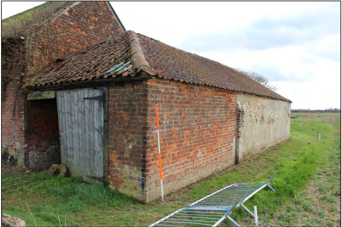
Photo 17: Overview of Building B, looking south-east
