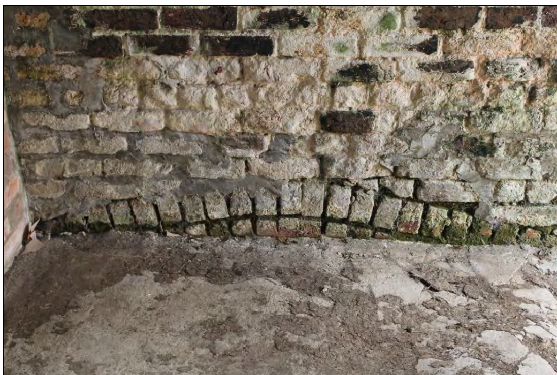
Photo 29: Brick segmental arch within Building D, also visible externally
