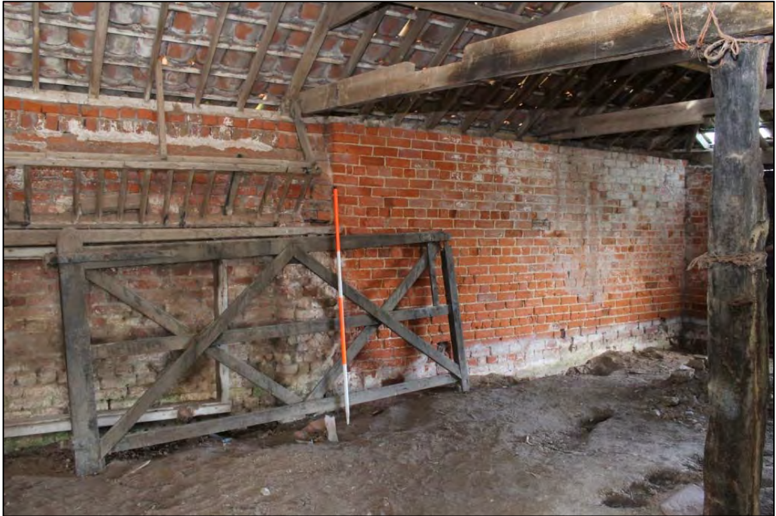
Photo 19: Overview of western elevation within Building B
