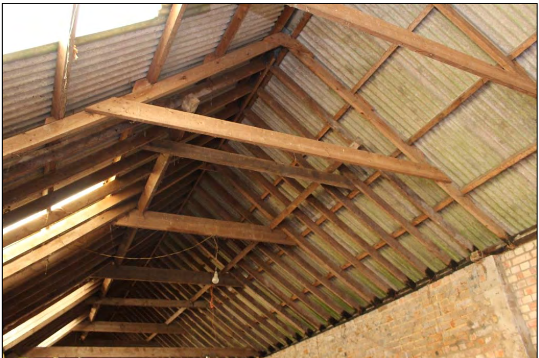
Photo 16: Width and placement of collars changes at the point of the earlier extension, also note the change in rafter spacing and termination of clasped purlins. The butt joint within the northern elevation can be seen in the lower right of the picture
