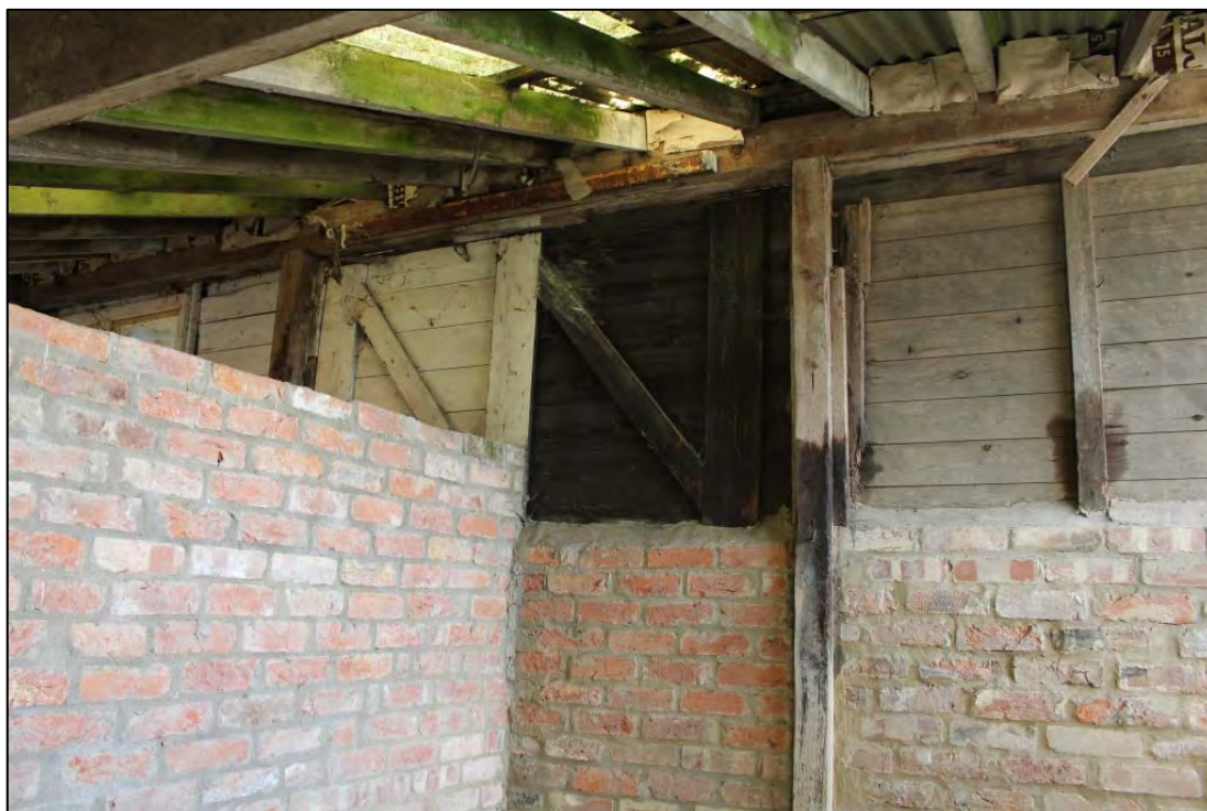
Photo 28: Overview of internal southern elevation
