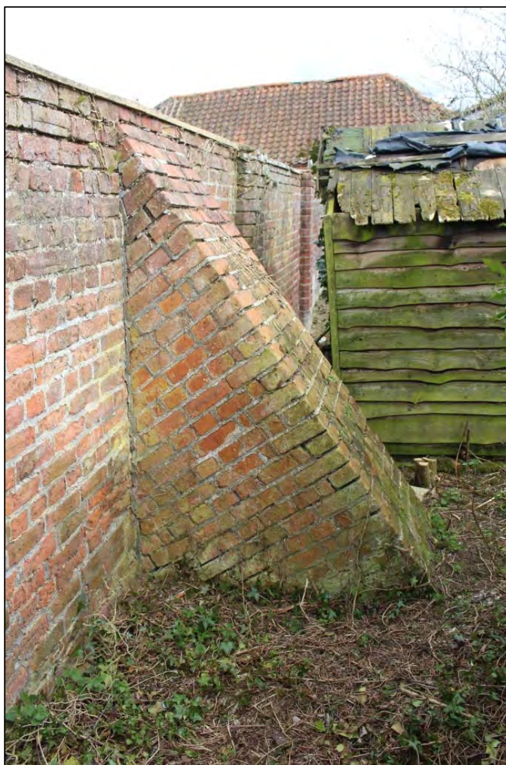
Photo 42: Angled buttress supporting southern wall
