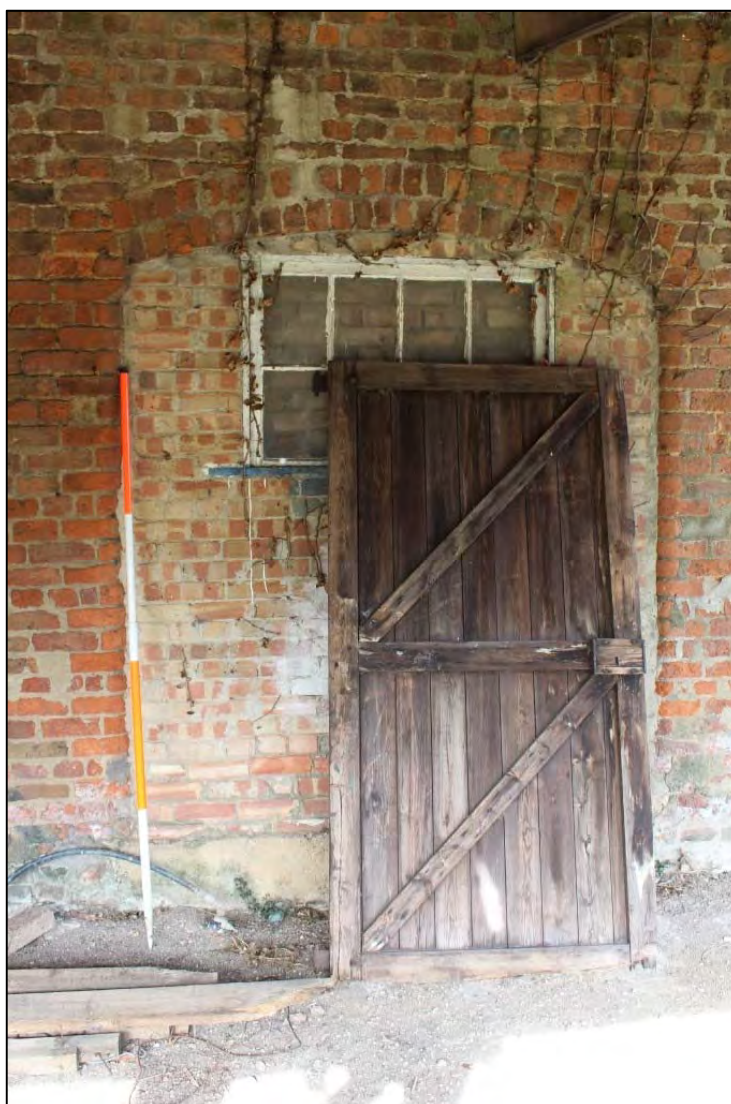
Photo 7: Overview of blocked up arch-headed opening within the southern elevation
