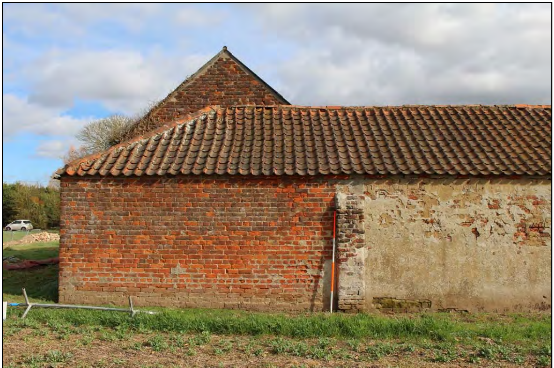
Photo 24: Overview of western elevation of Building B
