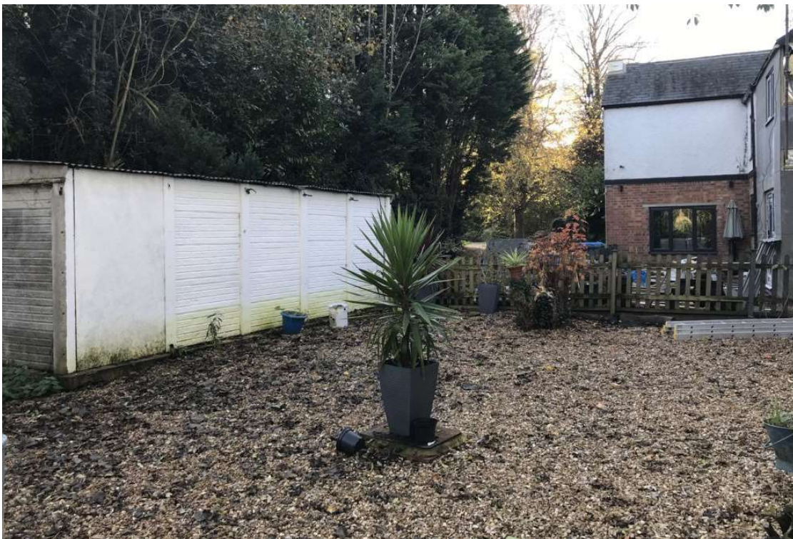
Figure 3. Photo of the old garage structure which would be demolished as part of the proposal .
