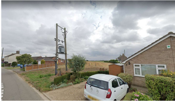
View into site from Broadgate South 357 in foreground
