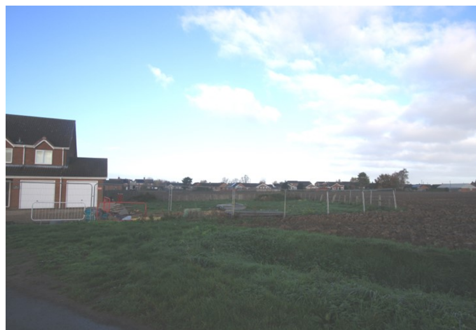
View of Site From Fengate Drove
