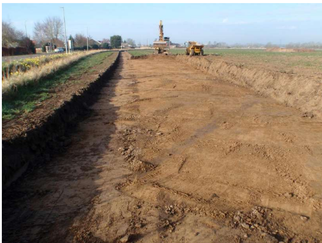
Plate 2. Stripping in progress, looking west
