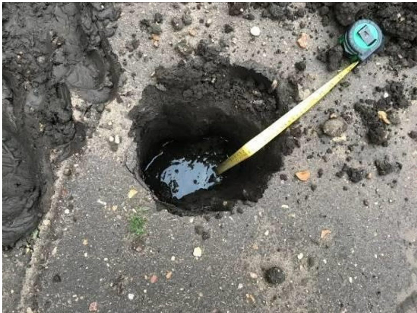
Fig 8 – test pit showing 0.6 m of Topsoil
