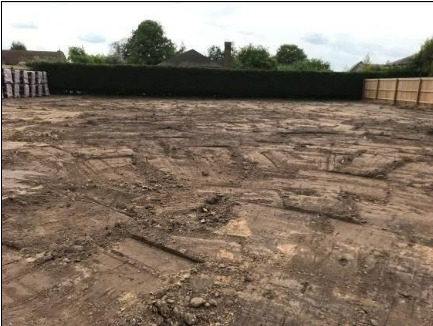
Fig 3– view to west across stripped ground
