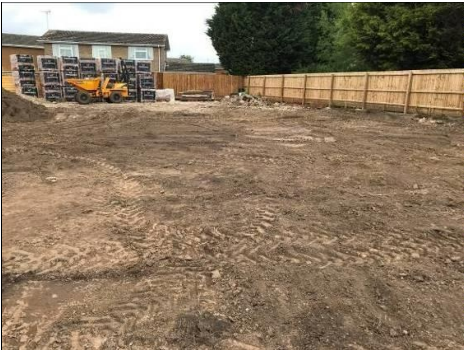
Fig 2 – view to east across stripped ground
