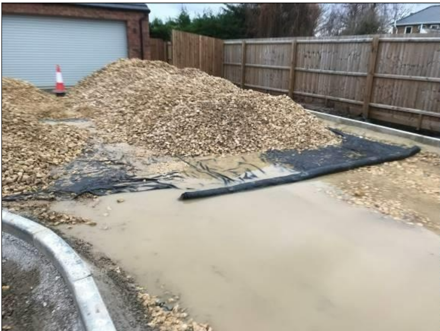
Fig 5 – stone layer and membrane under pavements
