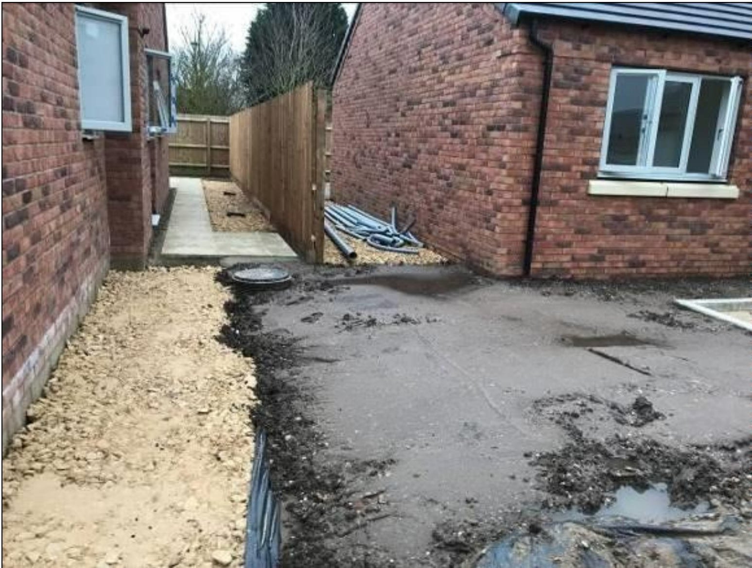
Fig 6 – stone layer, membrane and Topsoil cover emplacement
