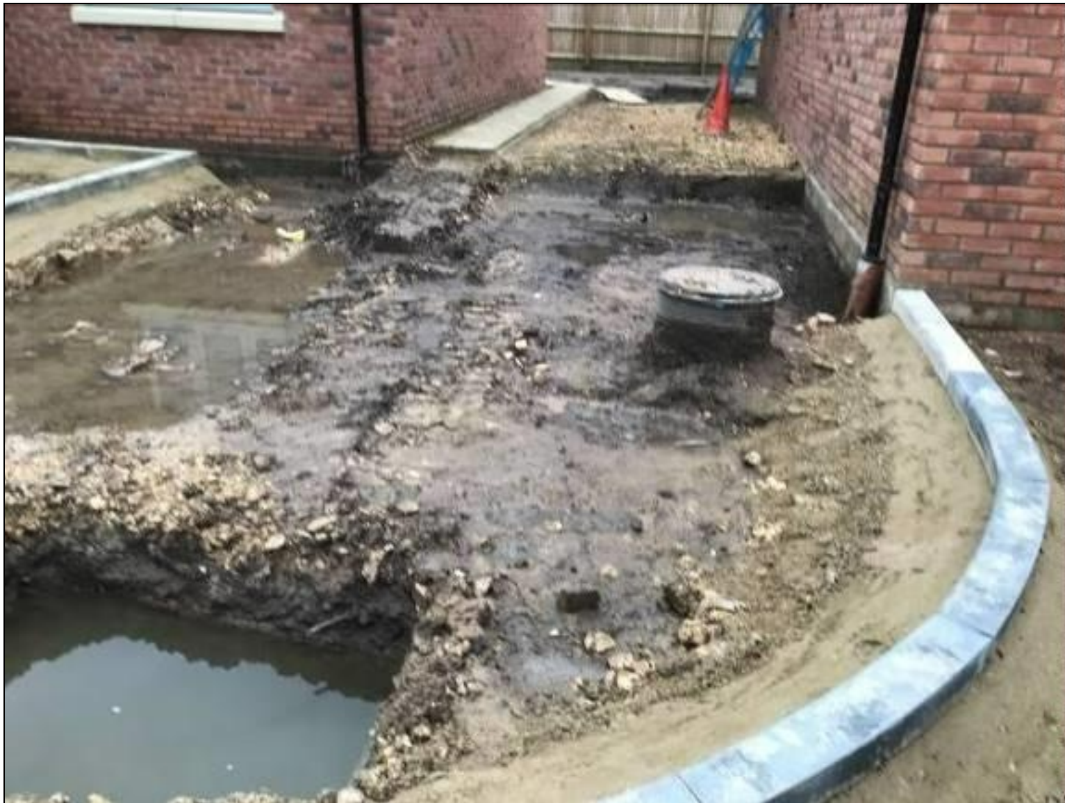
Fig 4 – stone layer awaiting finishing
