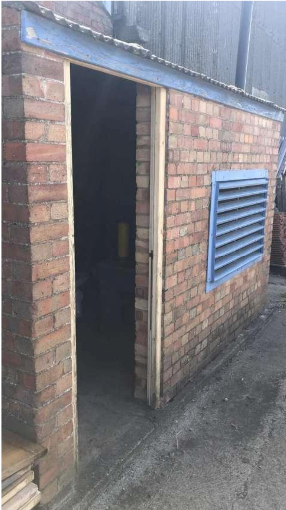
Photo 13 Small extension adjacent to water tank
