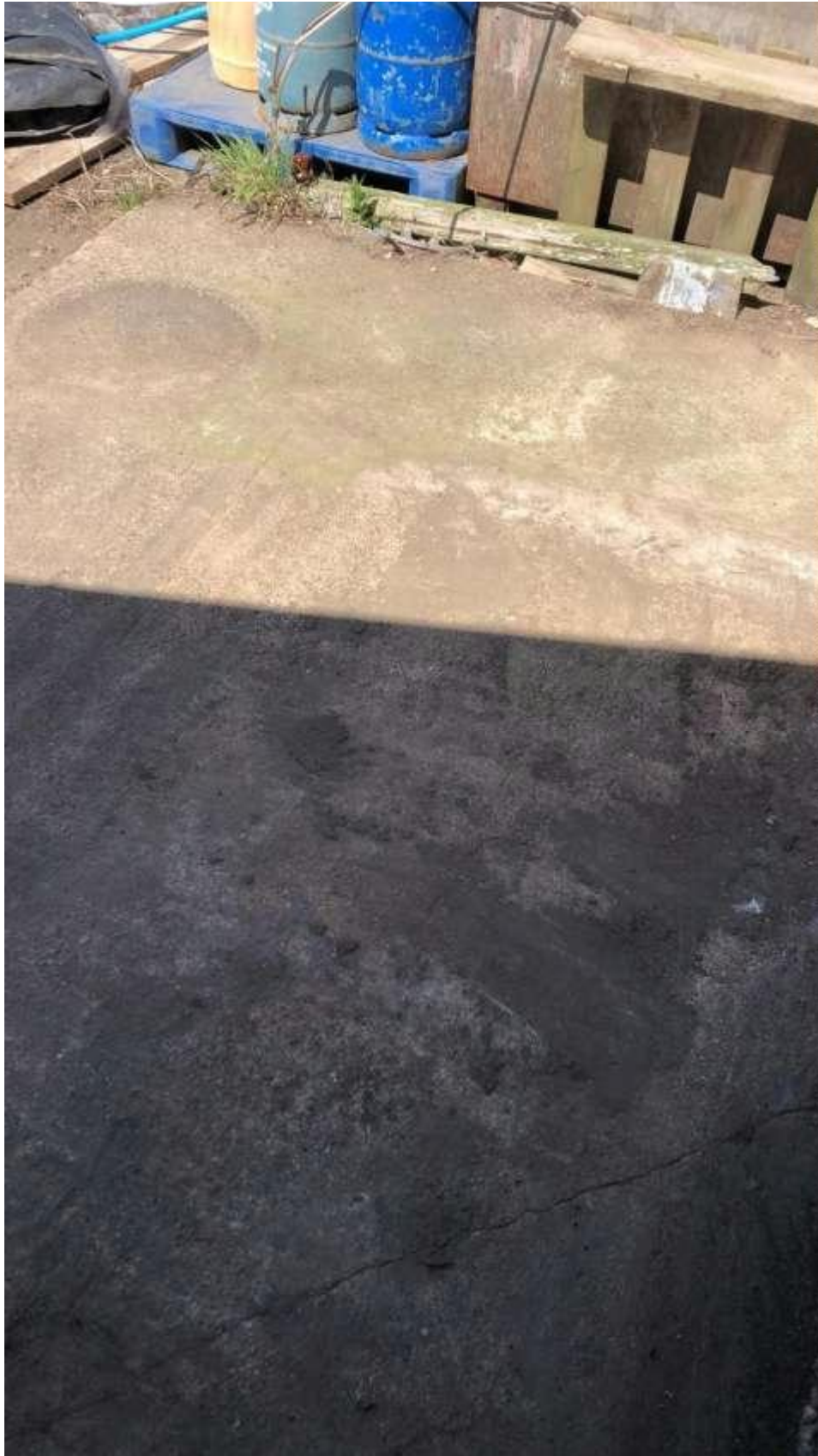
Photo 12 Site of blue tank looking towards the front
