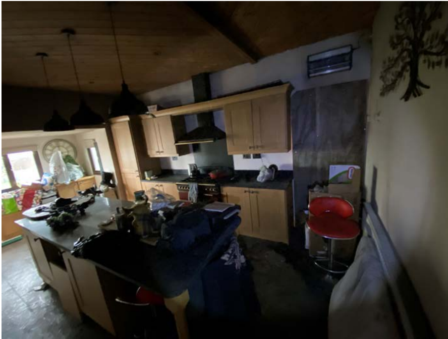
Photo 11 – Kitchen two within Building E
