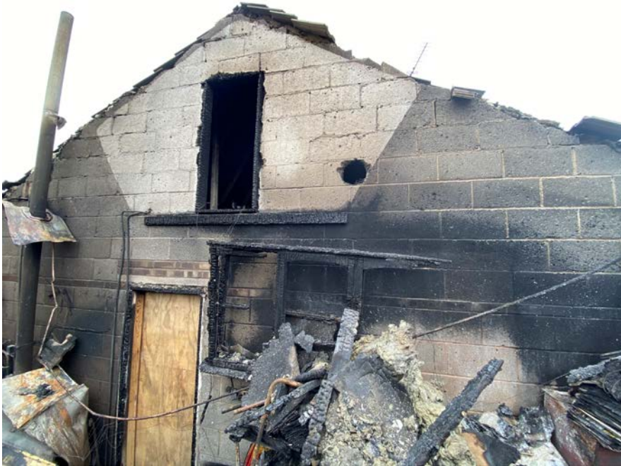
Photo 7- Workshop 1 and partition (door to) kitchen and access to loft void.
