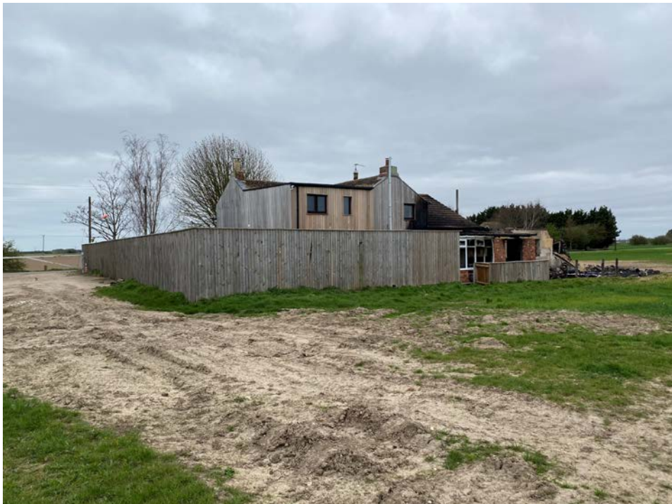
Photo 5 – Left and rear elevation
