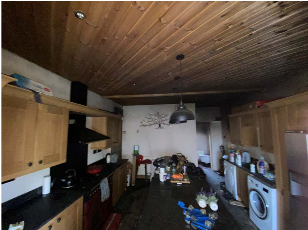
Photo 12 – Kitchen two within Building E
