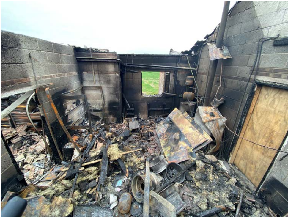
Photo 6 – Workshop 1 and partition (door to) kitchen.
