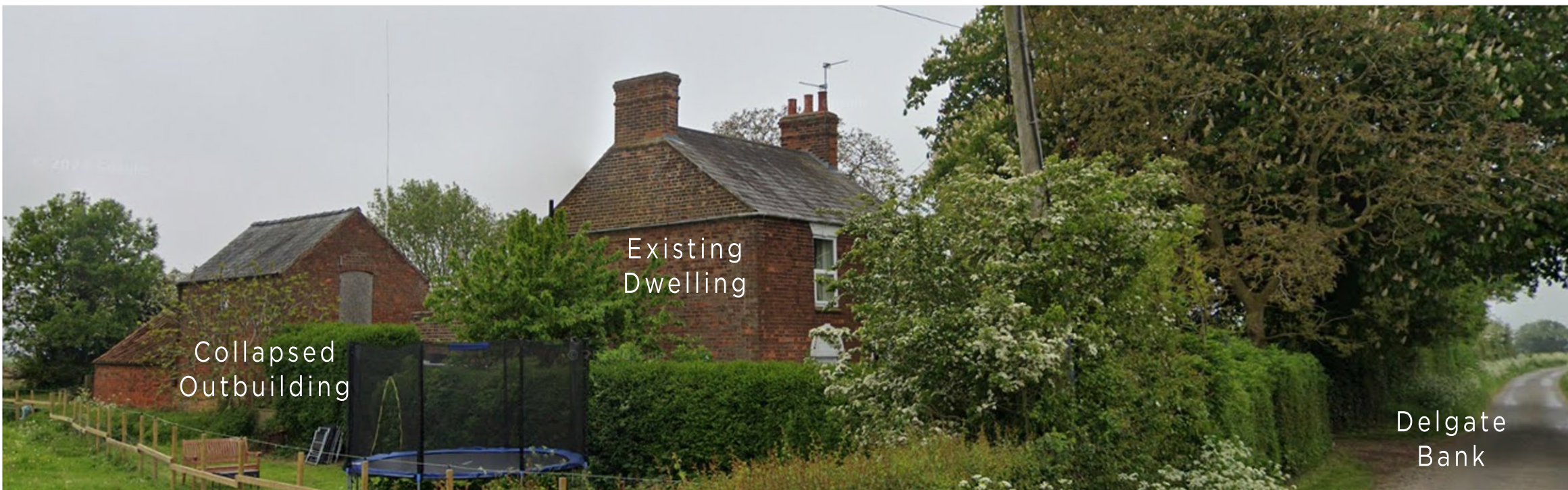
View of Existing/Collapsed Outbuilding (Sourced from Google Street View imagery)
