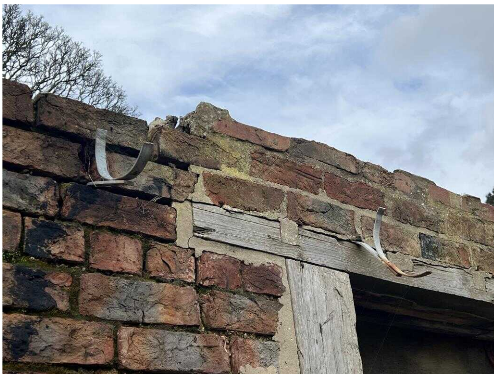
Fig. 35 – Detail of timber around openings on south elevation.
