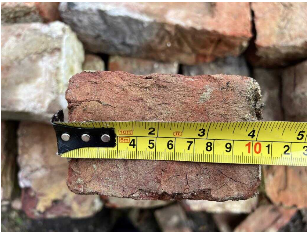
Fig. 23 – Brick, typical width 105mm.
