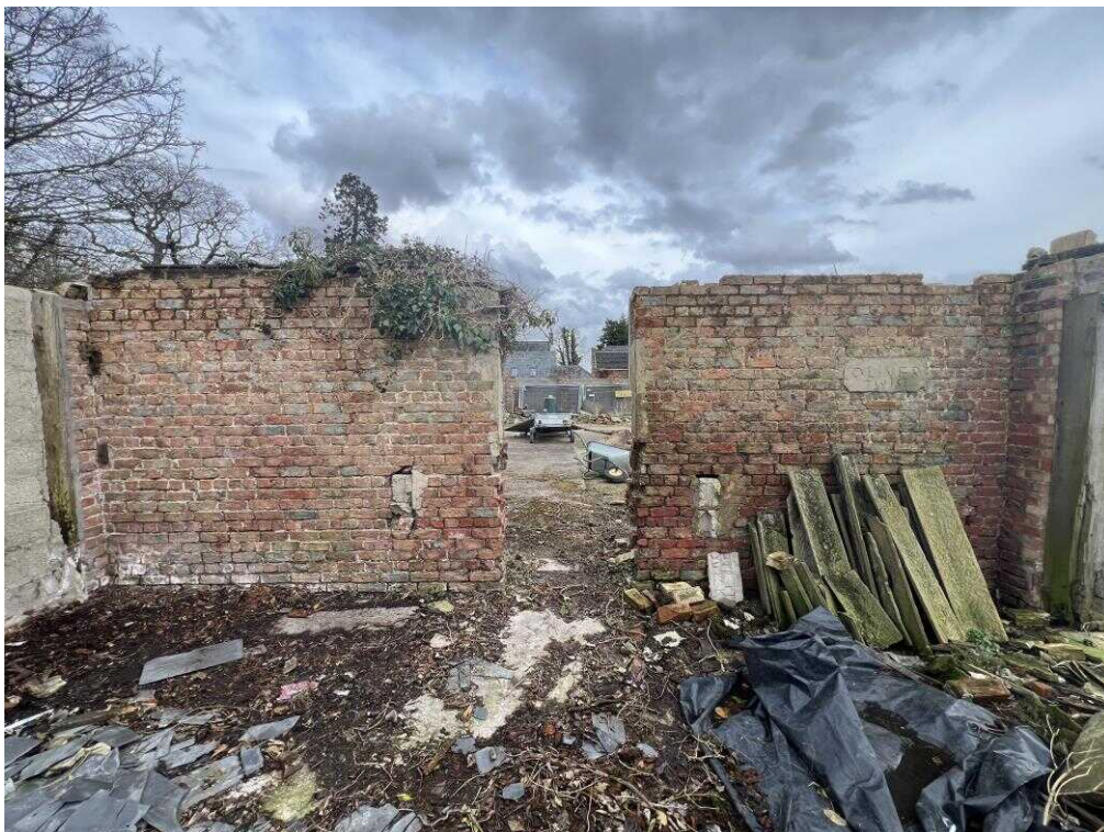
Fig. 17 – Interior view of room looking to east.
