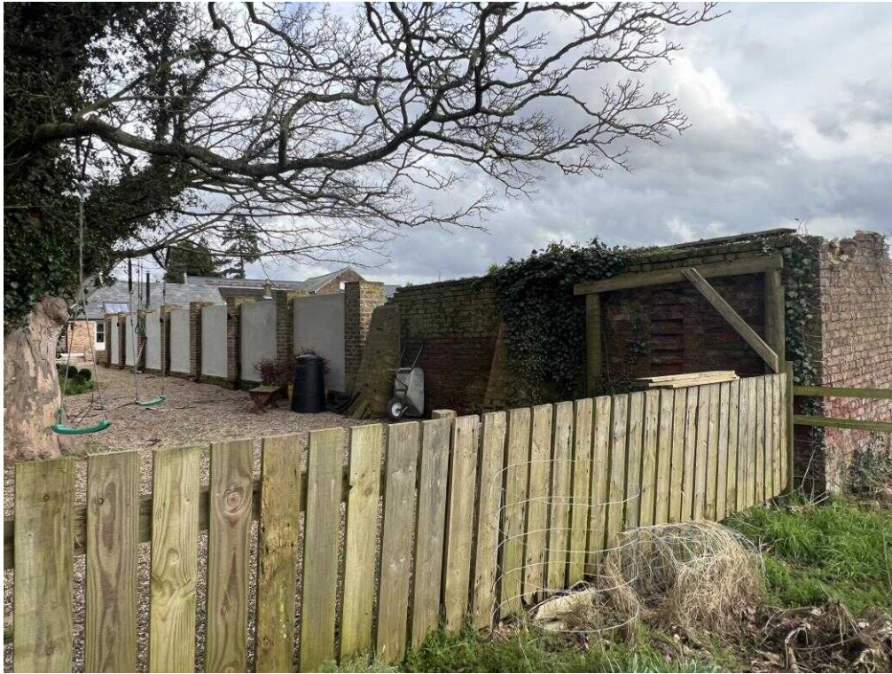
Fig. 12 – Distant view from north. Note – the north elevation is on the site boundary, more distant views are not available from public land.
