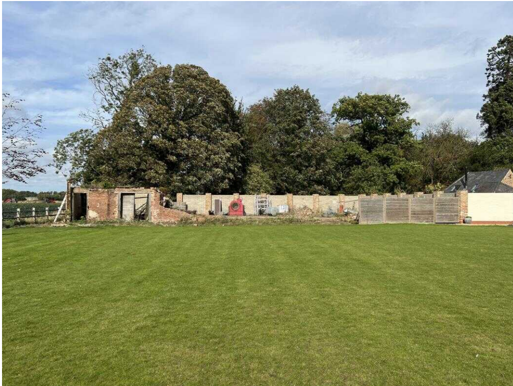
Fig. 06 – Distant view from south.
