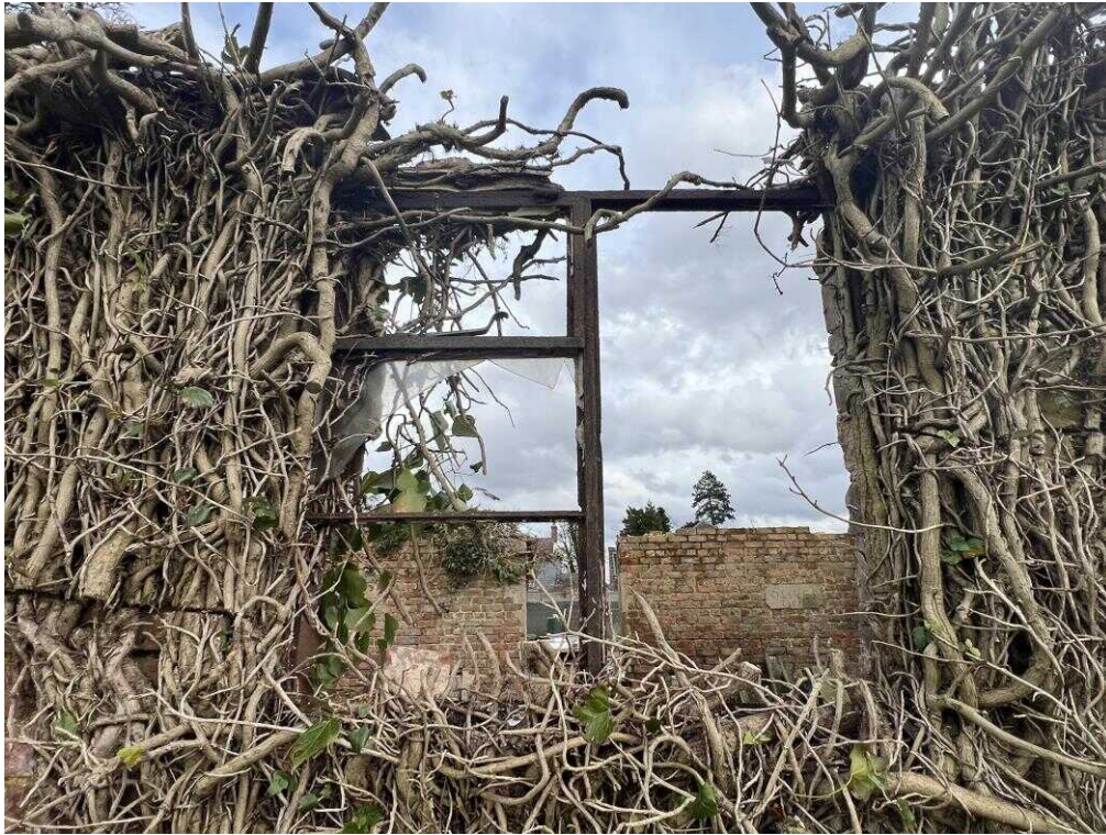
Fig. 43– Steel framed window in west elevation.
