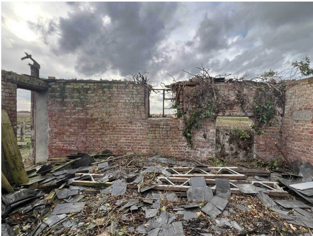
Fig. 15 – Interior view of room looking to west.
