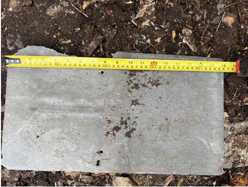
Fig. 30 – Roof slate detail 460mm x 260mm x 6mm (loose on floor).
