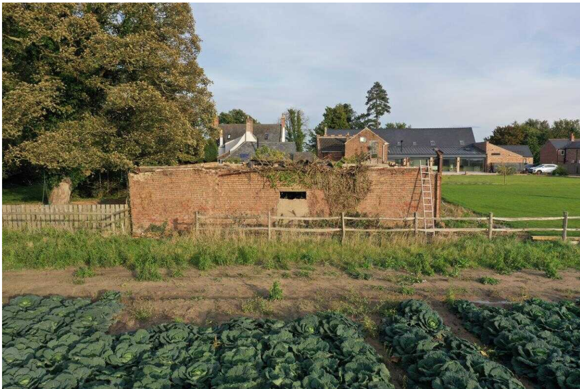
Fig. 09 – Close view from west.
