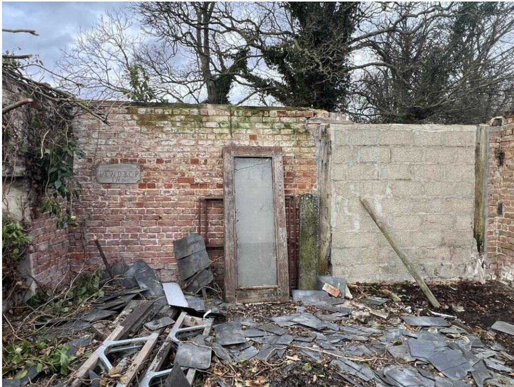
Fig. 16 – Interior view of room looking to north.
