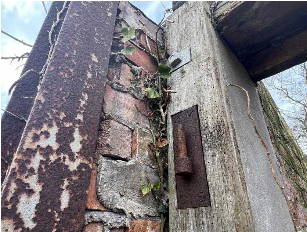
Fig. 40 – Hinge fitting adjacent single door opening on south elevation.
