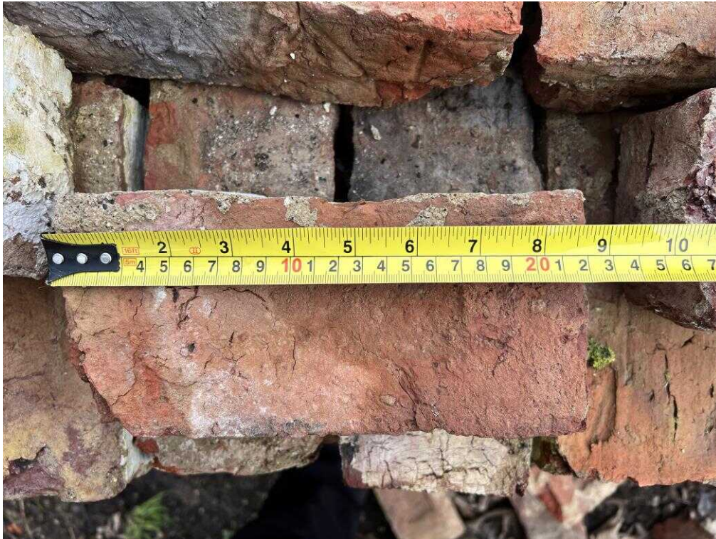
Fig. 22 – Brick, typical length 220mm.
