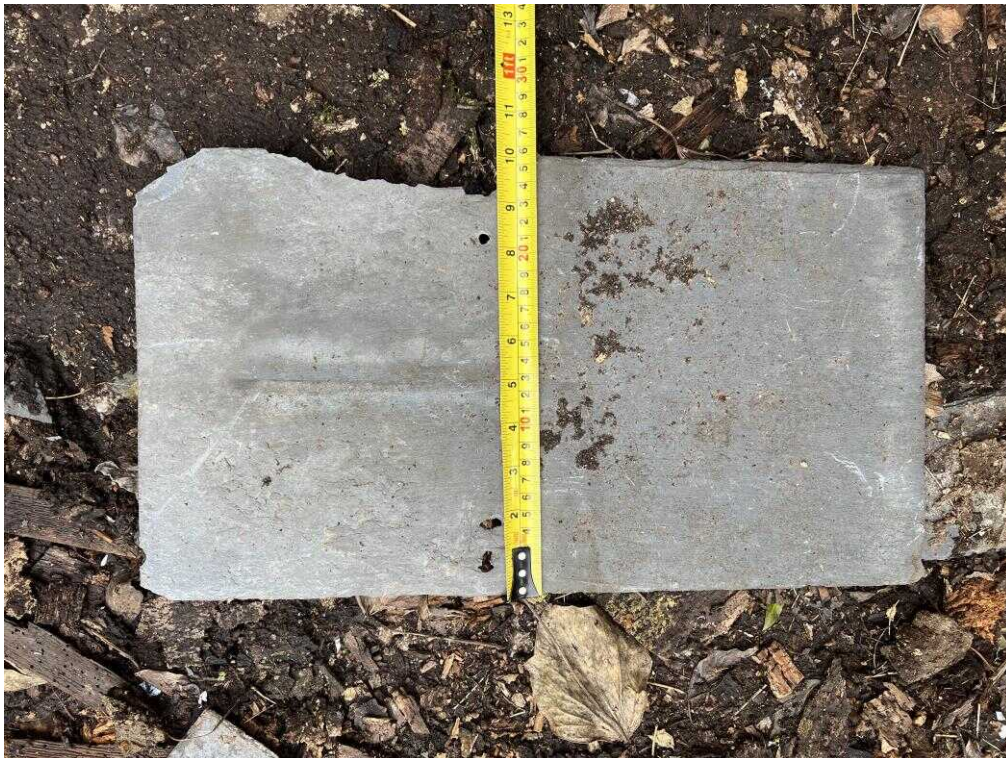
Fig. 31 – Roof slate detail 460mm x 260mm x 6mm (loose on floor).
