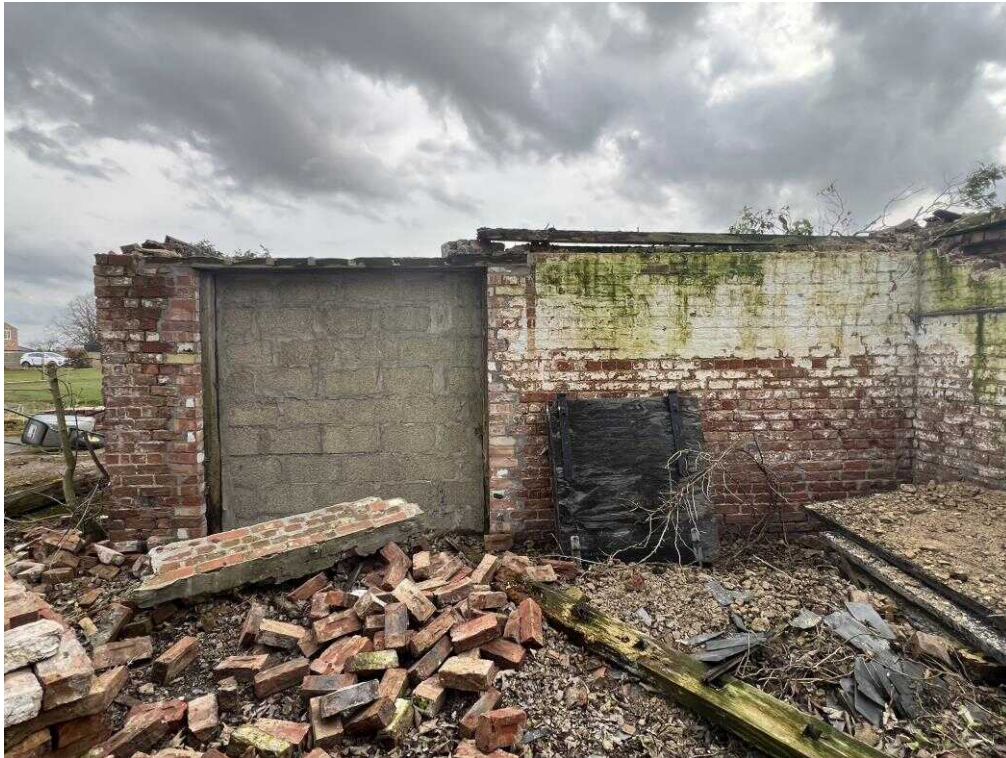
Fig. 18 – View within covered bay looking to south.
