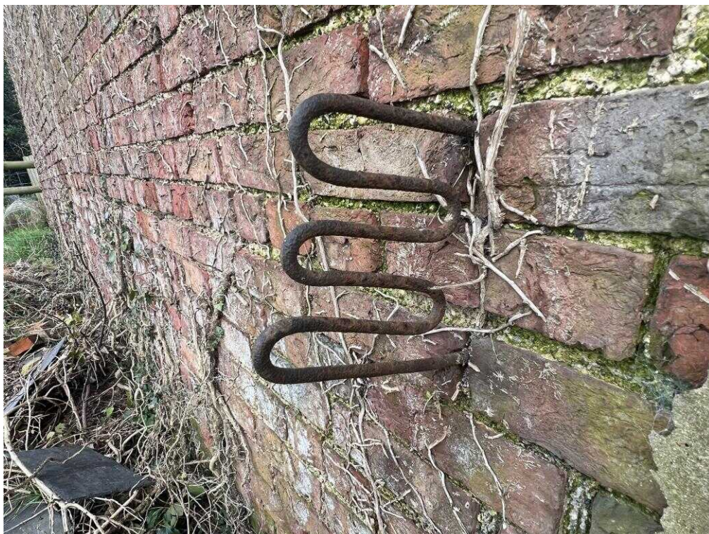
Fig. 38 – Iron fixture on external wall, west elevation.
