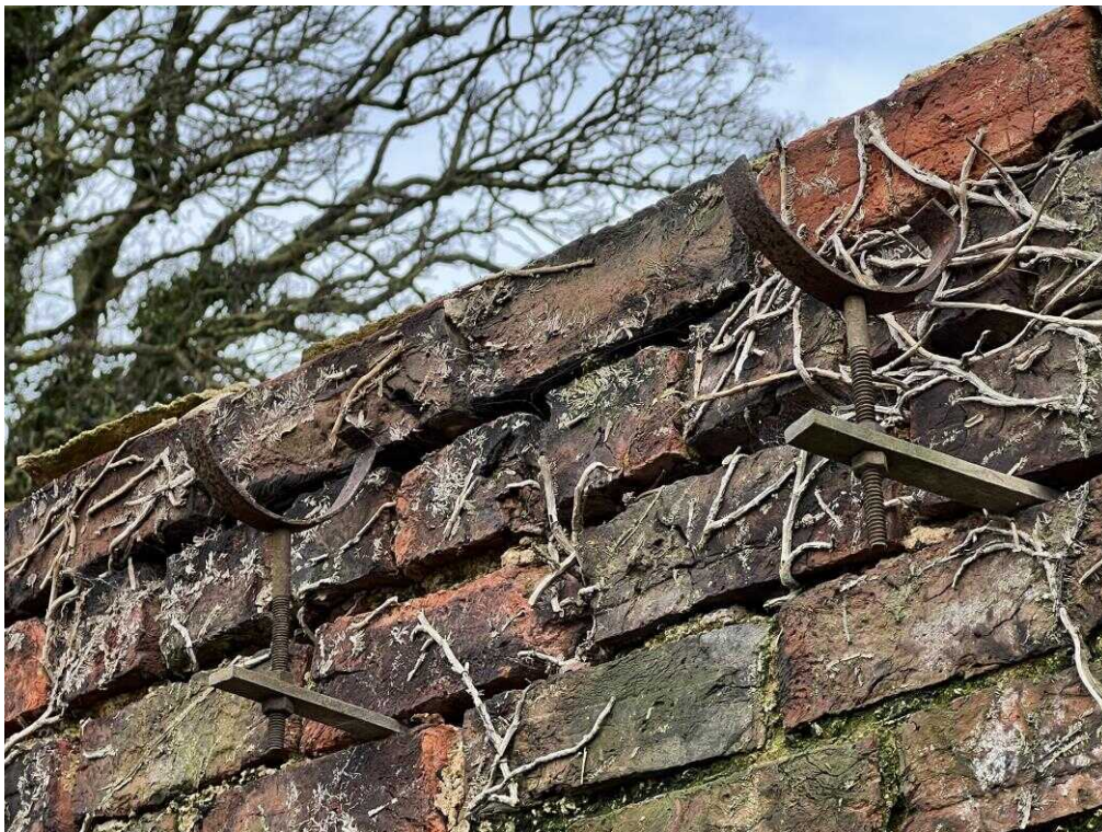
Fig. 28 – Gutter brackets evident on south end of west wall only.
