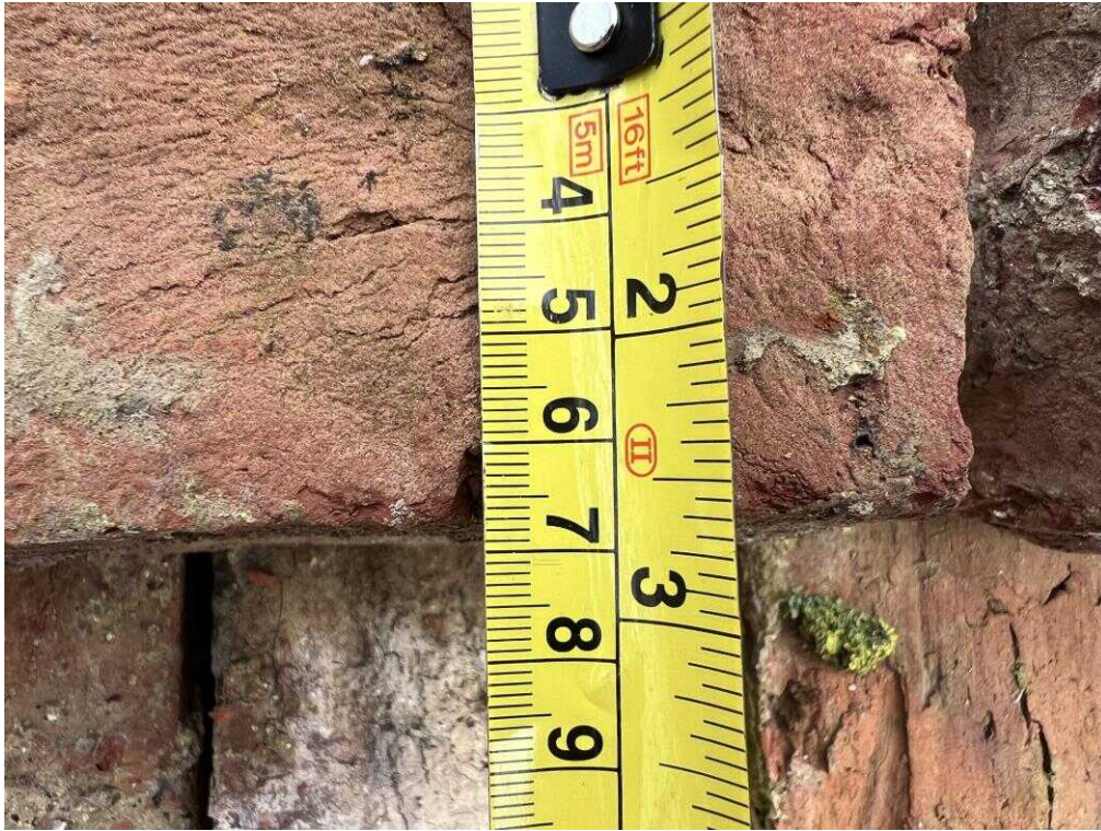
Fig. 24 – Brick, typical depth 70mm.
