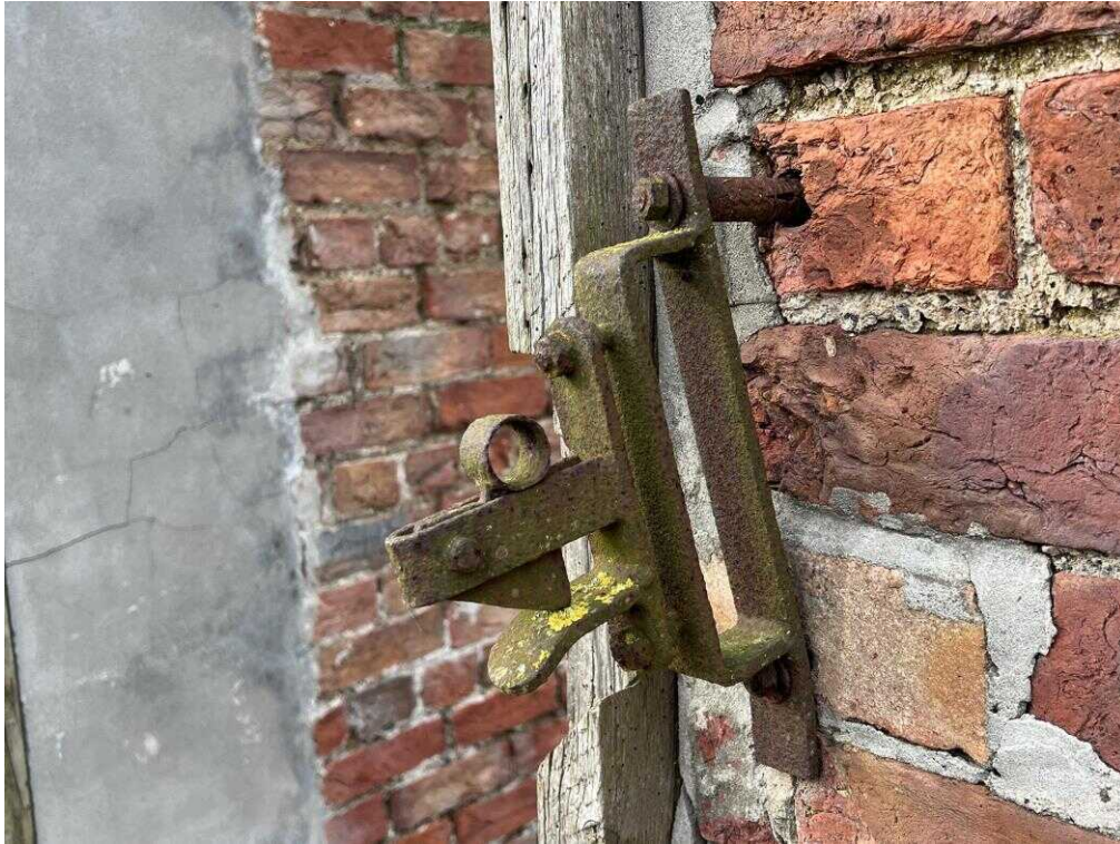
Fig. 39 – Latch adjacent single door opening on south elevation.
