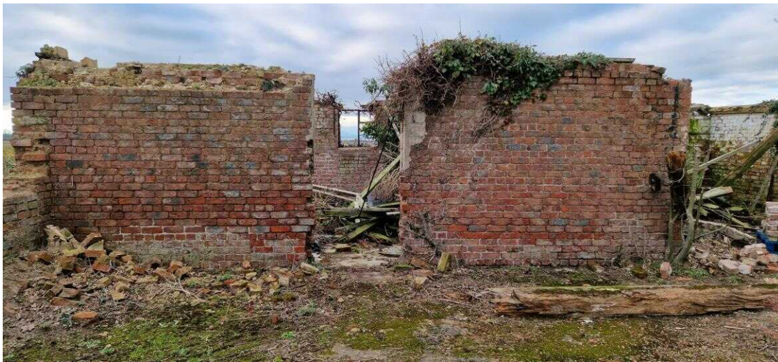
Fig. 11 – Close view from east.
