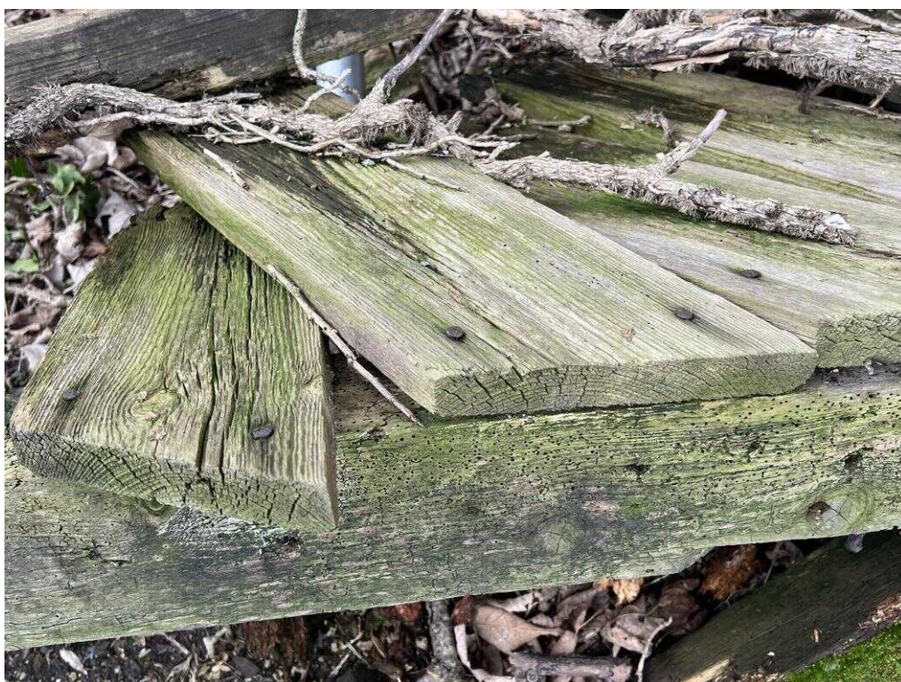
Fig. 33 – Detail of weather-boarding infill from east gable of roofed-in area.
