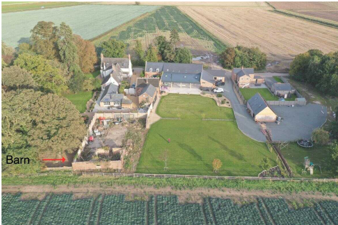
Fig. 04 – High-level view from west.
