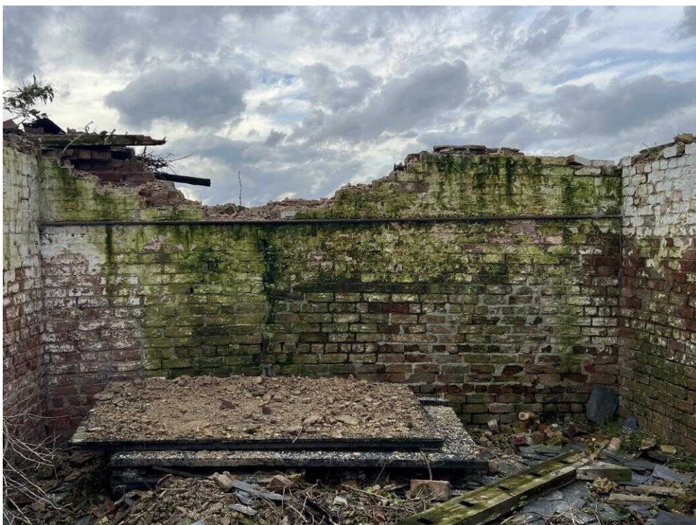
Fig. 19 – View within covered bay looking to west.
