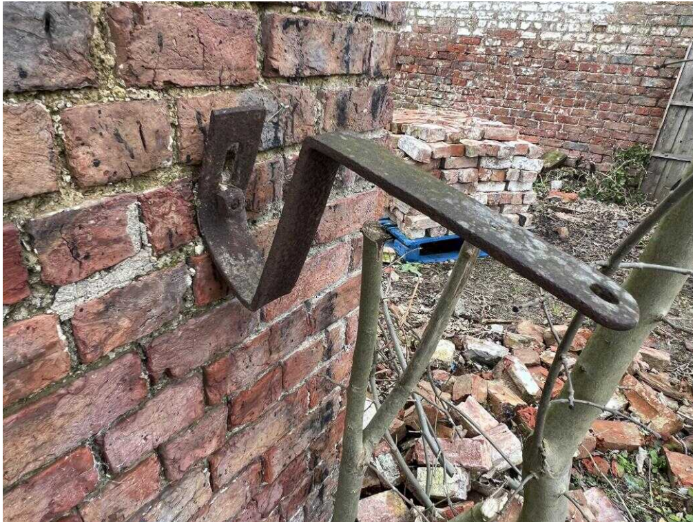
Fig. 41 – Bracket at mid-height, north end of east wall, external.
