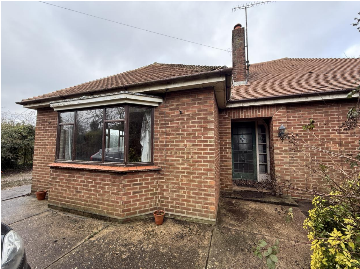
View of existing bungalow
