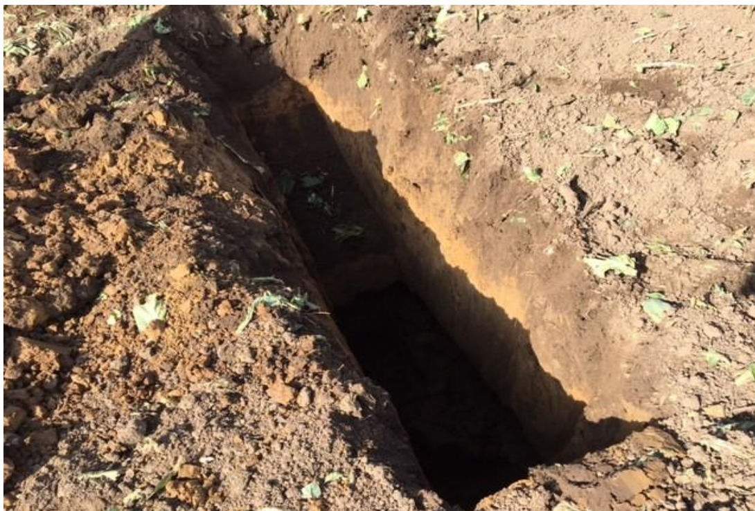
Photograph 5: View of a trial pit excavated on Site.
