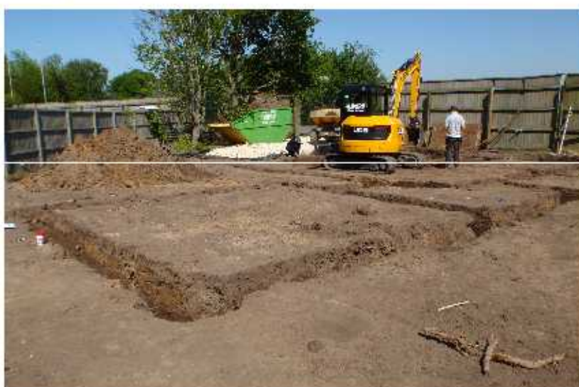
Plate 3. General view of footings, looking northeast
