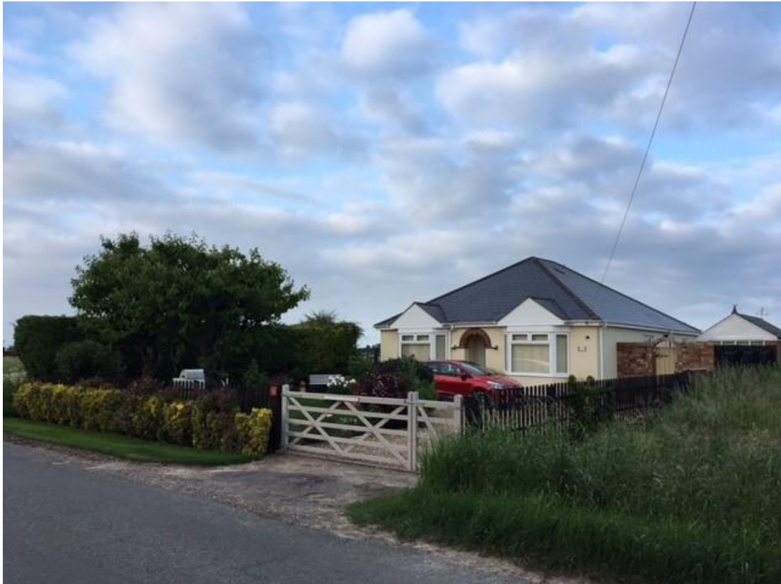
Bungalow on opposite side of Broadgate (247 Broadgate)
