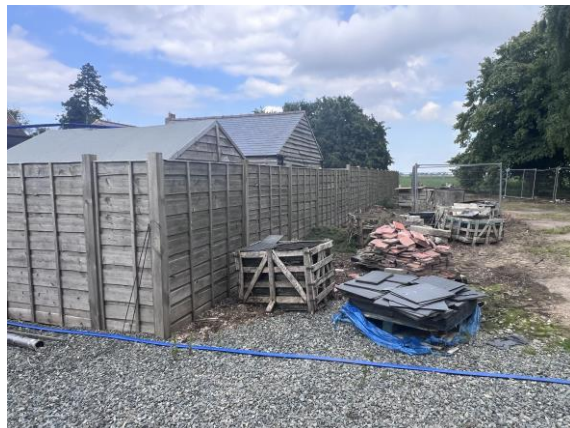
Fig. 05 – North boundary, neighbouring fence.
