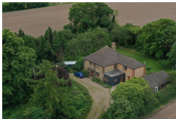
Fig. 11 – Substantial dwelling south of the site.
