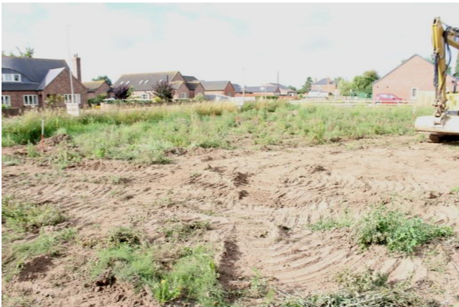
Plate 2: Pre-site works, from the north-east
