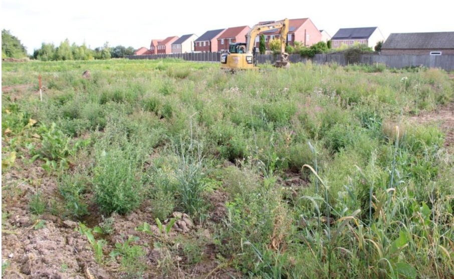
Plate 1: Pre-site works, from the south-west
