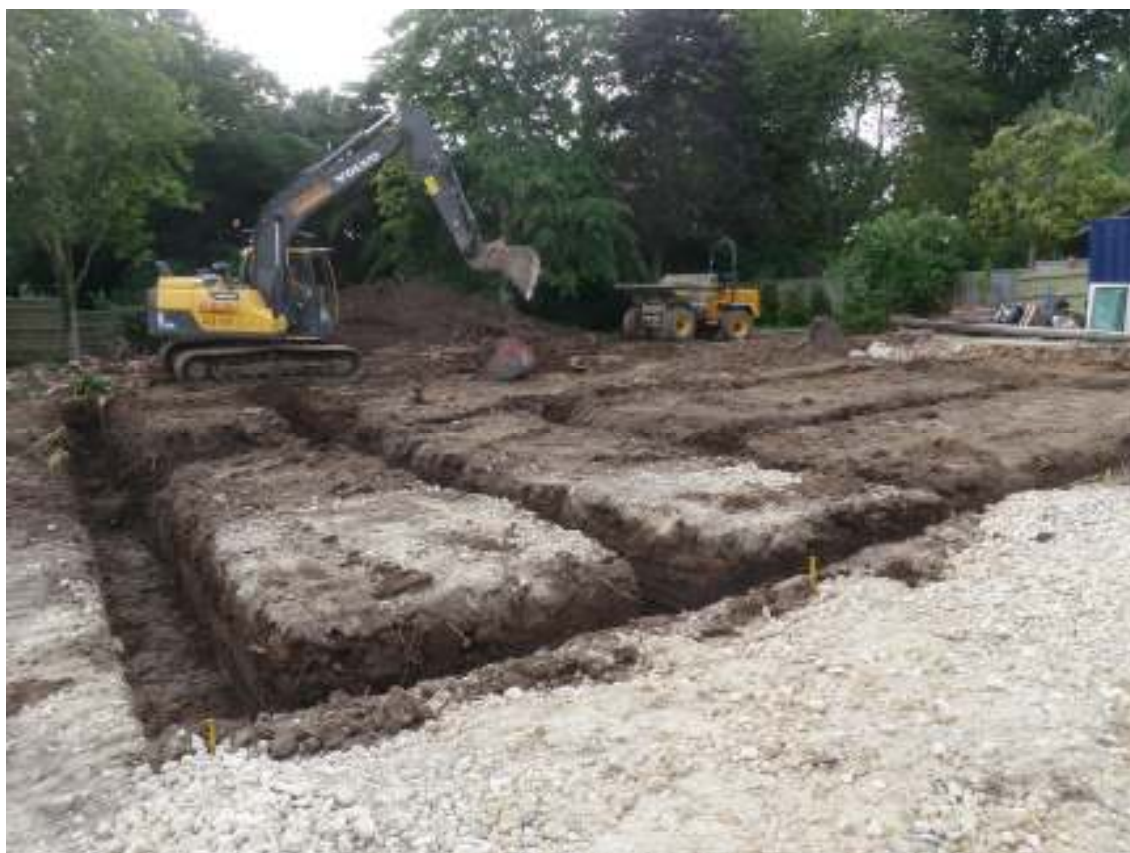
Plate 5. Overall view of house footings looking west
