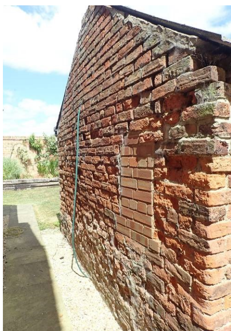
Plate 4. The west elevation of building 1 with a blocked window aperture on its south end
