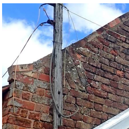
Plate 15 (above). Detail of the tumbled brickwork on the south elevation of Building 2
