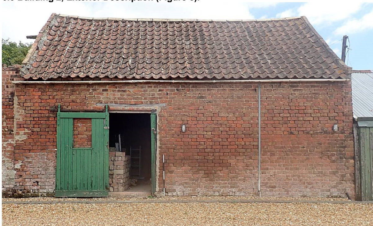
Plate 14. The west elevation of the southern part of Building 2
