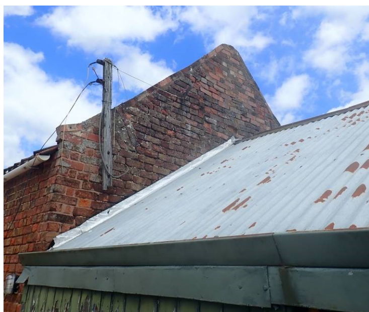
Plate 15 (above). Detail of the tumbled brickwork on the south elevation of Building 2
