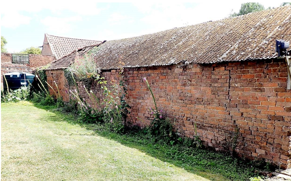
Plate 5. The north elevation of Building 1
