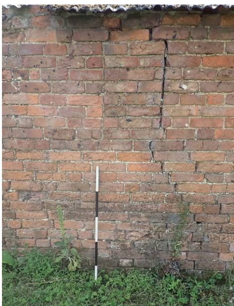
Plate 6. Blocked aperture on the west end of the north elevation of Building 1
