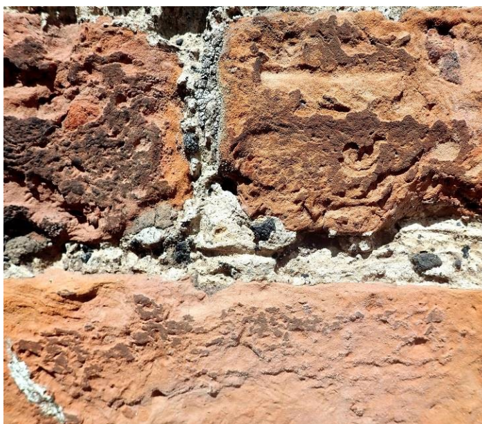
Plate 7. Detail of the lime mortar on Building 1
