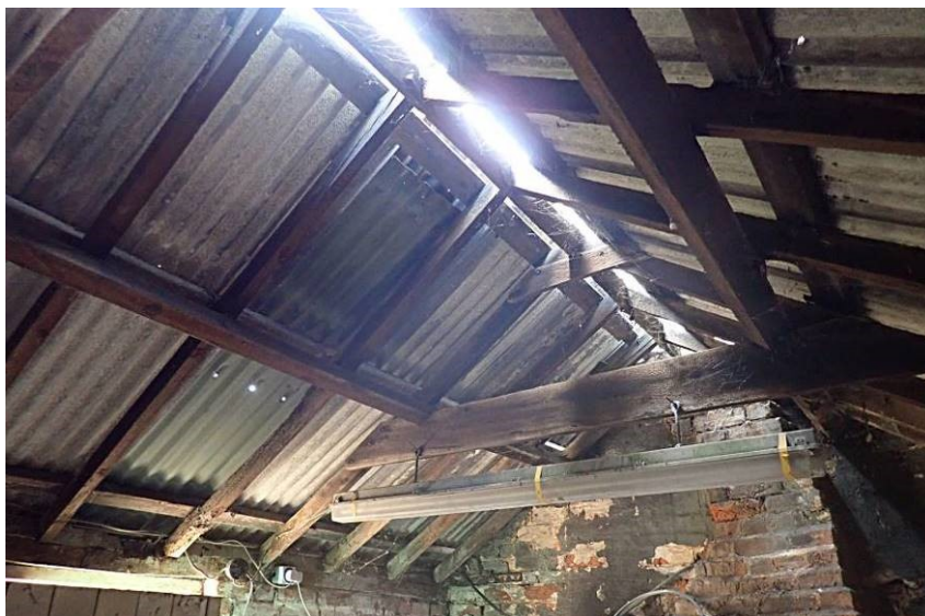
Plate 11. Replacement roof timbers in Building 1
