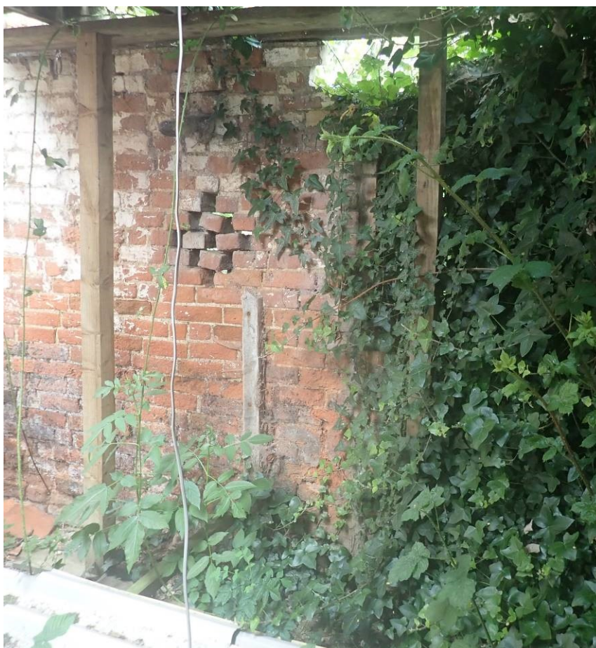
Plate 27. The breather slit and position of a blocked doorway in Room 2 of Building 2
