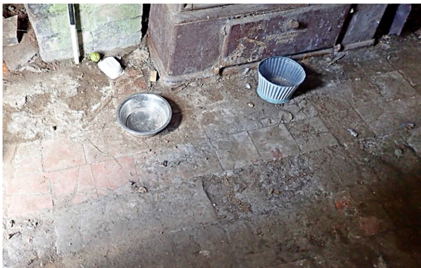
Plate 8. The quarry tile floor in Room 1 of Building 1
