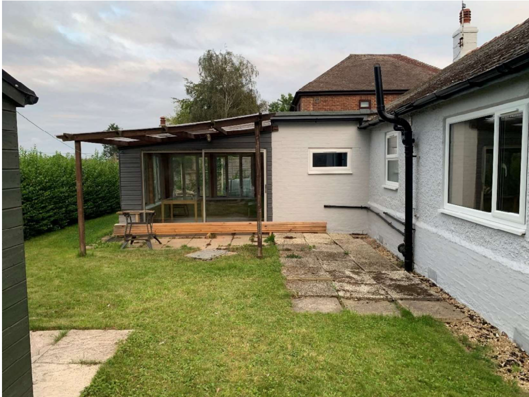
External view of new window
