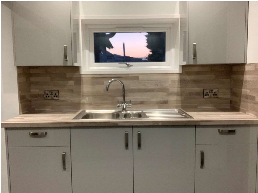
Internal view of new window
