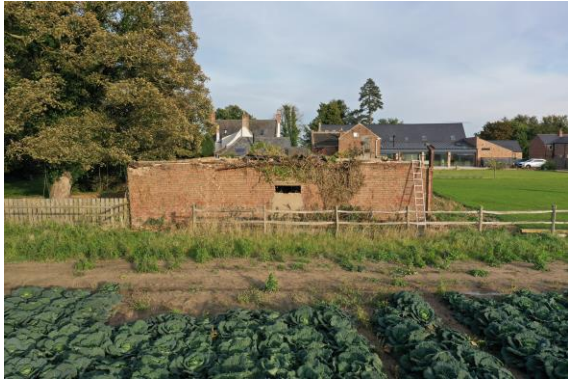
Fig. 09 – View of barn from west.
