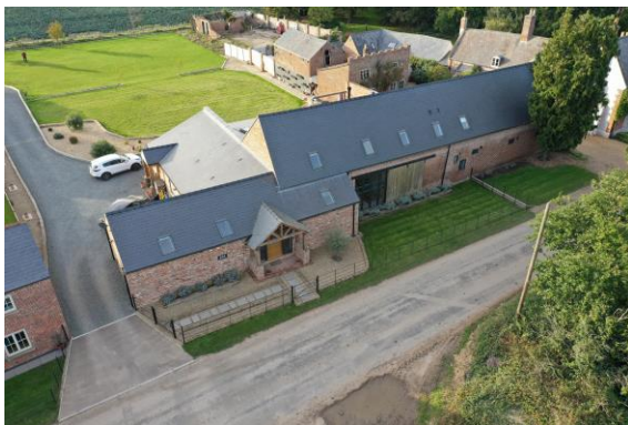
Fig. 07 – View of larger barn from south-east.
