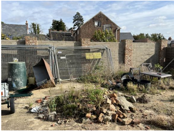
Fig. 02 – East boundary, high boundary wall.
