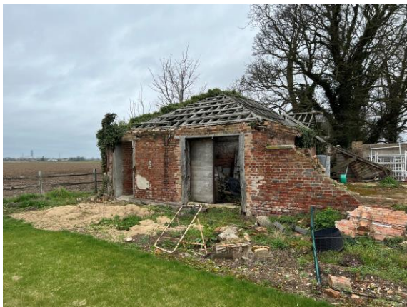
Fig. 04 – West boundary, timber fence (to left of barn).
