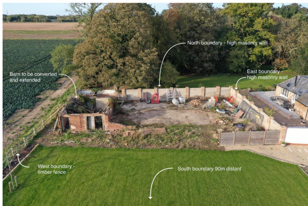
Fig. 01 – Aerial view showing the barn in relation to the various site boundaries.
