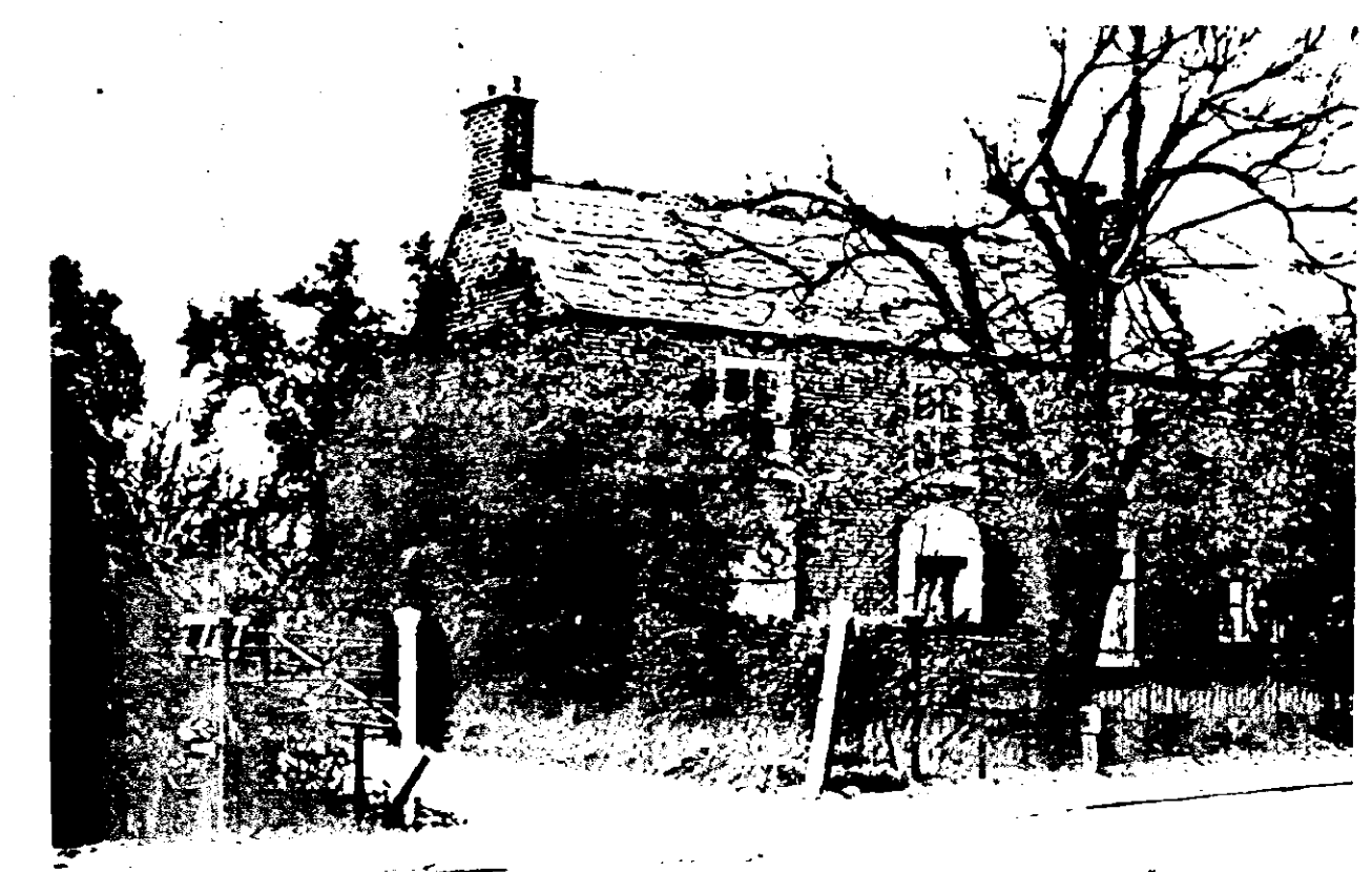
EXISTING VEHICULAR ACCESS TO OAKLEIGH HOUSE IS EXTREMELY DANGEROUS. proposal will remove this unsatisfactory hazard.
