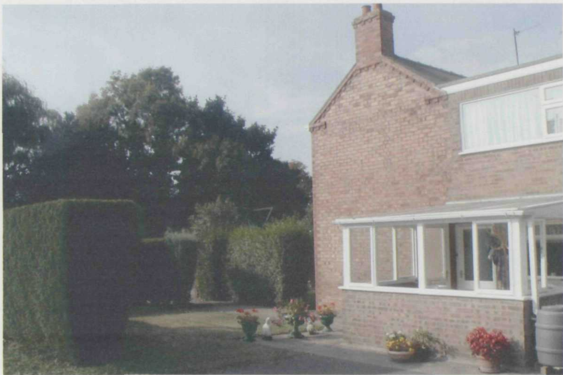
view south west inside property with east wall on right
