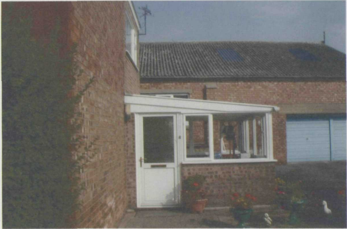
view from inside property looking north with east wall on left
