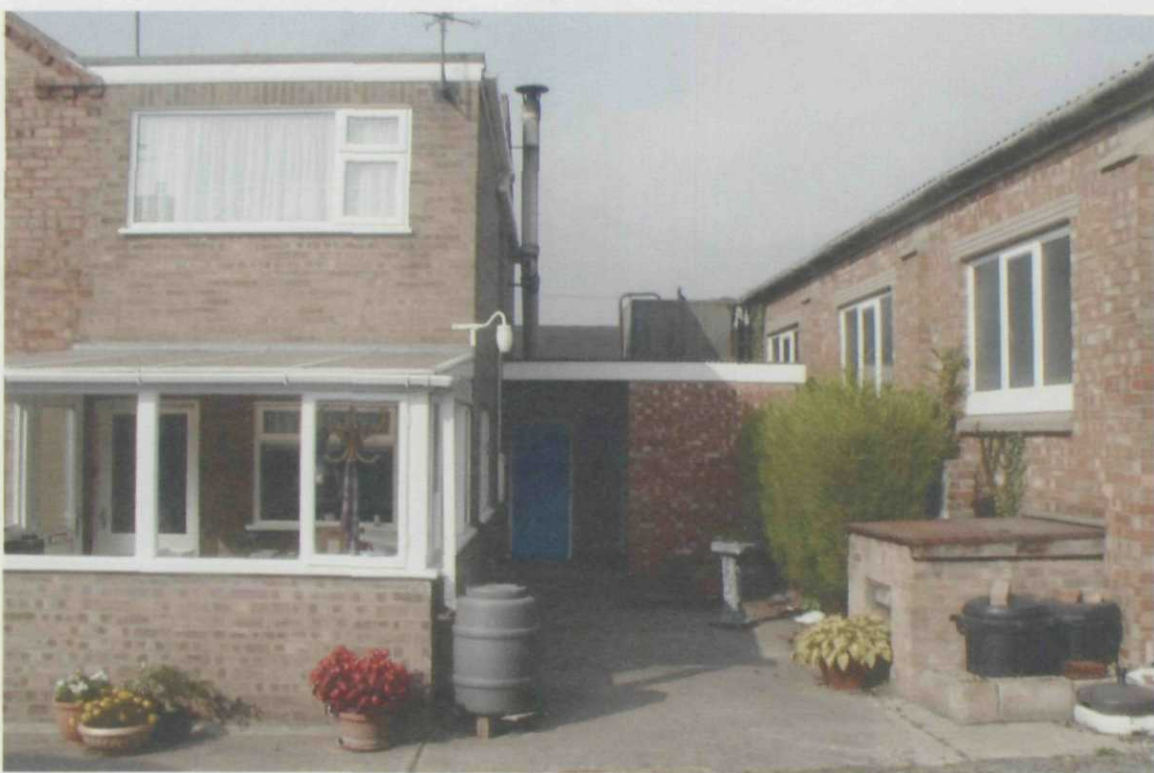
looking west view of east side + rear (north side) of property with store/depot on right of picture
