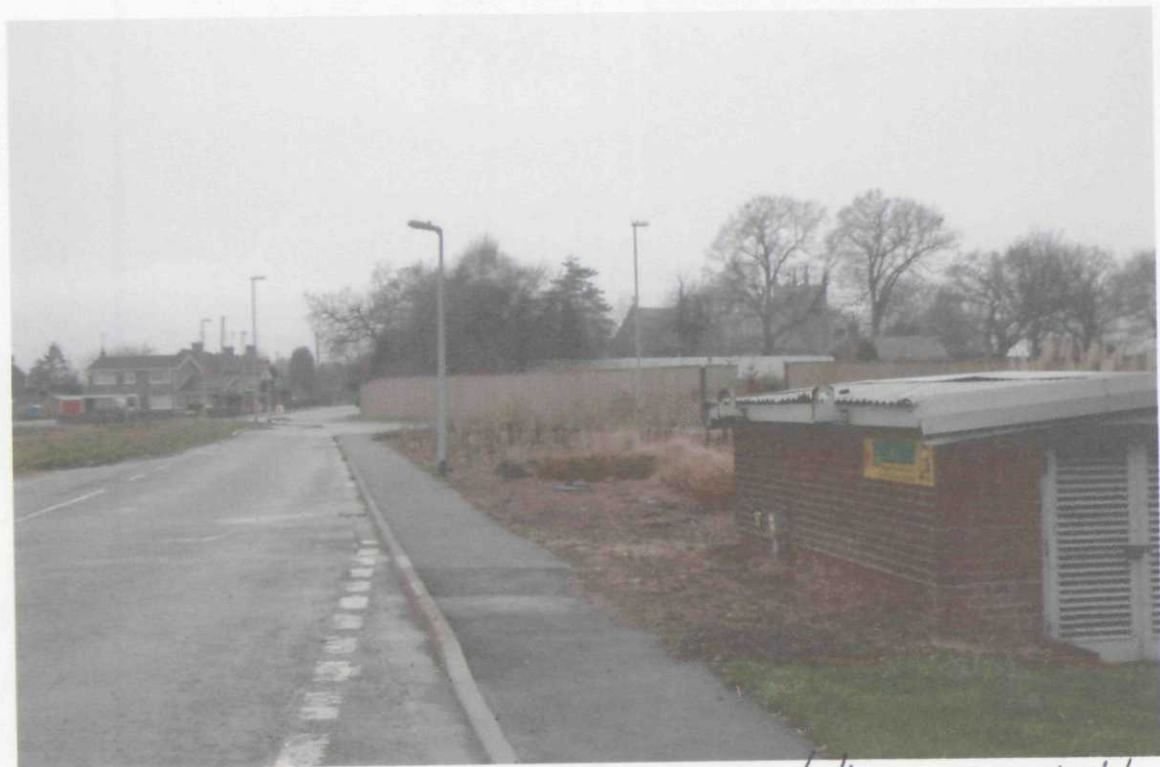
view south from A151 substation on right
