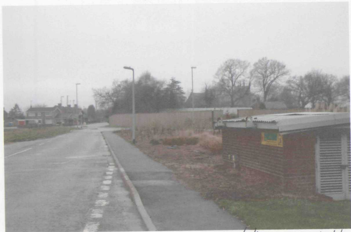
view south from A151 substation on right
