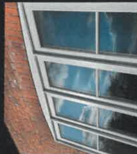
Multilayer stiffener used to replicate the original aesthetics of the windows
