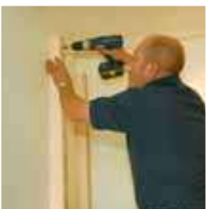
1. SWIP Studs fixed to wall
