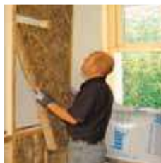
2. SWIP Batt between SWIP Studs
