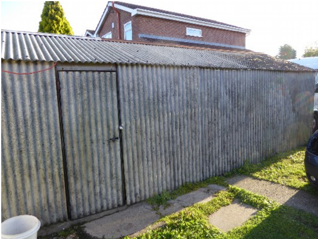
Photo 4 Cement stabilized fibre panels on garage at Cedarwood
