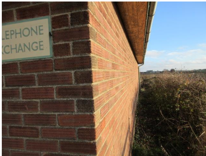
Photograph # 5 (Side – South facing elevation)
