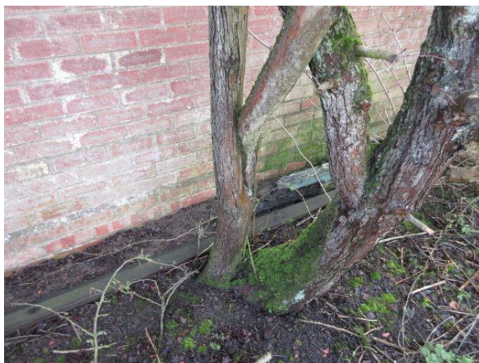
Photograph # 15 (Side – North facing elevation – Adjacent Tree – low level )
