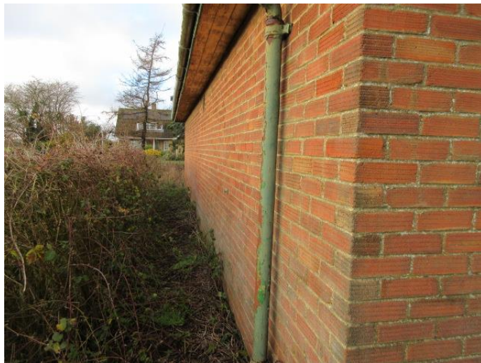
Photograph # 6 (Side – South facing elevation)
