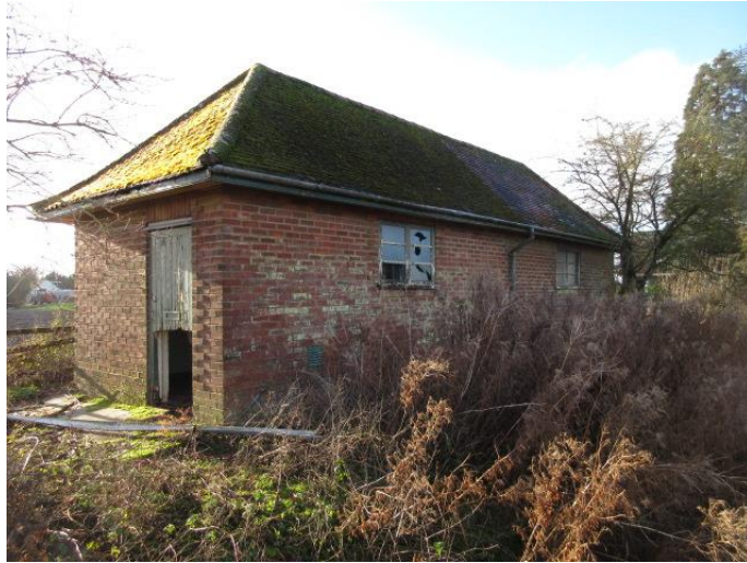
Photograph # 4 (Side – North facing elevation / Rear – East facing elevation)
