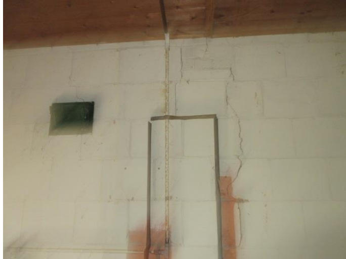
Photograph # 10 (Typical Internal – Side – South facing elevation)
