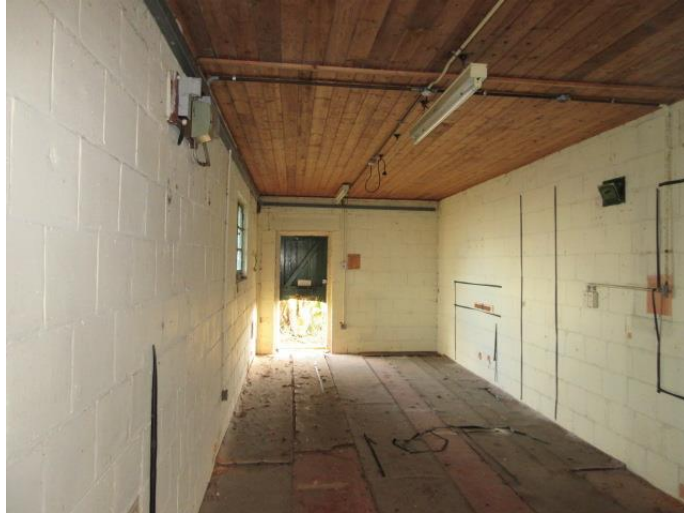
Photograph # 19 (Typical Internal)
