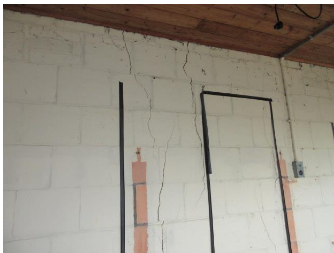
Photograph # 12 (Typical Internal – Side – South facing elevation)
