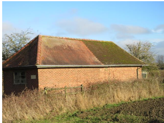
Photograph # 2 (Side – South facing elevation)
