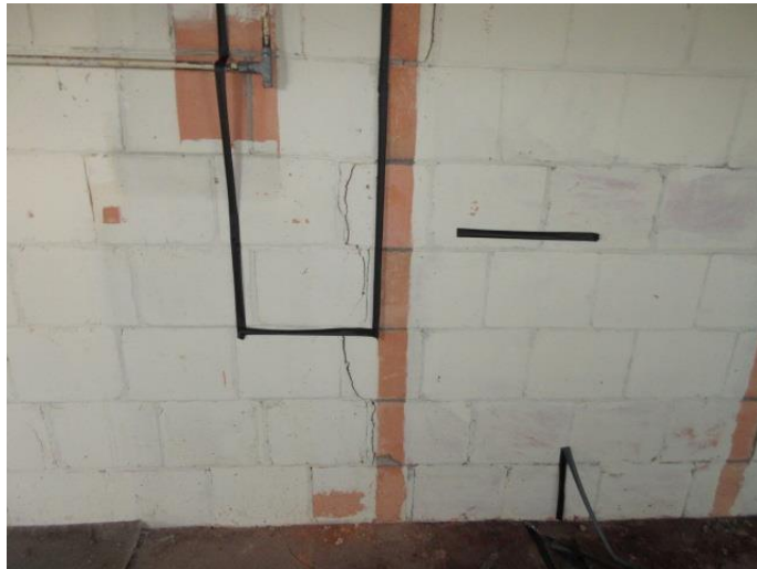
Photograph # 11 (Typical Internal – Side – South facing elevation)
