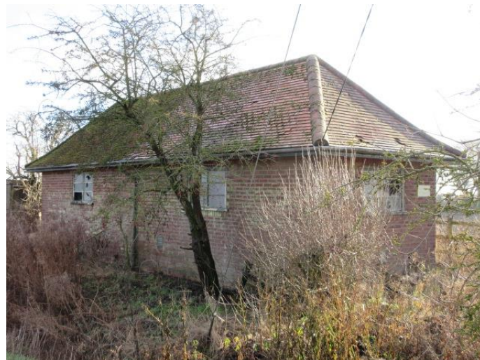
Photograph # 3 (Side – North facing elevation) (
