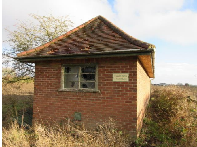
Photograph # 1 (Front – West facing elevation)
