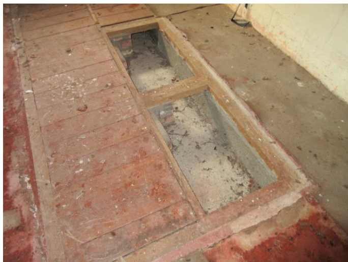
Photograph # 21 (Typical Internal – slab with former recess / pits still present)
