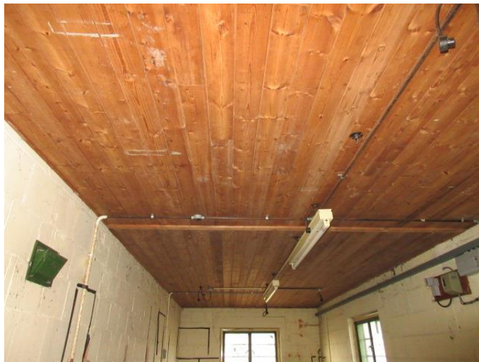
Photograph # 20 (Typical Internal - Underside of Ceiling)
